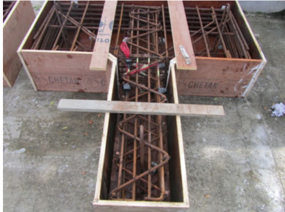
Fig. 4 Beam mould with reinforcements
