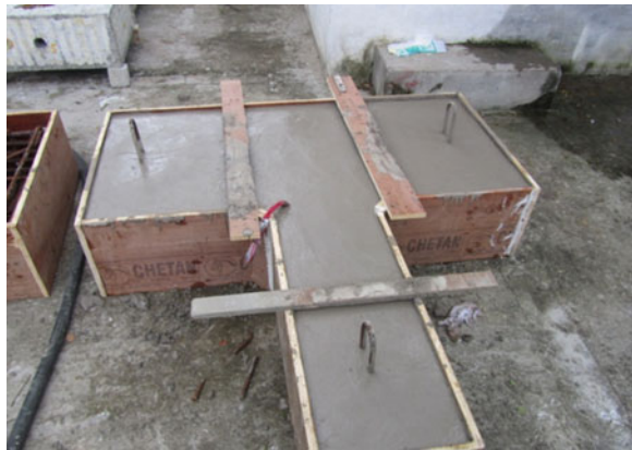
Fig. 5 Beam specimen after casting
