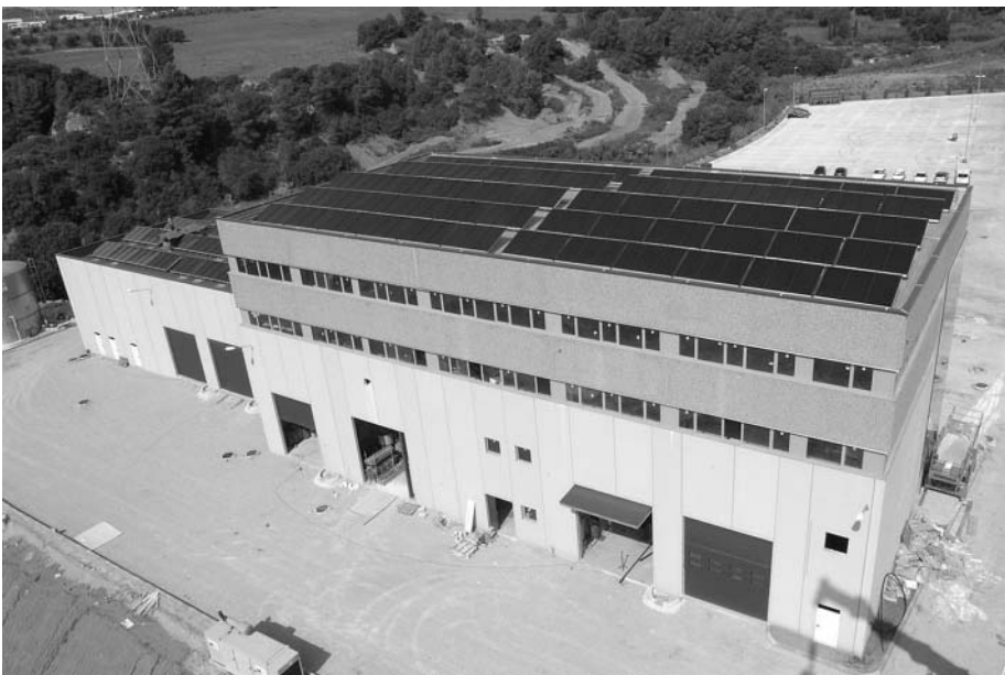
FIGURE 18.40 Parking service Castellbisbal SA, container washing, Spain. Installed capacity: 357 kW th . (From Aiguasol Engineering, Spain. With permission.)
