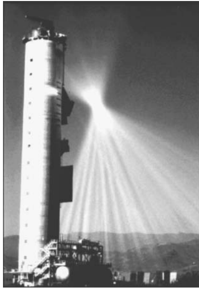
FIGURE 19.48 Lateral view of the 80-m concrete tower of the CESA-1 facility located at the Plataforma Solar de Almería in Spain. The concentrated flux is aiming a standby position previous to start operation.
