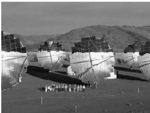
FIGURE 20.40 Several 25-kW solar systems modules. Again, note the people in the foreground for an idea of module scale.
