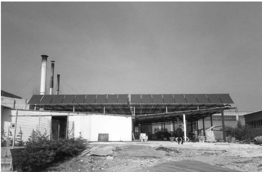
FIGURE 18.38 Alpino SA, dairy industry, Greece. Installed capacity: 518 kW th . (From Alpino SA, Greece. With permission.)
