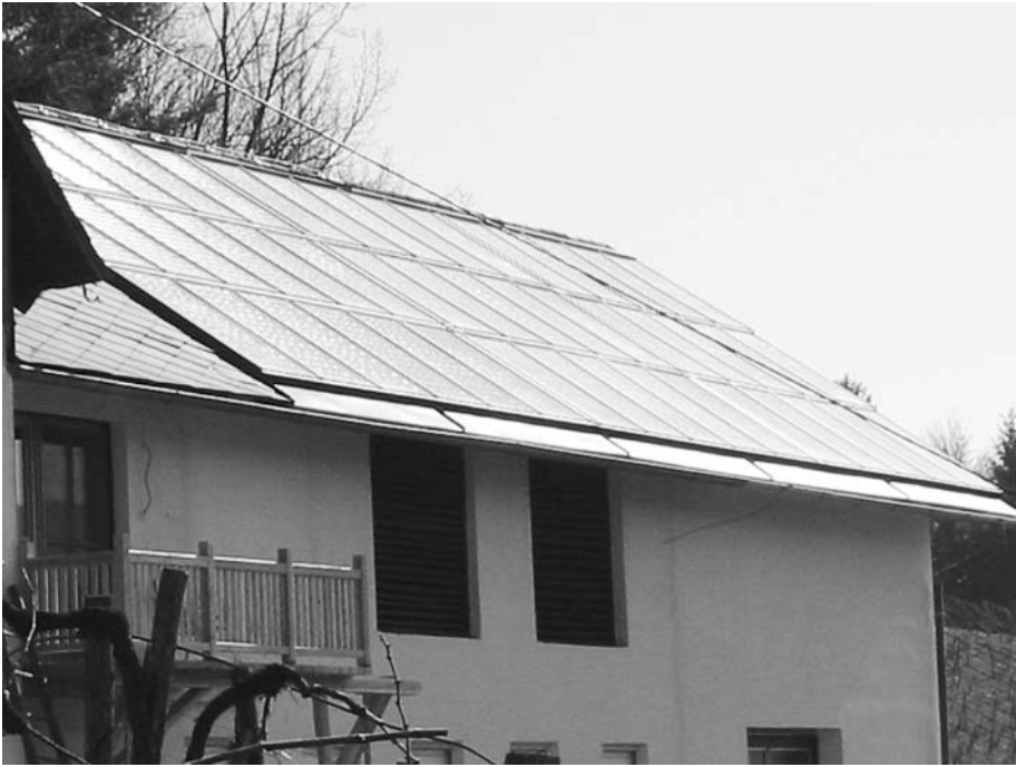
FIGURE 18.39 Wine cooling and bottle washing, Austria. Installed capacity: 70 kW th . (From S.O.L.I.D. GmbH, Austria. With permission.)
