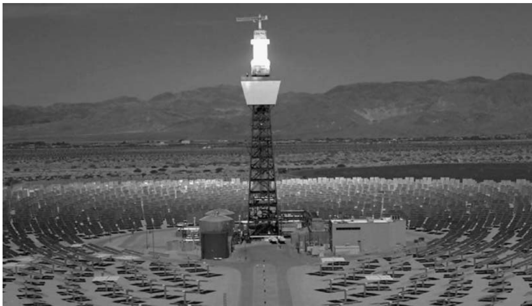
FIGURE 19.64 Aerial view of Solar Two power plant located in Barstow, California. Cylindrical 42-MW receiver appears illuminated. Hot and cold molten storage tanks are located close to the tower.
