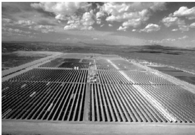
FIGURE 19.37 Aerial view of the SEGS III and IV plants.
