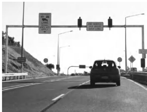
Figure 4.12. Drop-by-drop flow on the Mt. Wellington on-ramp
