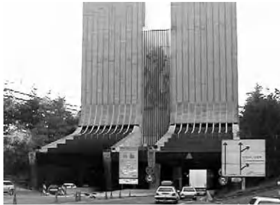
Figure 4.11. The Fourvière tunnel, Lyon
