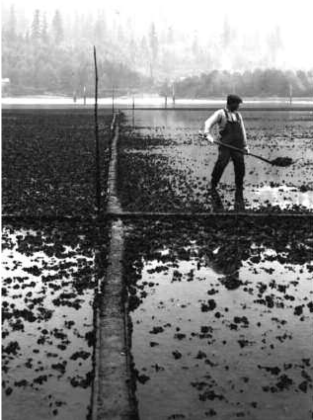
Oyster farmer repairing an oyster dike on the Pacific coast of America in the 1930s. Oyster dikes are constructed to control water depth and levels of sedimentation.
