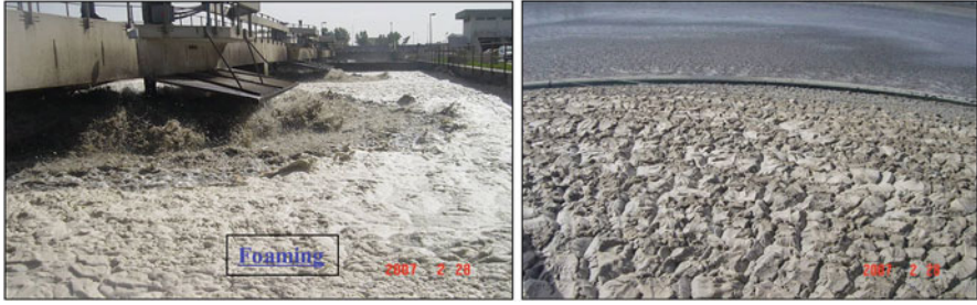
Fig. 4.2 Conventional aeration tank ( left ) and extensive foaming observed in the activated sludge process of Dubai’s sewage treatment plant, Dubai-UAE. ( Courtesy: Dubai Municipality, DSTP Division)
