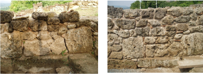
Figure 3: Historic masonry before (left) and after (right) restoration.
