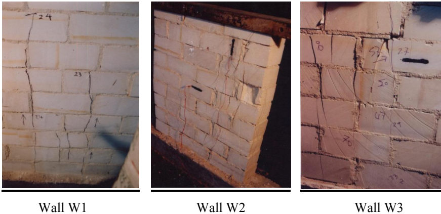
Figure 5: Crack pattern at failure of single leaf wall structure.
