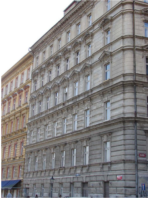
Figure 1: View of the assessed building.
