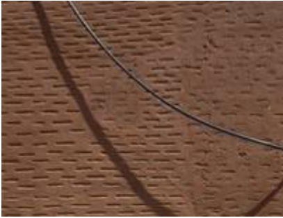
Figure 3: Image of the wall.
