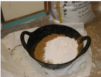
Figure 14: Gypsum mortar preparation.
