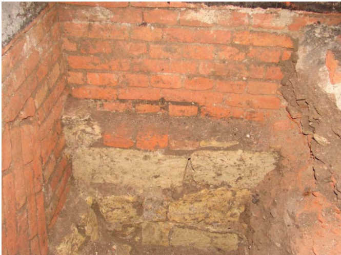
Figure 2: Masonry of a wall and foundations.
