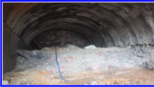
Figure 2. Whole section excavation of the lower bench.
