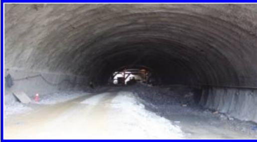
Figure 3. Step excavation of the lower bench.
