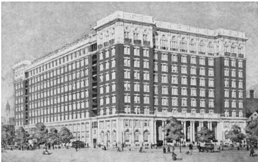
Figure 1.1 The Curtis Publishing Company building in Philadelphia.
