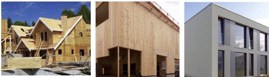
Figure 1.14 Natural fibre composite hybrid building system (left = wood composites, middle = cross-laminated lumber and right = composite construction).
