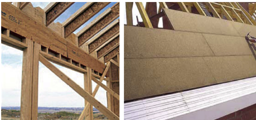
Figure 1.7 Natural fibre composites for roofing construction (left = I-joist and right = fibre board blocking).
