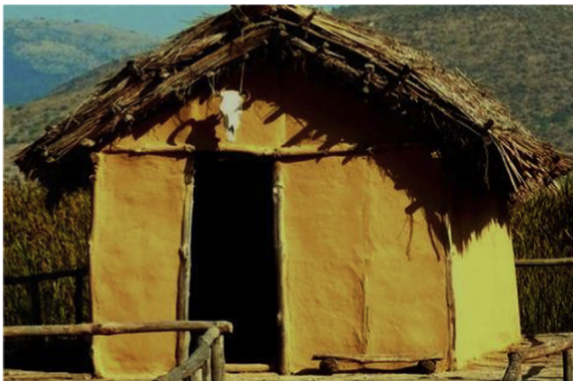
Figure 9.1 Representation of traditional application of natural fibre rebar: clay wall with reed reinforcement in Dispilio, Kastoria Lake, Greece (settlement older than 5000 BC).
