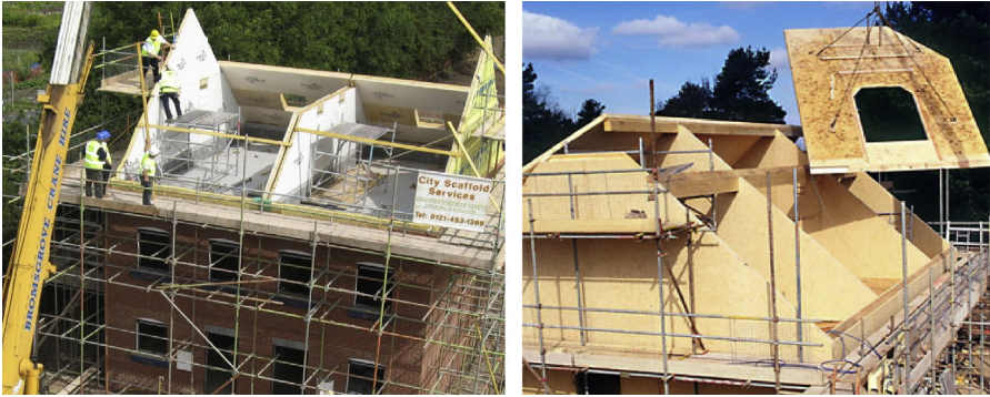
Figure 1.8 Off-site roofing components in building construction.
