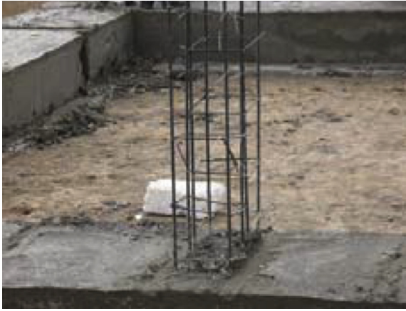
Figure 9.9 Use of basalt composite bars in seismostation in Lanzhou, China.
