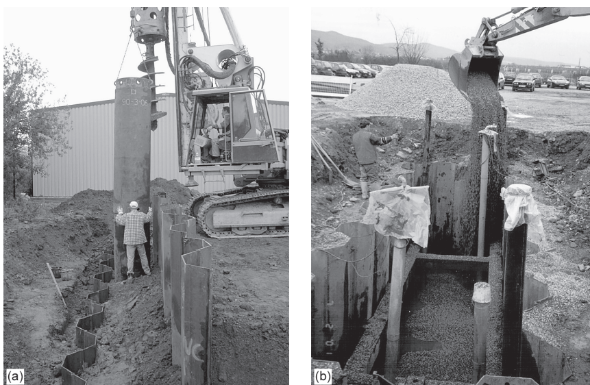
Fig. 3.9. Edenkoben. (a) Set-up of the vertical drainage system using a large-diameter borehole construction method. (b) Filling the gate with \text{Fe}^0 . (Courtesy of Peschla & Rochmes GmbH, Dipl.-Geol. Rochmes (Dipl.-Ing. Woll))
