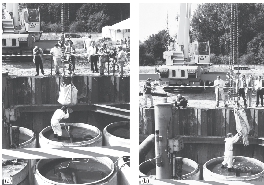
Fig. 3.2. Charging the last gate segments with granular iron in Bernau (September 2001)
