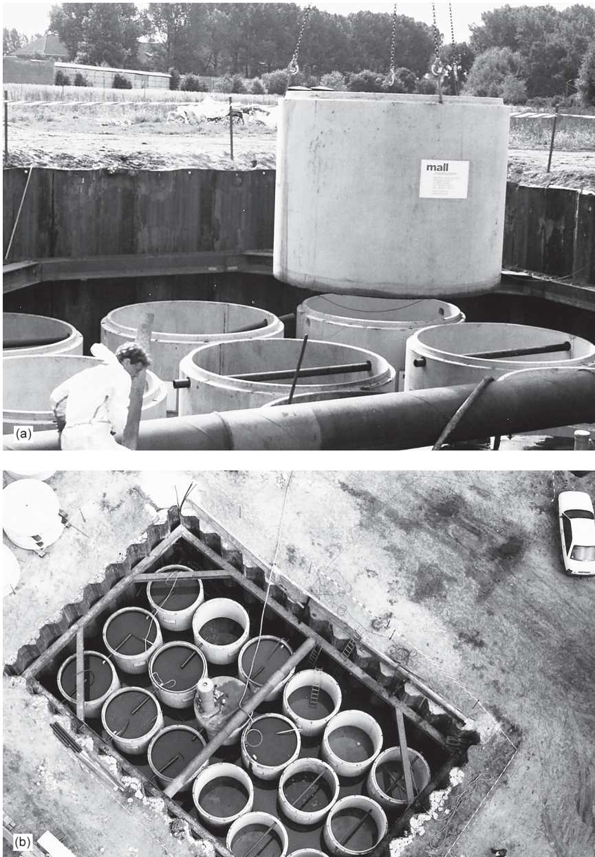
Fig. 3.3. (a) Fitting/installation of the single reactor segments and (b) overview of the whole gate construction of the Bernau PRB (September 2001)
