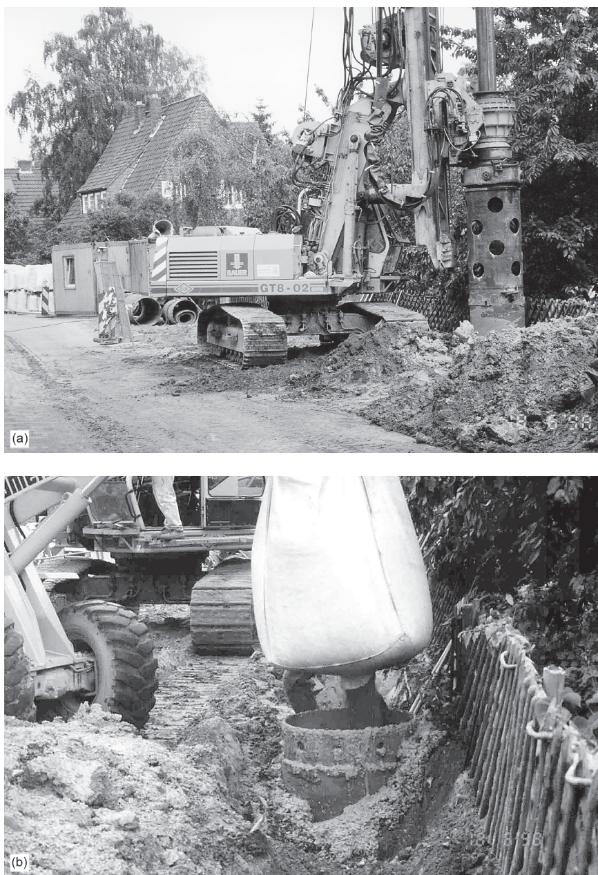
Fig. 3.17. (a) Set-up of the continuous wall in Rheine using the large-diameter borehole method. (b) Filling the borehole with reactive materials. (Courtesy of Mull und Partner Ingenieur GmbH (Dr-Ing. Möller, Dr Wegner))
