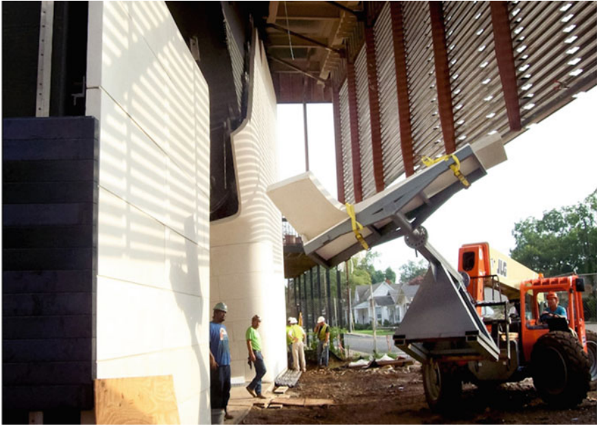
Fig. 4.41 Installation of the customized stone paneling (© 2011 CASE Design, Inc.)
