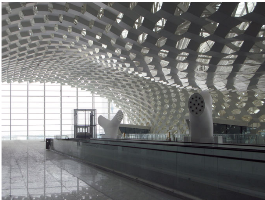
Fig. 4.26 The interior is strongly characterized by the dynamism of the punctured tube which acts as walls and roof (Courtesy of © Archivio Fuksas)
