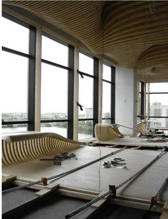
Fig. 4.45 Ceiling and benches during the installation (Reproduced with permission of dECOI)
