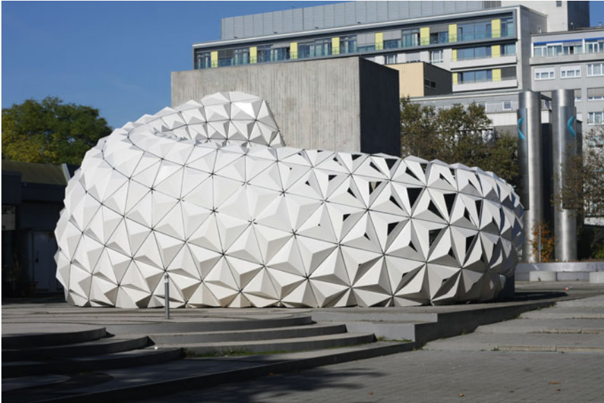
Fig. 4.19 Arboskin Pavilion built with bioplastic components (Reproduced with permission of ITKE, Courtesy of Manfred Richard Hammer)
