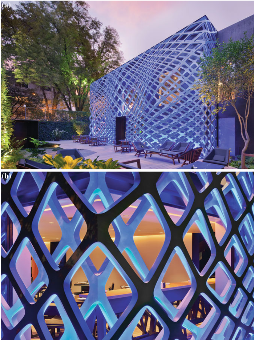
Fig. 4.9 a External view: a 1920s house has been wrapped by a digitally handcrafted cladding (Reproduced with permission of Rojkind Arquitectos, photo by Paul Rivera). b Detail of the metal cladding: slightly offsetting the layers and painting them two tones of gray , give the illusion of movement enhanced by the blue LEDs lights during the night (Reproduced with permission of Rojkind Arquitectos, photo by Paul Rivera)
