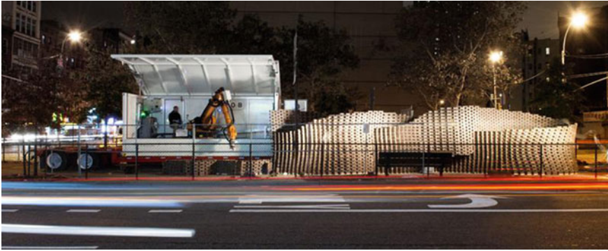
Fig. 3.8 Pike Loop, A Robot-built installation in NYC—Gramazio & Kohler, pioneers in the use of industrial robots in the construction field (Courtesy of ETH)
