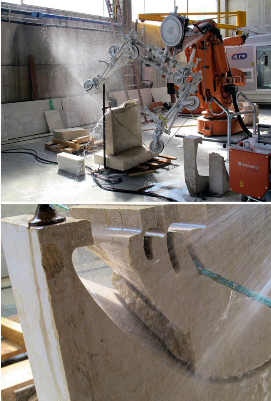
Fig. 3.19 Robotic Diamond Wire Sawing (RDWS) uses a diamond wire in order to fabricate marble pieces (Courtesy of Jelle Feringa)
