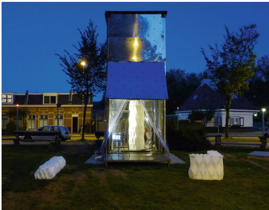
Fig. 4.37 The 3D printed components of the 3D Print Canal House are produced directly on site by the KamerMaker (Reproduced with permission of DUS Architects)
