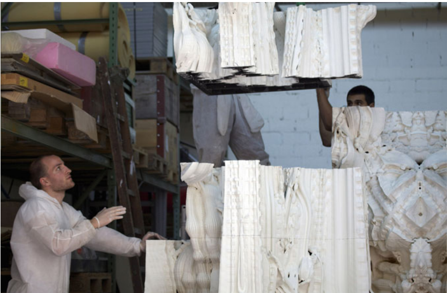
Fig. 4.51 The whole room has been printed in six large elements, designed to be transported and assembled together (Demetris Shammass, Achilleas Xydis)
