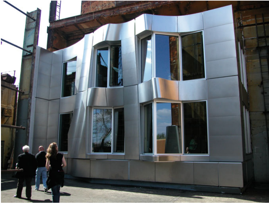
Fig. 4.18 Mockup of the cladding system (Reproduced with permission of Gehry Partners, LPP) Gehry Partners, LLP
