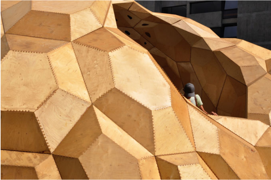
Fig. 3.21 ICD/ITKE Research pavilion 2011 was realized with just 6.5 mm thin plywood sheets connected through differentiated finger joints (Courtesy of © ICD/ITKE University of Stuttgart)
