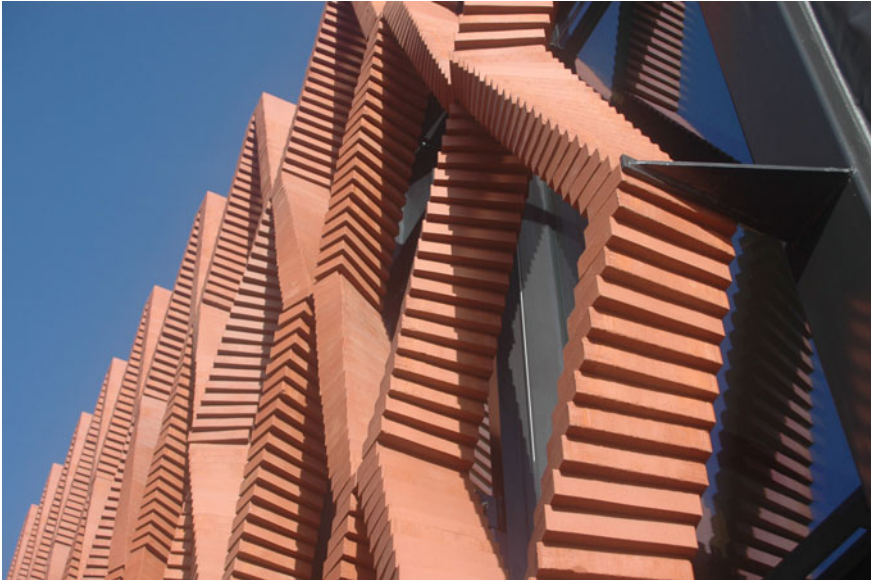
Fig. 4.5 The design of the façade would have been almost impossible to realize by a human (Reproduced with permission of © Gramazio & Kohler)
