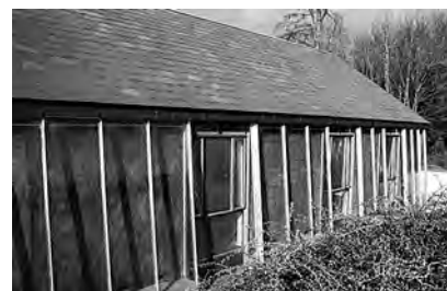
4.4 Trombe-Michel principle applied to Irish agricultural cottage in Carlow – south façade
