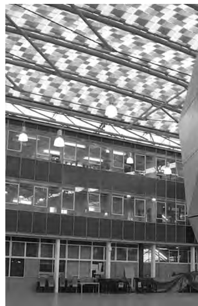
6.5 ETFE canopy at Kingsdale School – note artificial lights inside while outside is sunlit
