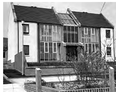
1.3 First Scottish passive solar housing in Stornoway by Western Isles Islands Council
