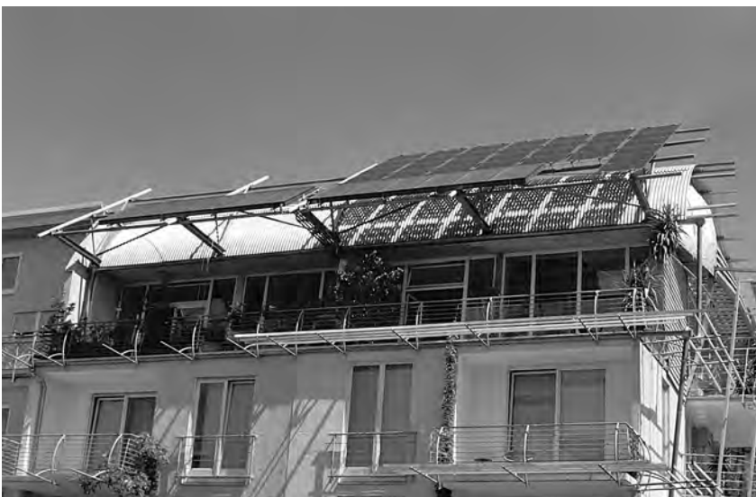
2.19a Terraced housing in Niewland, Amersfoort – PV arrays on flat roofs are not visible
