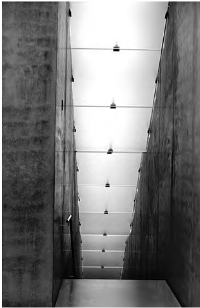
5.6 Kunsthaus in Bregenz a detail of glass rain-screen at external corner on sunny day b looking down staircase, with indirect daylight through ceiling on sunny day
