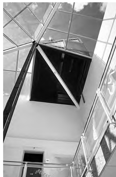
5.15a Looking up 'shark's fin' tower of atrium at Wasa City at Gävle
