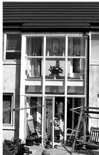
4.13 Semi-recessed, double-height sunspaces at Ballantrae
