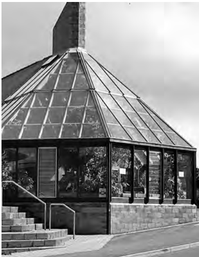
6.14 Winter garden located on top of boiler house at Kilwinning
