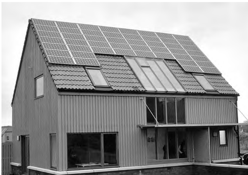
4.9 Solar house at Ayton with double-height, recessed glazed sun-porch
