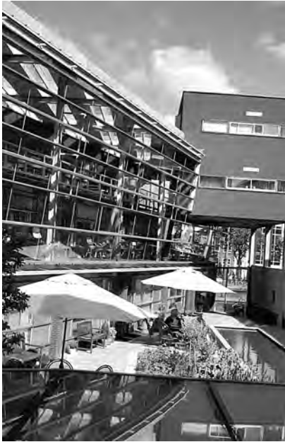
3.1a Looking east in Gravinnehof (mid afternoon in August) – glass roof of communal lounge in foreground and glass and timber screen to access promenades to left
