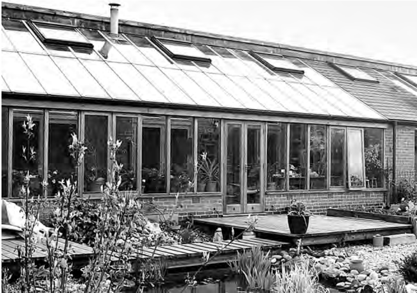
3.7 The south façade of one of the Hockerton houses – late morning in April before PV array added on top of the wall between sunspaces and heated rooms
