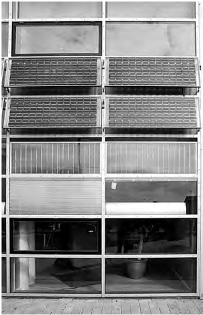
5.20 Detail of south façade of Brundtland Centre in Toftlund with glazing hierarchy, noting the twin array of PV panels between floors
