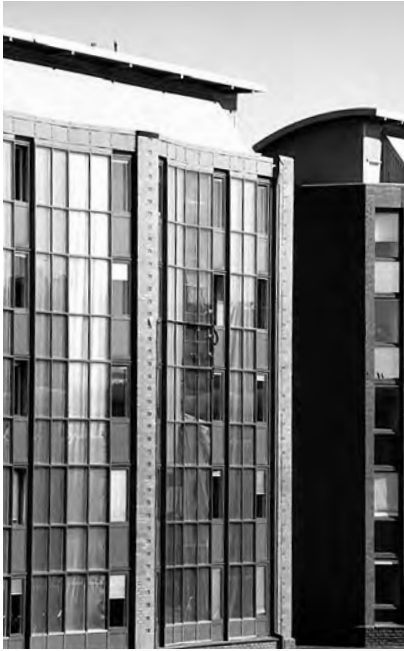
4.6 Solar TI façade of a student residence in Glasgow, facing slightly west of south
