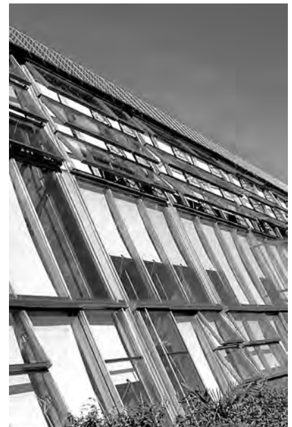
2.3 Solar terrace in Zollikofen, Berne: a PV array visually echoes opening windows at top of façade b blanked by blinds in warm weather
