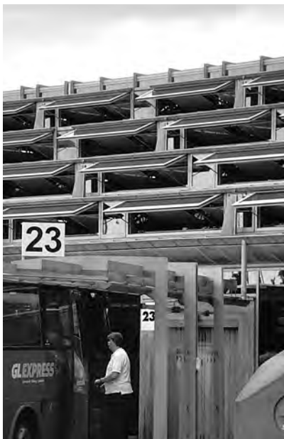
5.11 Bus station at Göteborg a inside concourse looking north-north-west – note asymmetric cross section b west-south-west façade, with stepped cascade of windows in open position
