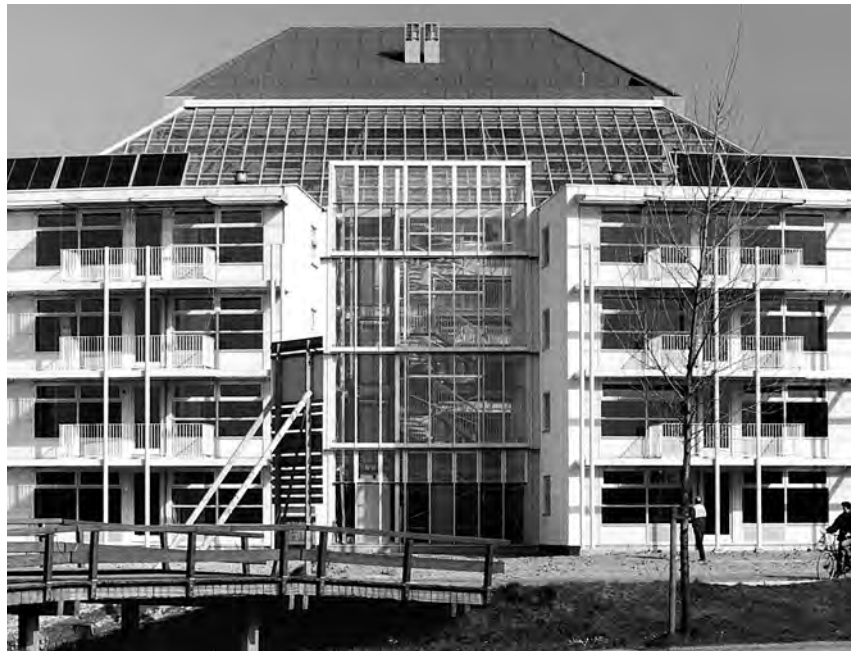
6.18 General view of south façade of Task XIII solar apartment block in Amstelveen
