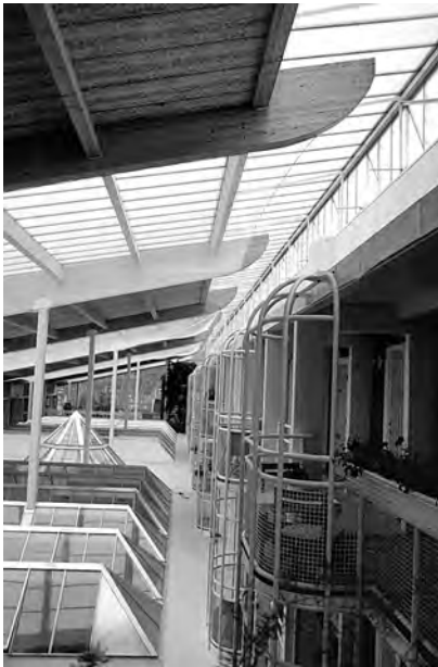
2.14 New atrium between old terraces at Söderhamn – note second layer of glazing to servicing accommodation at ground level
