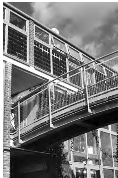
7.2 Part of south façade of BedZED terrace
