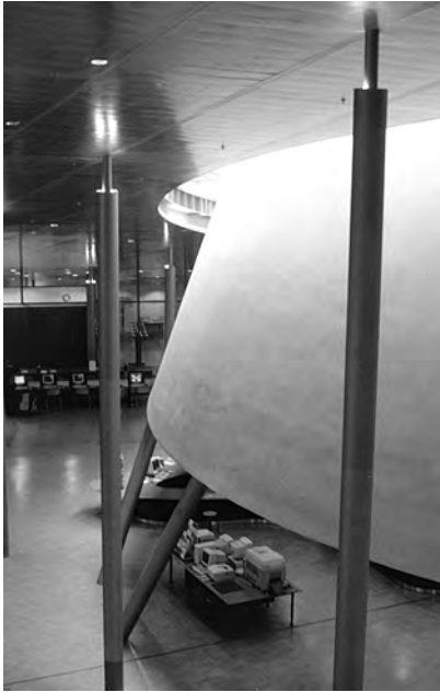
5.12 The cone sheds daylight deep into the library at Delft Technical University
