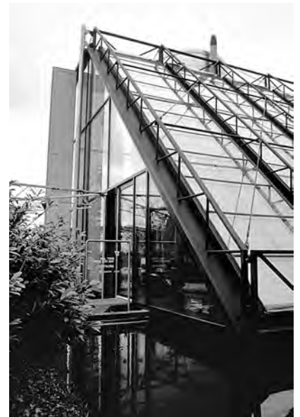
2.2a ‘Fantasy’ solar house in Almere: active flat-plate collector doubles as a south-facing roof
