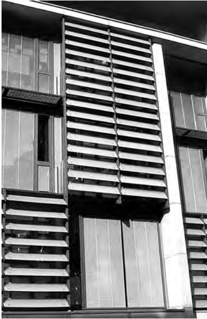
6.3 South façade of junior school in Glasgow, showing glass louvres and glazing with integral venetian blinds – note pupils' work attached to glass
