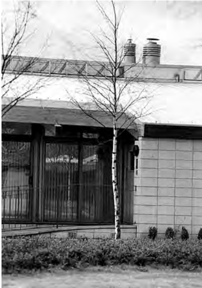
2.11 Southern façade of Scottish dementia unit
