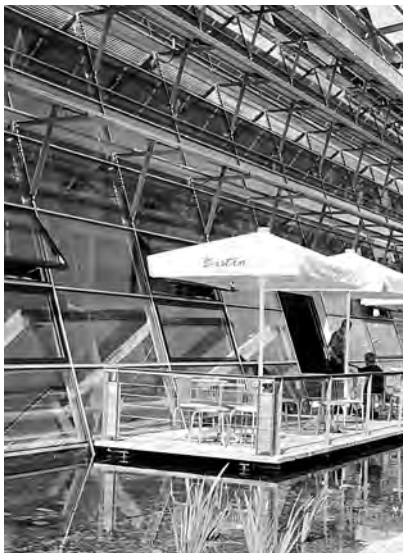
5.10 'Showroom' for PV factory in Freiburg – louvres functionally advertise the product
