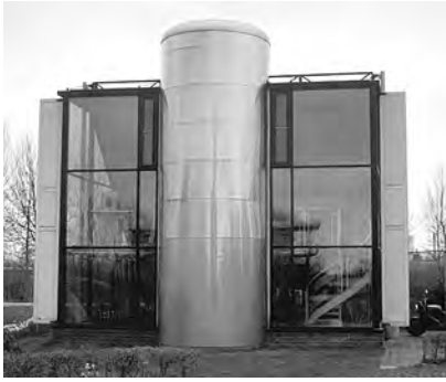
2.2b 'Fantasy' solar house in Almere: seasonal thermal store makes a statement on the public side of the house
