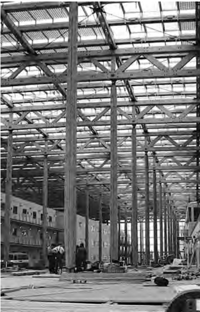
2.16 Inside Akademie Mont-Cenis during construction in the summer of 1999
