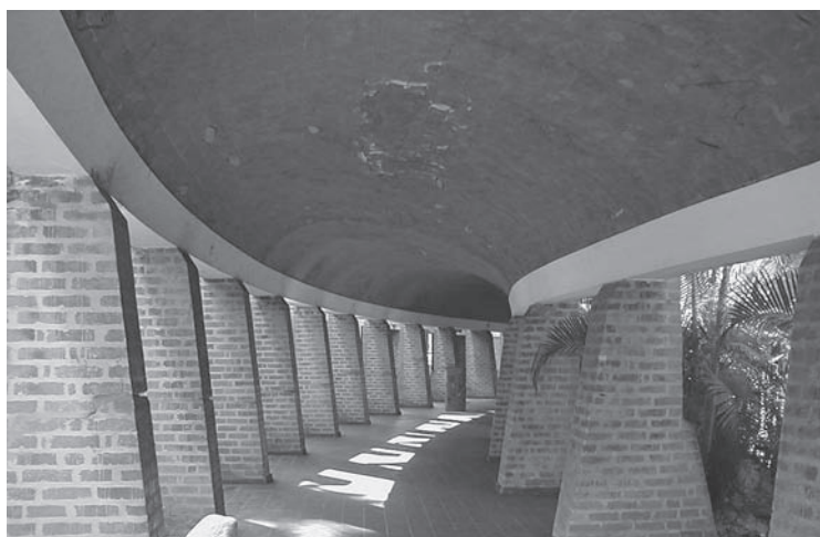
FIGURE 4.20. Cuba's Escuelas de Arte. One of the finest complexes built in Cuba since 1959. The schools are known for the use of local building materials that draw on red clays that characterize most of the island's soils. Terra-cotta materials and Catalan vaulted ceilings symbolize both the authenticity and optimism of the design. The domes seen in the top and bottom images grace the complexes, and are framed by concrete lattice sunscreens that serve as glassless "windows." High-vaulted domes (light colored, top image) allow for rising warm air to escape through the ceiling tops. These pod-like domes serve as art and dance studios. Cracked and flaking brick and tiles can be seen in the ceilings of both images, taken in 2004.
