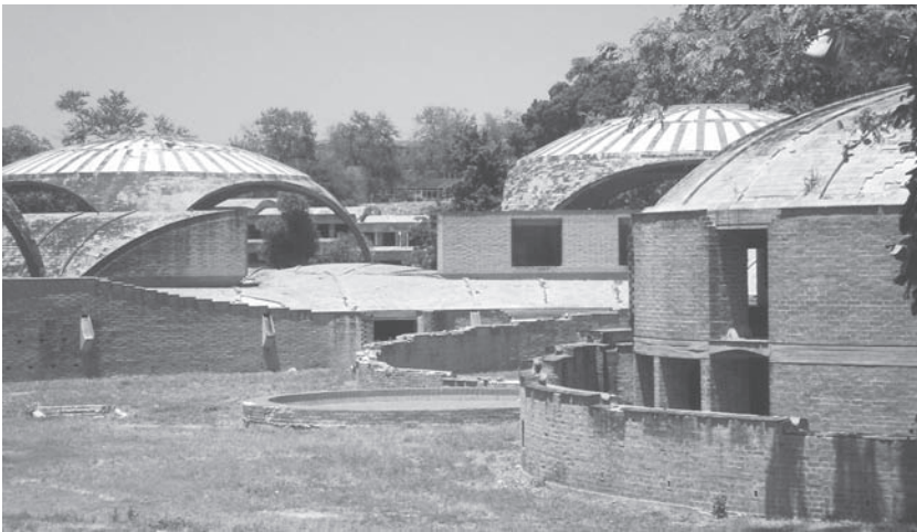
FIGURE 4.19. A portion of the incomplete Escuelas de Arte, in Cubanacán, western Havana City Province. Construction started in the early 1960s.
