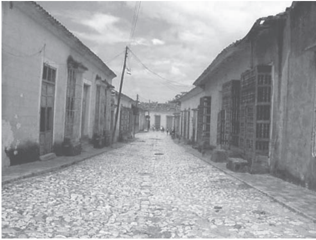
FIGURE 4.11. Many of the streets in Trinidad are built with a blend of local river rock and ship ballast from European ports.
