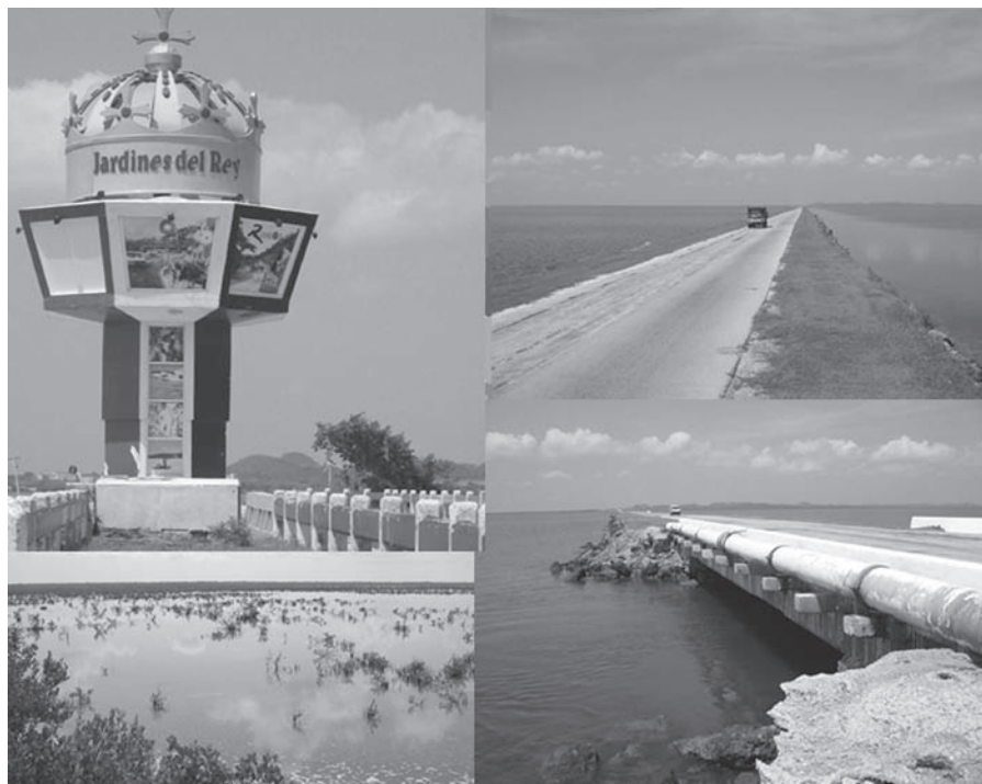
FIGURE 5.11. Cayo Coco Causeway ( pedraplenes ), 2004. Clockwise from upper left: Looking south from the Jardines del Rey “crown” entrance toward the mainland; a truck along the causeway; one of several intermittent underpasses allowing water to pass from west to east (note water main pumping fresh water from mainland to Coco Key); and marshland to the east of the causeway.
