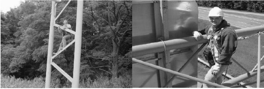
Fig. 16.8. Inspector climbing a structure using a double lanyard system, from (Federal Highway Administration 2005).
