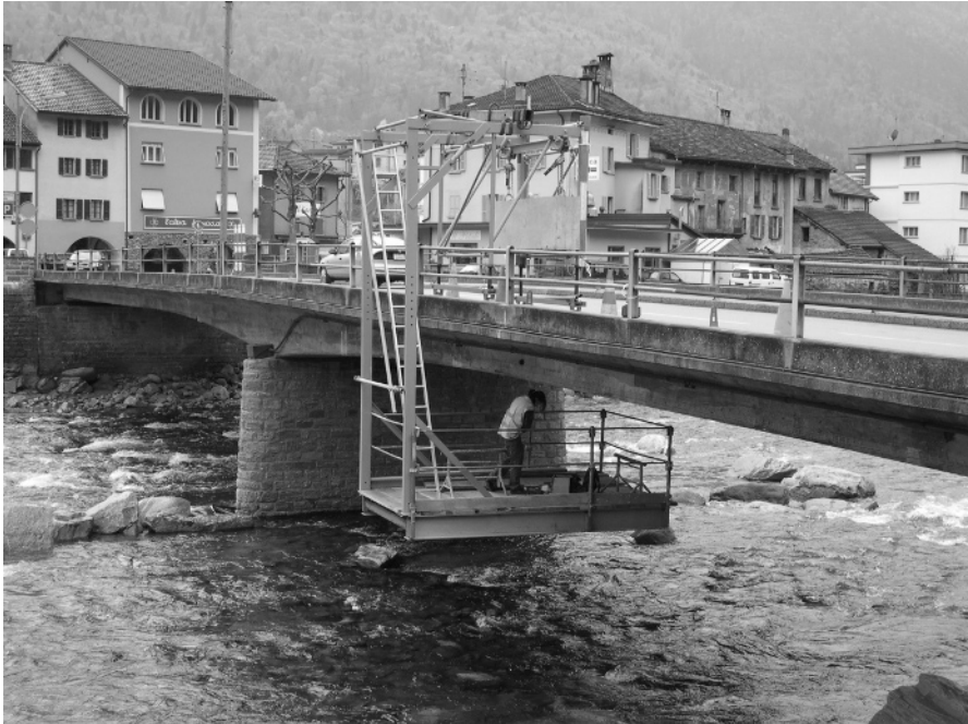
Fig. 16.7. Scaffold to access the soffit of a river bridge.
