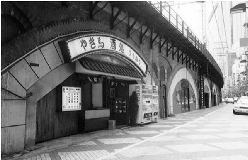
Fig. 14.24. Photo of a continuous arch bridge.
