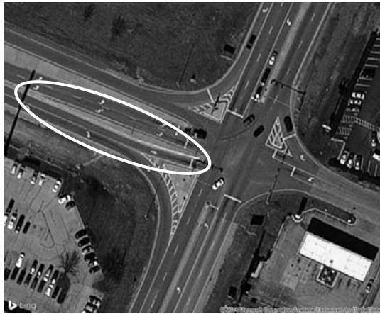
Fig. 4. Raised median for separating same direction of traffic on an exit ramp.
