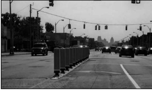
Fig. 3. Application of longitudinal channelization in restriction of left-turn access (Morena and Ault 2013).
