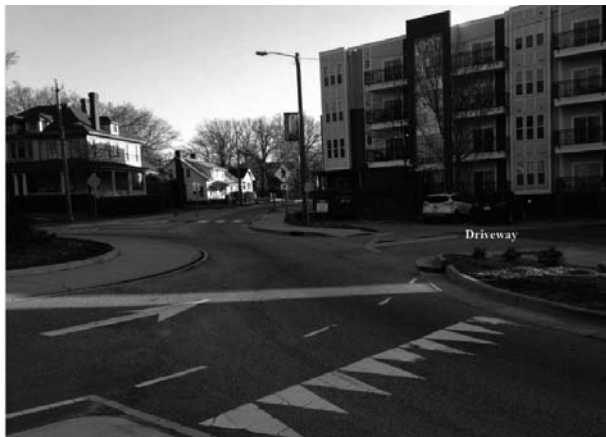
Figure 5. A Case Study: Roundabout with No Slip Lane and a Driveway off Hillsborough Street and W. Morgan Street, Raleigh, NC – Scenario S2 (with a Driveway).
