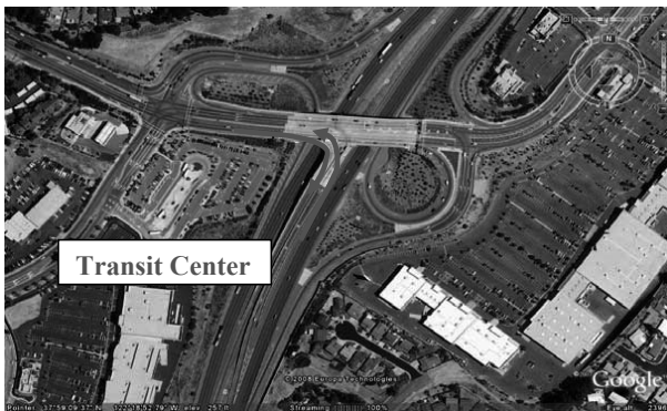
Figure 5. Transit dedicated access ramps.
