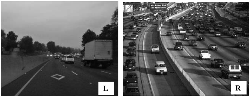
Figure 2. A HOV lane contiguous with mixed-flow lanes.
