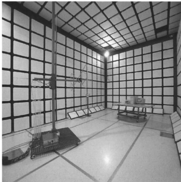
Figure 2.1 EMC semianechoic chamber.
