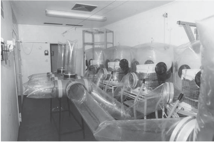
Fig. 7. Distribution system with four isolators connected to the distribution steel pipe.
