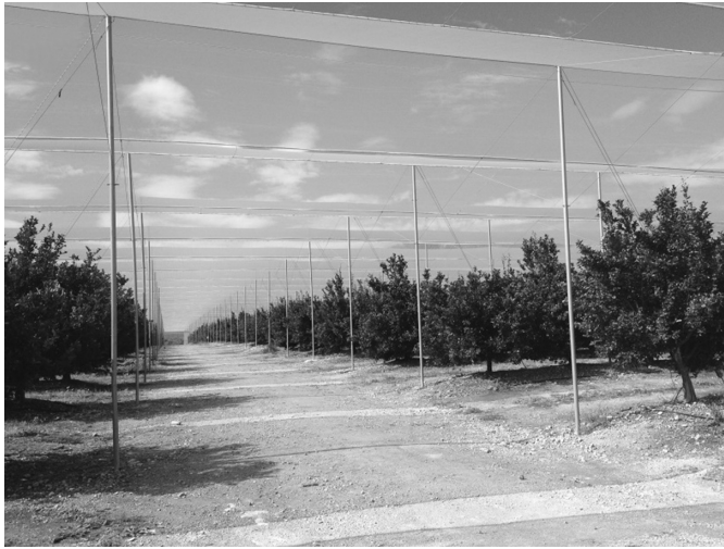
Figure 1.3 Shade House (Courtesy of ININSA Greenhouses, www.fabricanteinvernaderos.com/english/ ).
