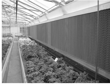
Figure 5.95 Cooling Pad (Courtesy of Dr. A.J. Both, Department of Environmental Sciences, Rutgers University, USA).
