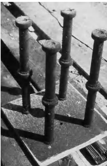
Fig. 2.13 Steel embed plate with welded headed studs
