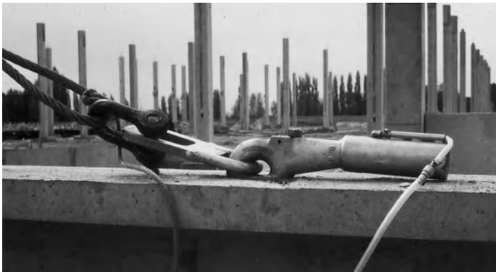
Fig. 2.6 Round-headed transport anchor
