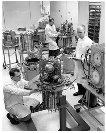
Figure 16 Pratt & Whitney technicians assemble alkali fuel cells for Apollo service modules, 1964.<sup>40</sup>
