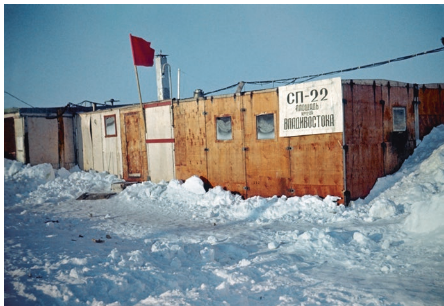
Fig. 14.7 Main complex of several interconnected prefabricated huts on drifting station NP-22 in May 1977. Developed by Russian designers Kanaki and Ovchinnikov, these comfortable mobile huts were officially termed PDKO after them, with PD standing for polyarny dom (in Russian) or polar house. The complex included mess room, kitchen, food storage, recreation room, and sauna. The sign reads: “NP-22 Vladivostok Square” after icebreaker Vladivostok , which together with M/V Captain Kondratiev delivered supplies, including the huts, for the first party of 10 in September 1973. The huts were assembled onboard before the ice camp was set up on the ice island (Photo by Igor Belkin)
