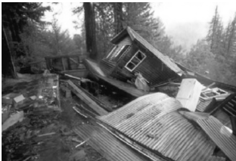
FIGURE 9.4 Aftermath of the Loma Prieta Earthquake Source: http://pubs.usgs.gov/dds/dds-29/
