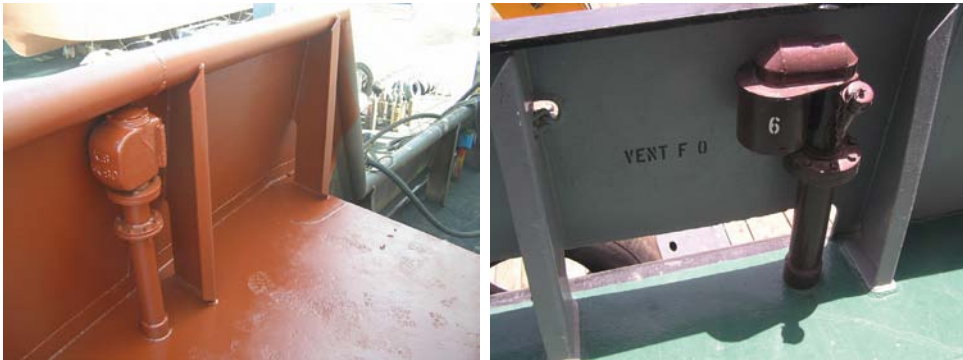
FIGURE 148 DB tanks' ventilators.
