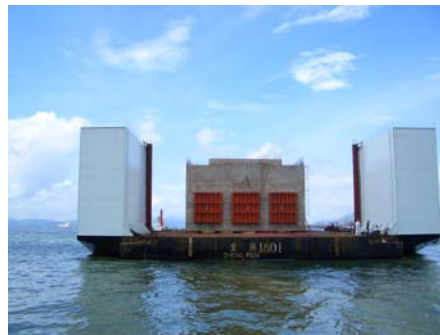
Figure 6. Fitting the caisson in place
