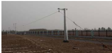
Figure 4. Prototype model of four poles and three span conductors
