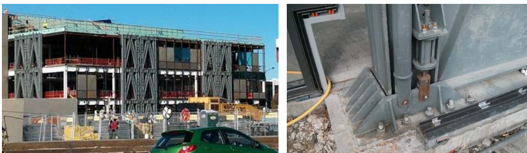
Figure 3 Kilmore Street Medical Centre, Christchurch, New Zealand: (left) view of building; (right) bottom corner of controlled rocking frame [photos by first author, May 2013]
