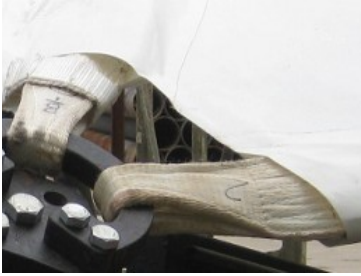
Figure.8 Polyester belt end with the membrane material processing
