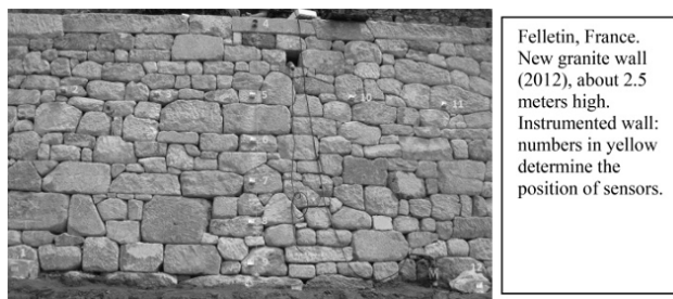
Figure 11.5. Drystone retaining wall masonry can be considered under plane strain, built by companies included in the ABPS 1 . Instrumentation is part of the PEDRA 2 project, photograph by Joachim Blanc-Gonnet
