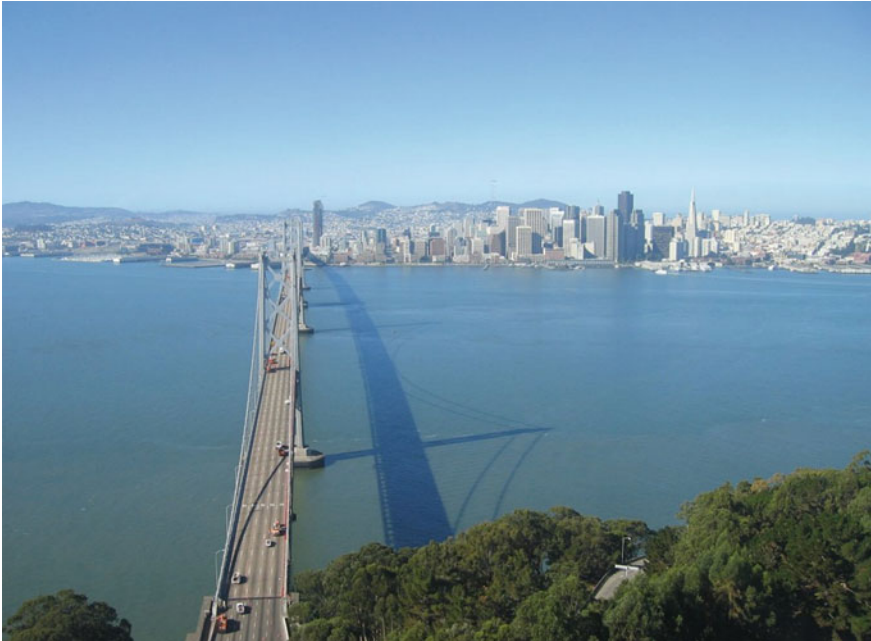
Fig. 2.1 The Oakland–San Francisco Bay Bridge, which was closed for one month following the 1989 Loma Prieta earthquake. Source Dan Bluestein, Wikimedia Commons
