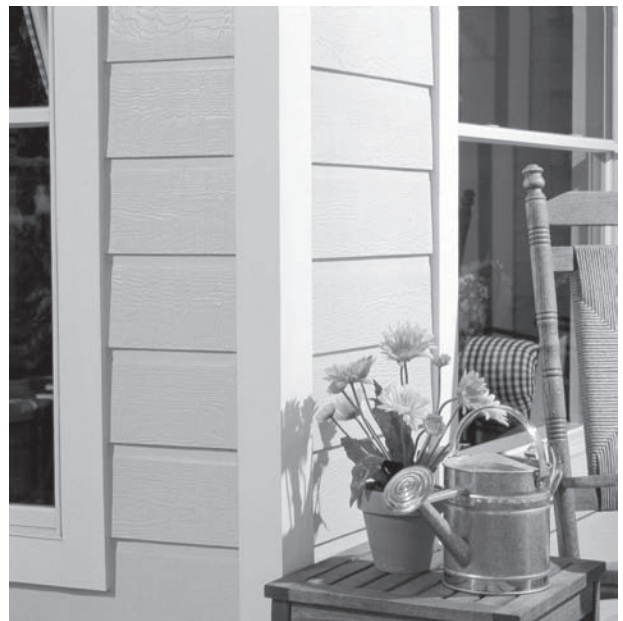
Figure 26-5. Fiber cement siding is made to look like wood siding but is more durable. Courtesy of James Hardie Building Products.
