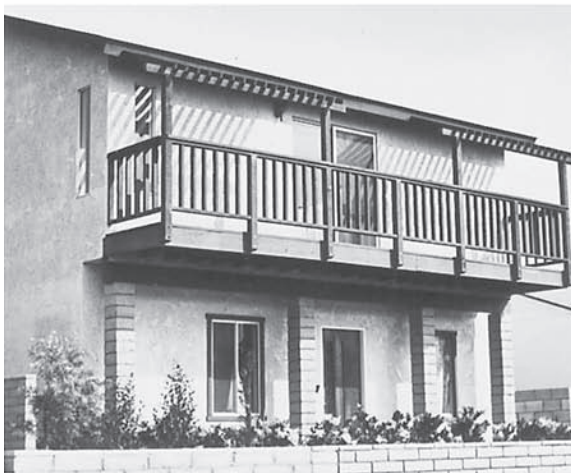
Figure 17-12. Typical uses of cantilevered framing.
