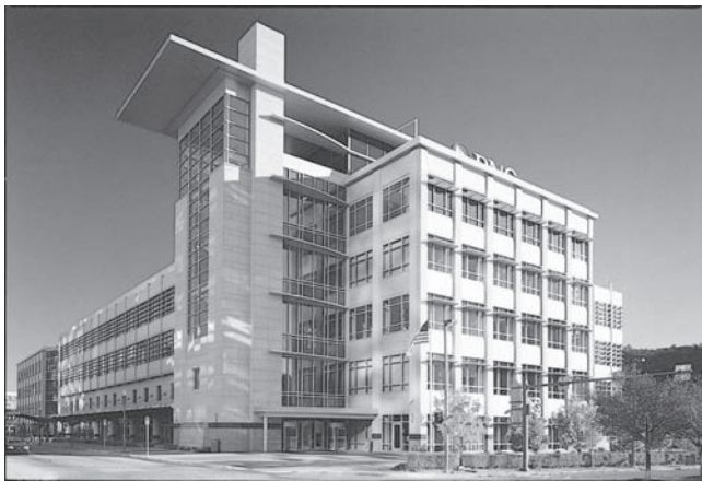
Figure 1-1(B). Commercial construction.
