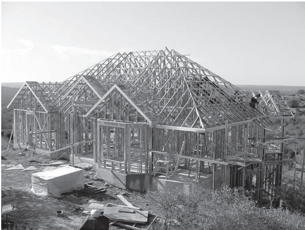
Figure 15–16. Metal framing. Courtesy of Dietrich Metal Framing.
