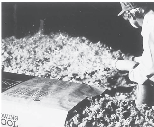
Figure 31-5. Blowing wool. Courtesy of Owens Corning Fiberglas Corporation.
