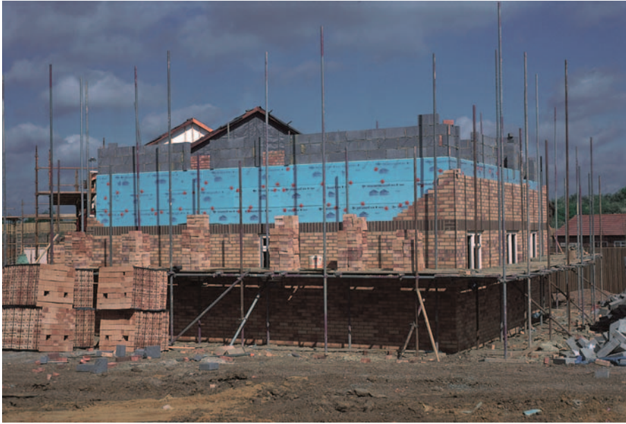
FIG 7.2 A traditional brick and block house under construction in the same estate as the house in Fig. 7.1.
