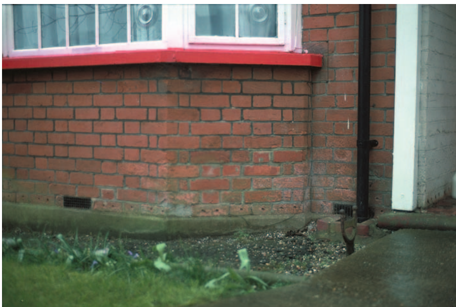
FIG 4.10 Drill holes at the base of the wall indicate that a chemical injection damp-proof course has been added.
