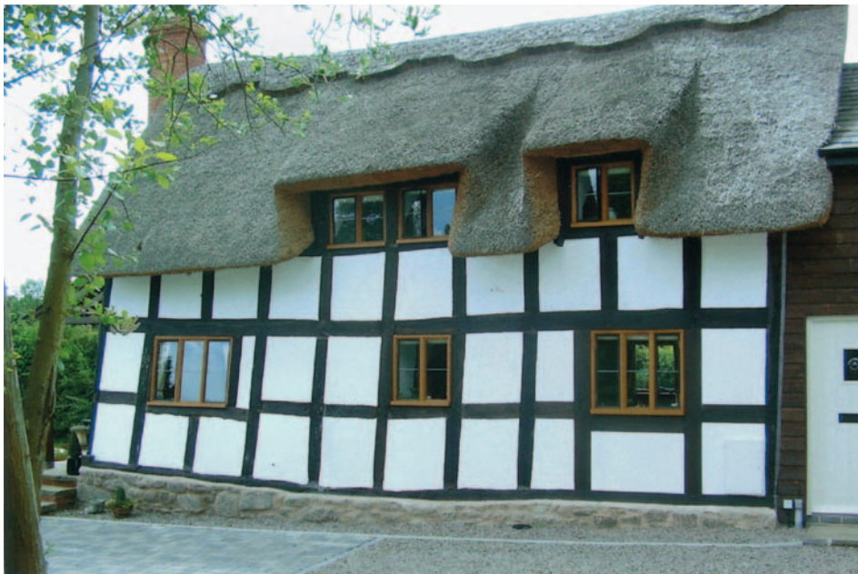
FIG 15.1 A “black and white” house in Herefordshire. A framework of oak wallplates, studs and beams provides the strength with an infilling of single skin brick, cob or wattle and daub. Timbers are morticed and tenoned using oak pegs. Walls are finished off inside and out with a lime render and lime wash. The structure sits on a stone pinning. Similar building methods were used throughout the middle ages. In Lincolnshire these houses are referred to as “Stud-and-mud” with a cob infilling generally used, and this type of construction crossed the Atlantic and was used by the first English settlers in Jamestown, Virginia.
