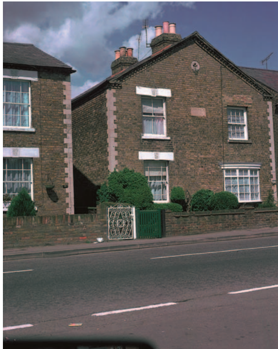
FIG 21.4 The arch over first floor window has spread and the lintel has dropped. This section of wall will need to be rebuilt.
