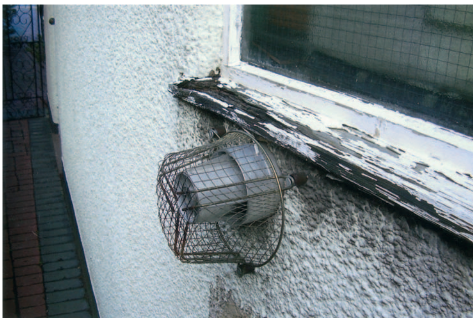
FIG 9.2 The location of this balanced flue directly under the window sill would not comply with current regulations. The discharge of flue gases – mostly water vapour – has had a predictable consequence in the form of wet rot to the window woodwork.
