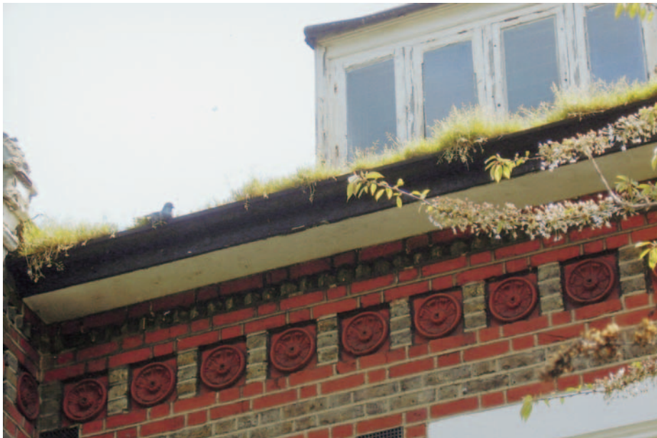
FIG 21.6 The grass growing in this gutter results from years of neglect. Sometimes conservation is just a matter of common sense.
