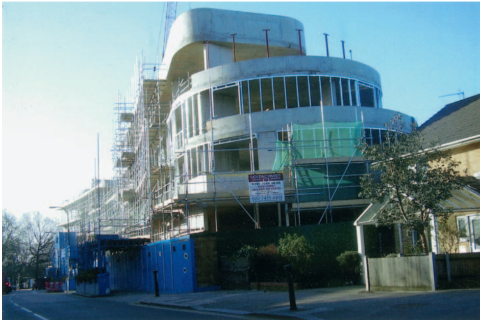
FIG 12.1 Concrete is artificial stone and ferrous reinforced cast-in-situ concrete construction makes use of some fortuitous chemistry. Steel reinforcement encased in Portland cement concrete does not normally rust, being protected by the alkali cement so provided that the depth of concrete covering the steel bars is satisfactory and so long as deleterious chemicals such as chlorides, sulphates or high alumina cement are not present, this type of construction is very durable. It also presents architects with the facility to incorporate slender columns and curved cantilerved elevations as in this building under construction in north London.
