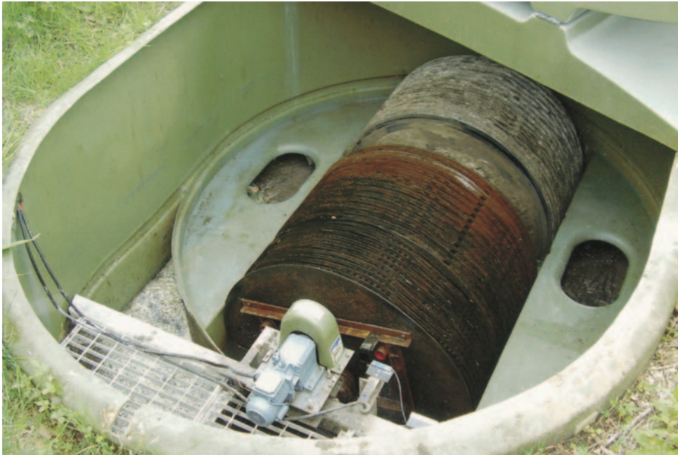
FIG 9.4 When mains drainage is not available a modern alternative is the Klargester Biodisk septic tank drainage system. Effluent enters the system and is rapidly broken down by bacteria with the process hastened by the electric motor and rotating disks which increase the exposure to oxygen in the air. The treated effluent emerging from the system is clear water suitable for draining into soakaways or an adjoining water course. Consent to discharge effluent is required from the Environment Agency. Periodic de-sludging is necessary.
