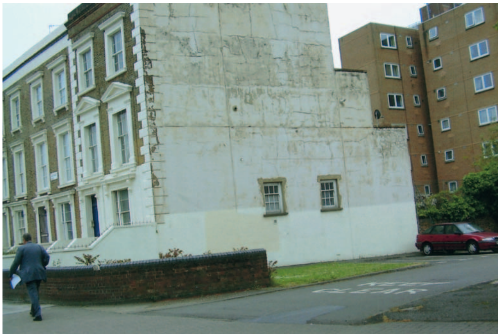
FIG 4.3 Stucco render has been applied to the flank wall of this London terrace. Poor preparation of the wall behind with inadequate keying, trapped moisture and the wrong mix, badly applied, combine to produce this unfortunate result. The builders need to hack it all off back to the brickwork and then start again. Many of these flank walls in London have resulted from Second World War bomb damage, so that part of a terrace has been demolished and something has to be done to weather-proof the exposed wall.
