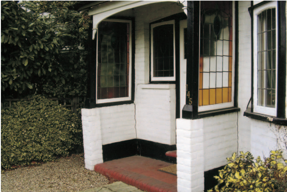
FIG 3.17 Builders will often use a very shallow foundation for a porch thinking that because the weight is low they do not need to excavate as deeply as for the main house; this is not so and the porch in this case will need to be rebuilt on deeper footings.
