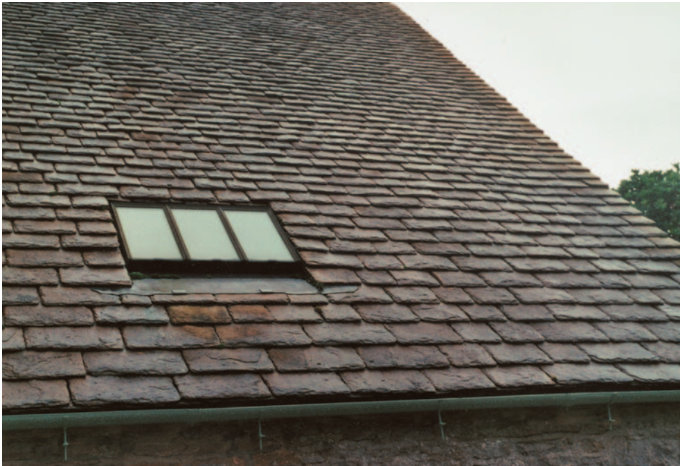
FIG 6.2 Cotswold stone roof with skylight and lead apron. Careful attention to detail is needed if leakage around skylights is to be avoided.
