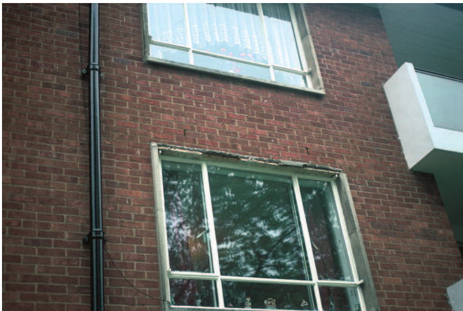
FIG 4.9 Inadequate cover for steel reinforcement in concrete lintel. Rust can take up to seven times the space of the steel it replaces causing bursting to the concrete surface.
