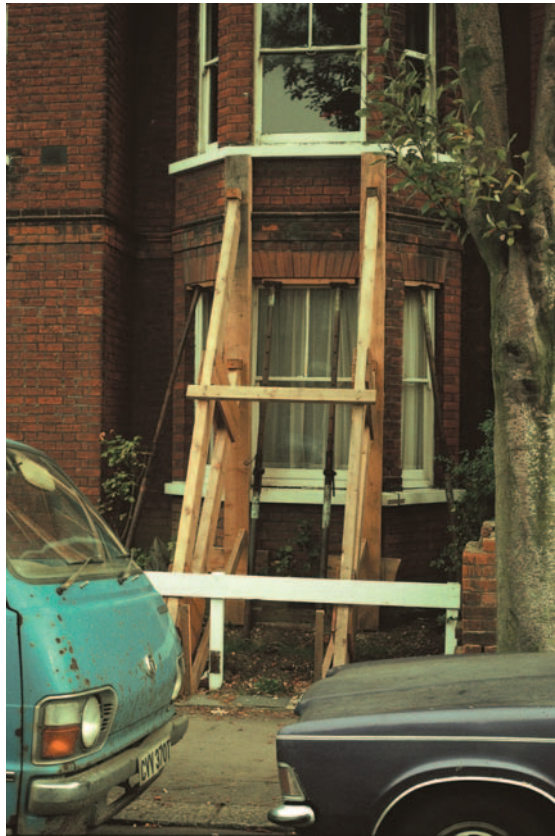
FIG 4.2 Raking shores used to support bay suffering from subsidence pending repair. Note the tree.
