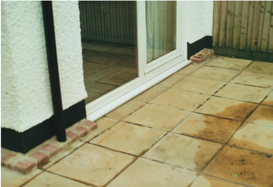
FIG 4.17 The paving is too high. It should be lowered to at least 150 mm (2 brick courses) below the damp-proof course or internal floor level whichever is the lower, with a slope away from the wall.
