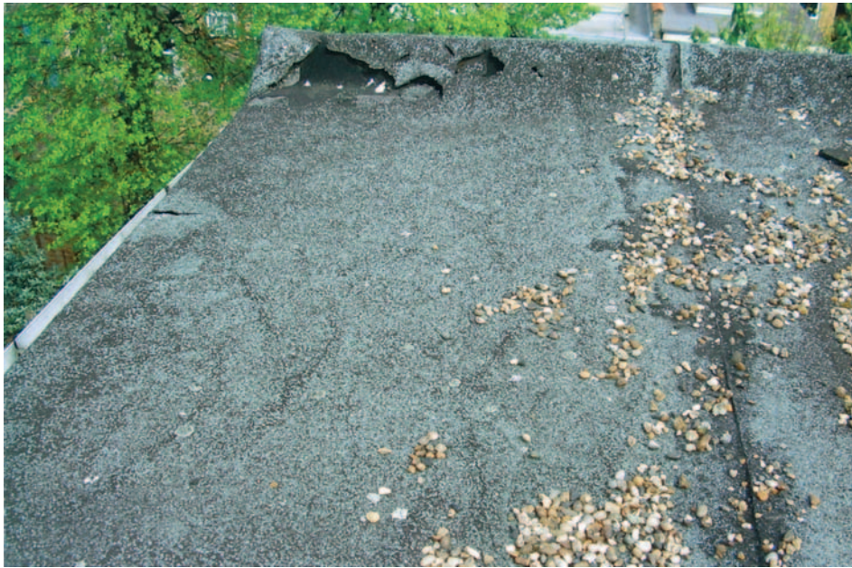
FIG 6.3 A flat roof surfaced in three layers of built-up mineral felt to British Standard 747. Typical life expectancy is less than 10 years. A number of important matters cannot be confirmed without exposure including the condition of timbers, insulation, ventilation under the decking and the presence or otherwise of a vapour barrier. Take care when walking on one of these roofs – the decking may be rotten, and collapse is possible. Watch out for holes cut in the ceiling beneath for downlights, or similar; these can provide a mechanism for warm damp air from the interior to pass into the roof void condensing on timbers and causing premature flat roof failure.
