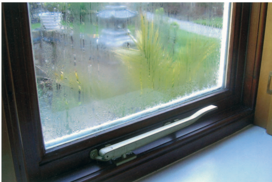
FIG 2.5 Condensation between the glass in double-glazed sealed units generally arises when the windows are between 10 and 20 years old, often (and conveniently for the manufacturers), just after the 10-year guarantee period has run out. The sealed units then have to be replaced. The cost/benefit and payback calculations for double glazing need to reflect the fact that these windows are not maintenance free. During a Building Survey, it is necessary to check any condensation on the glass to see if it is inside, outside or between the panes. If it is between the panes, there is likely to be a developing problem with the windows which could be expensive for the client.
