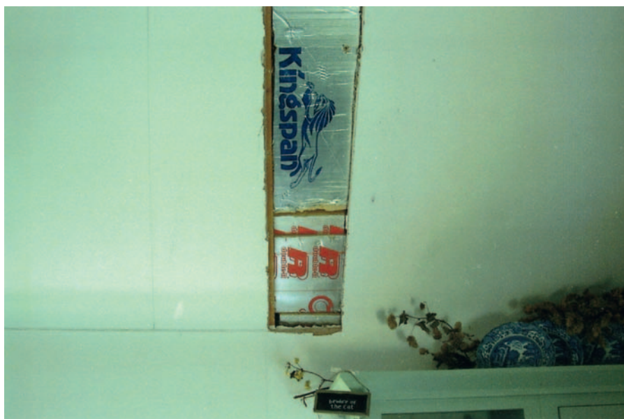
FIG 11.2 A section of plasterboard to a sloping ceiling is removed revealing Kingspan foam insulation panels. Normally, the actual level of insulation above a ceiling cannot be confirmed in these circumstances because there is no access behind. So, the computer program used to provide an energy rating makes certain assumptions based upon the age of the property and the Building Regulations applicable at the time it was built. This presupposes, of course, that the property is correctly dated and that the builders complied with the Regulations.
