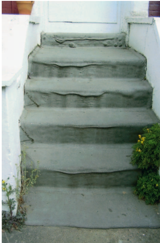
FIG 6.5 Asphalt is used for flat roof covering, basement tanking and as a waterproof surface coating to steps if there are vaults or other accommodation beneath. Vapour blowing and creep can be a problem. Creep to the asphalt on these south-facing steps results from poor preparation and application of the asphalt exacerbated by trapped moisture and exposure to the full heat of the sun.
