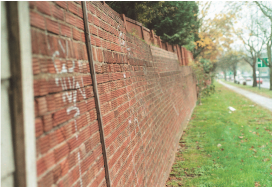
FIG 2.4 If leaning boundary walls have to be rebuilt this can be very expensive.
