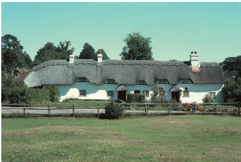
FIG 6.9 Hampshire thatch with eyebrow window details.
