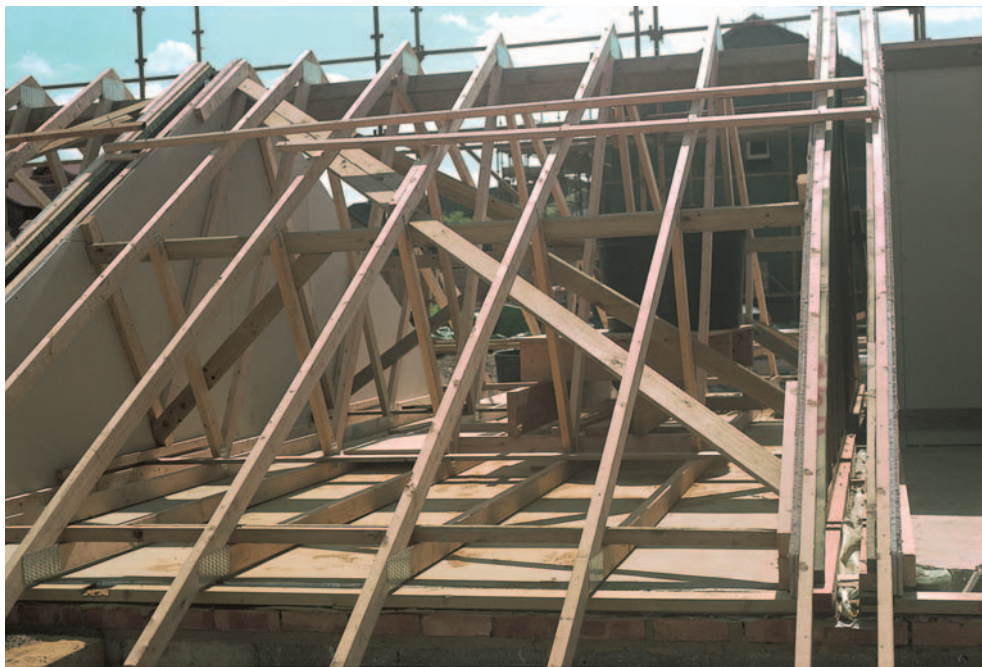
FIG 6.8 Modern gang-nailed trussed rafter roofs require diagonal bracing and gable-end strapping to prevent racking.
