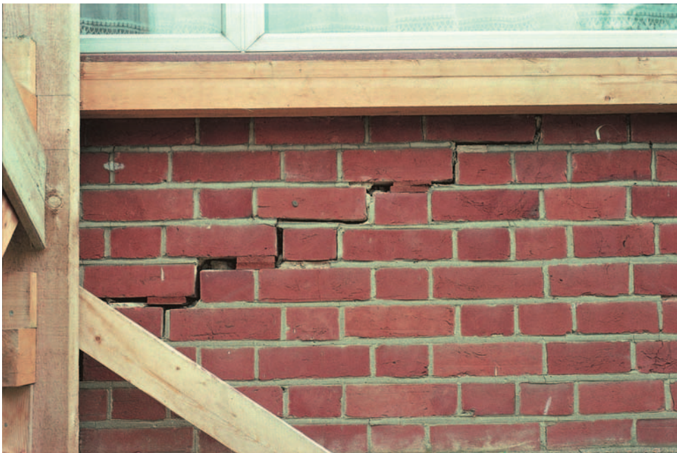
FIG 3.15 Subsidence has affected the lower part of this wall. As a temporary measure raking shores have been placed against the wall and hardwood wedges driven into the open bed joints to prevent further movement of the construction above.
