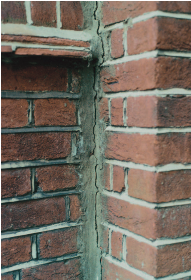
FIG 3.4 This settlement fracture has been poorly repaired and opened up again indicating continuing movement.
