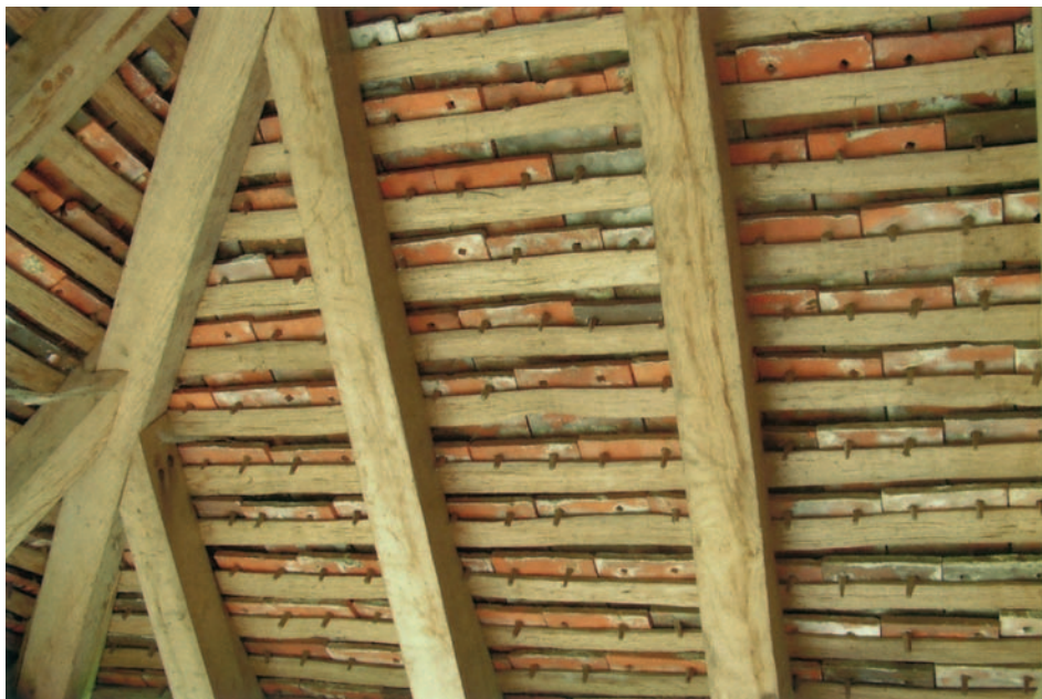
FIG 6.1 Double lap plain clay tiles held in place using traditional wooden pegs on battens with no underfelt. Pegs may rot or shrink causing them to fall out – as has happened to some here – then tiles slip. Tiles can be replaced and, if there is no underfelt, new pegs inserted from beneath, although then the pegs will taper the wrong way and need to be pinned to the battens. This type of tile was gradually superseded in the 19th century by plain tiles with nibs to hold the tiles on the battens. These plain tiles with nibs remain very popular today in both traditional clay and modern concrete form and incorporate nail holes just below the nibs so that they can also be nailed to the battens for an even more secure fixing.
