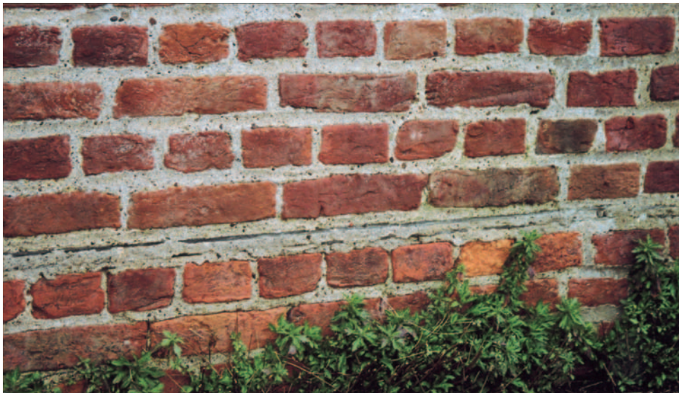
FIG 4.18 Hand-made red facing bricks set in lime mortar to English Bond with a two-course slate damp-proof course. Good ground clearance below the damp-proof course.
