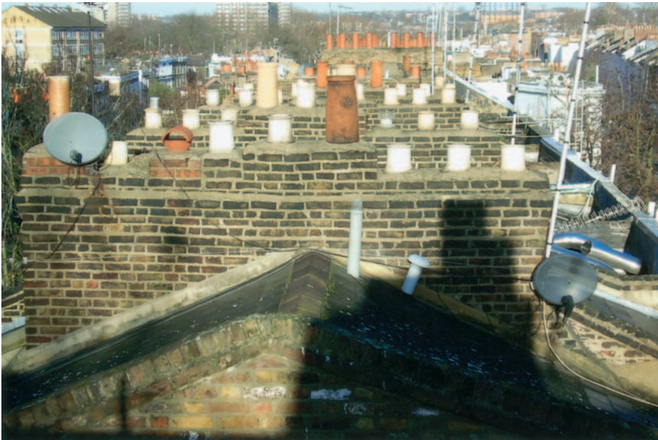
FIG 6.7 In Victorian London almost every room had a fireplace with the flues gathered together in shared chimney stacks over the party walls. Lots of scope here for downward damp penetration. Redundant flues should be vented at the base with hooded pots on top to keep them dry. Often only a limited view will be available from ground level even with the use of binoculars but many of these roofs have external trapdoors from the roofspace, especially the centre-valley or “butterfly” London roofs, so the surveyor can climb out onto the roof to view the construction at close quarters.
