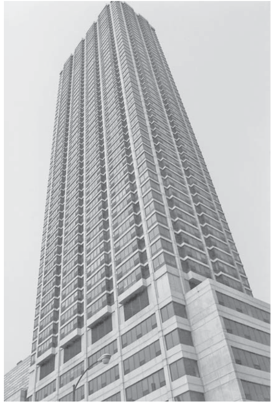
High-rise building, Chicago, Illinois.
