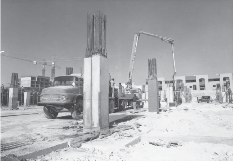
Reinforced concrete tied column under construction. The two columns are separated by an expansion joint.
