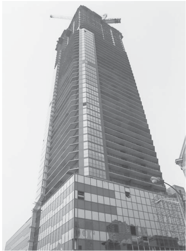
Office building under construction, Chicago, Illinois.
