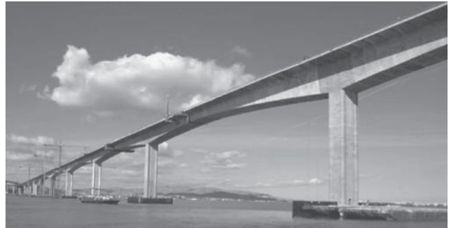
Benicia-Martinez Bridge, California.
