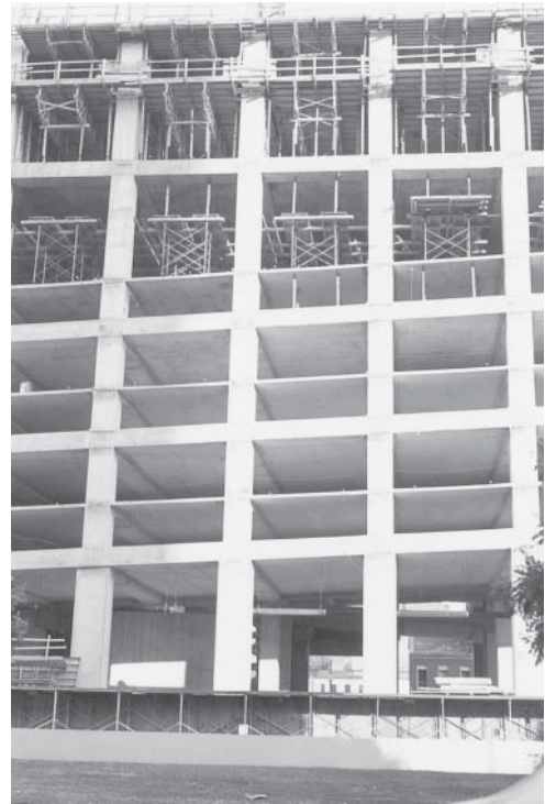
Continuous slabs in a parking structure, New Orleans, Louisiana.
