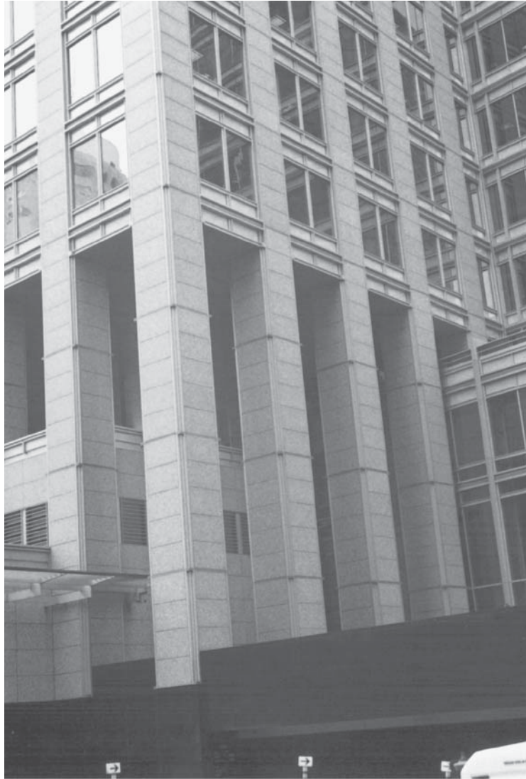
Long columns in an office building.
