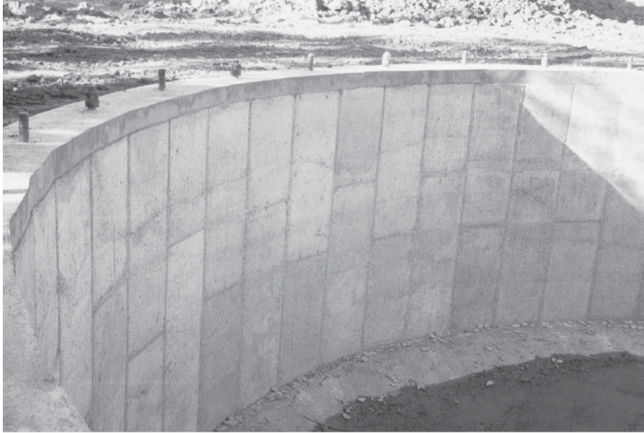
Reinforced concrete retaining wall.
