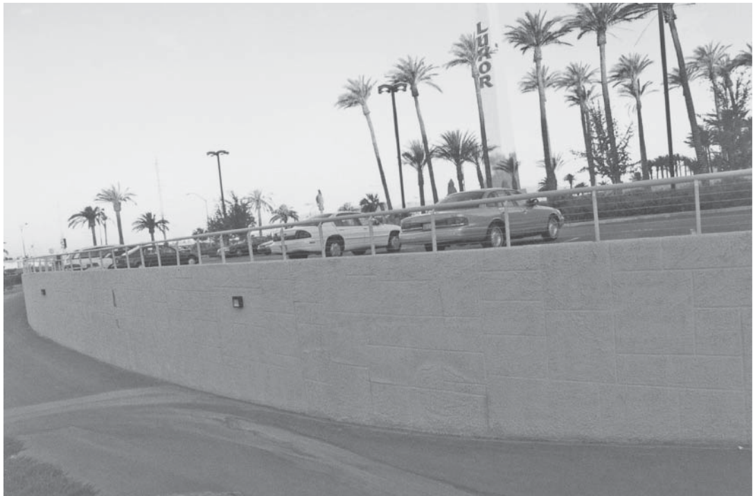
Retaining wall in a parking area.
