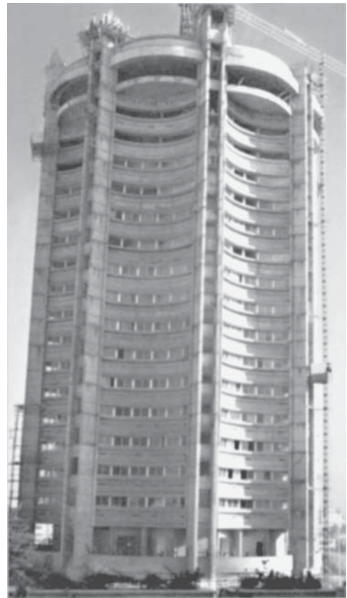
Curved beams in an office building.
