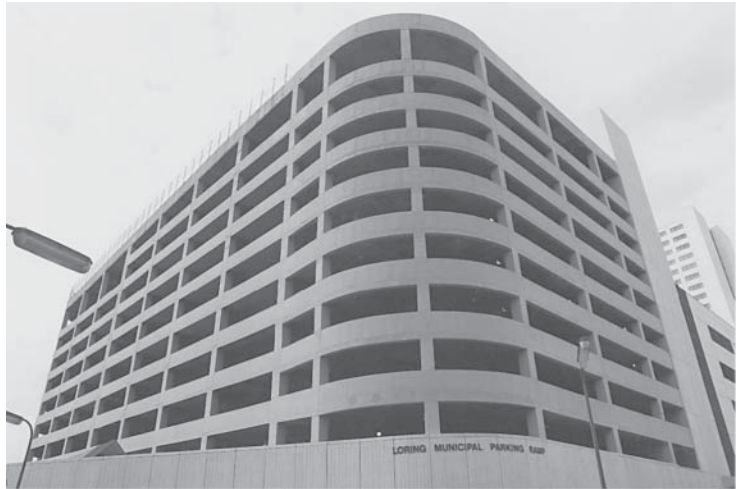
Reinforced concrete parking structure, Minneapolis, Minnesota.
