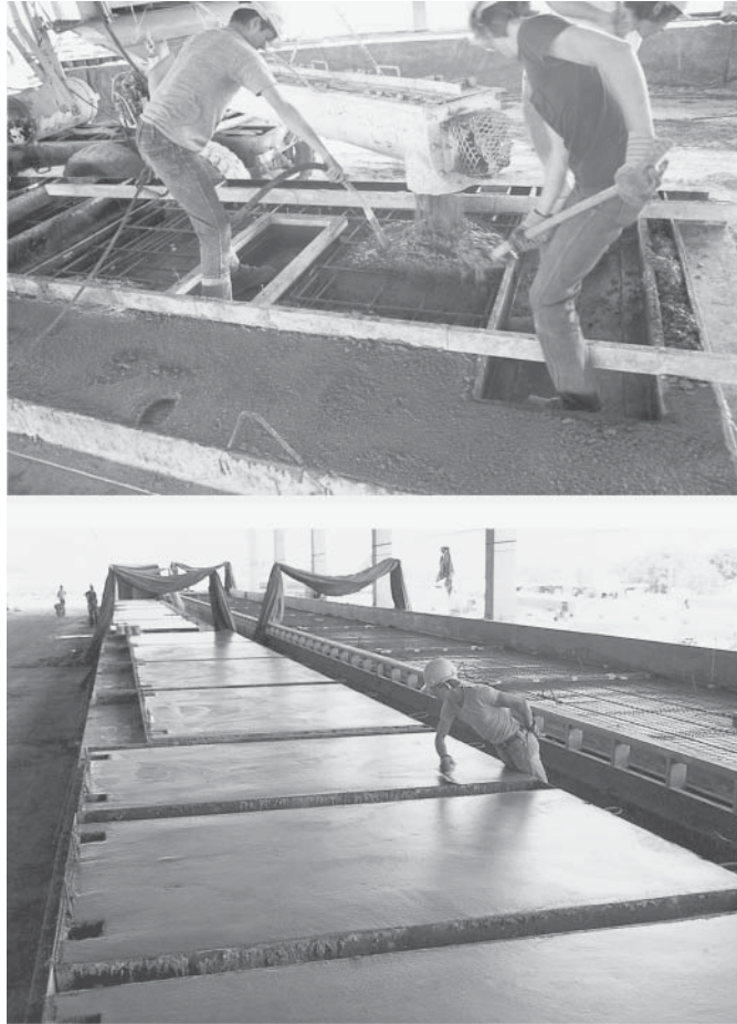
Casting and finishing precast concrete wall panels.
