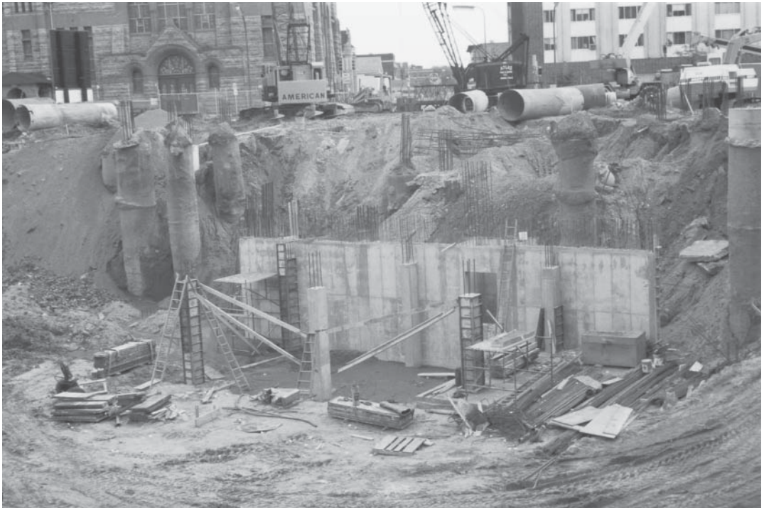
Wall and column footings, partly covered.
