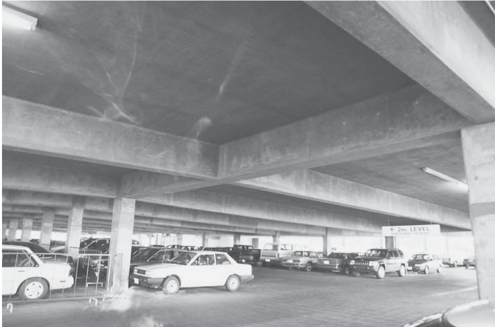
Slab on beams.
