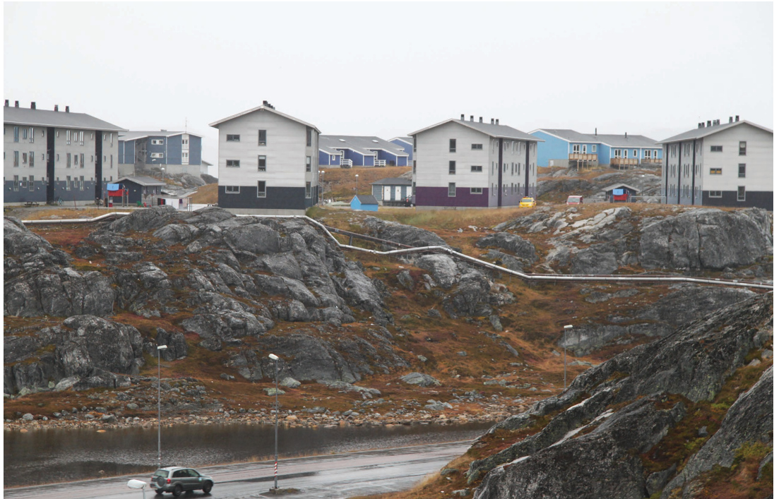
Figure 11.1 An insulated, heated, metal-encased water pipe zigzagging across the facets of the rocky terrain in Nuuk Photo: the author.
