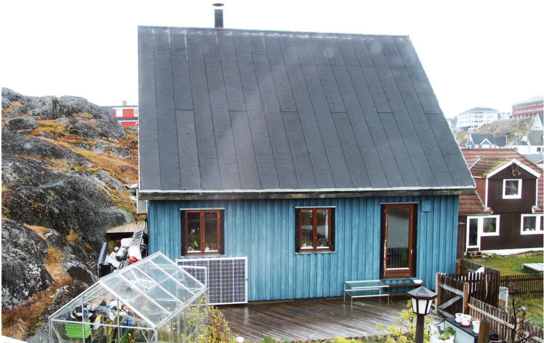
Figure 11.4 A private house in Nuuk with a casually mounted solar panel on its façade. As vertical mounting is needed due to the low sun angle, the façades of homes and buildings are altered through these additions.
