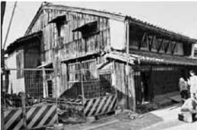
Figure 18.8 A traditional Nagahama house before renovation
