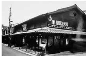
Figure 18.6 A Nagahama location after renovation
