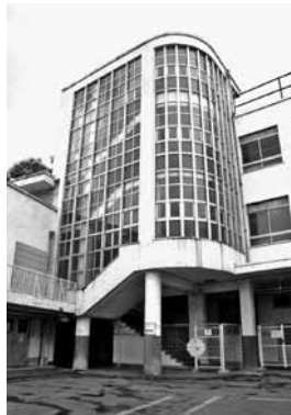
Figure 18.26 Yotsuya 5th Elementary School Provided by the Shinjuku Ward, Tokyo.
