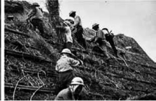
Figure 18.21 Repairing a thatched roof
