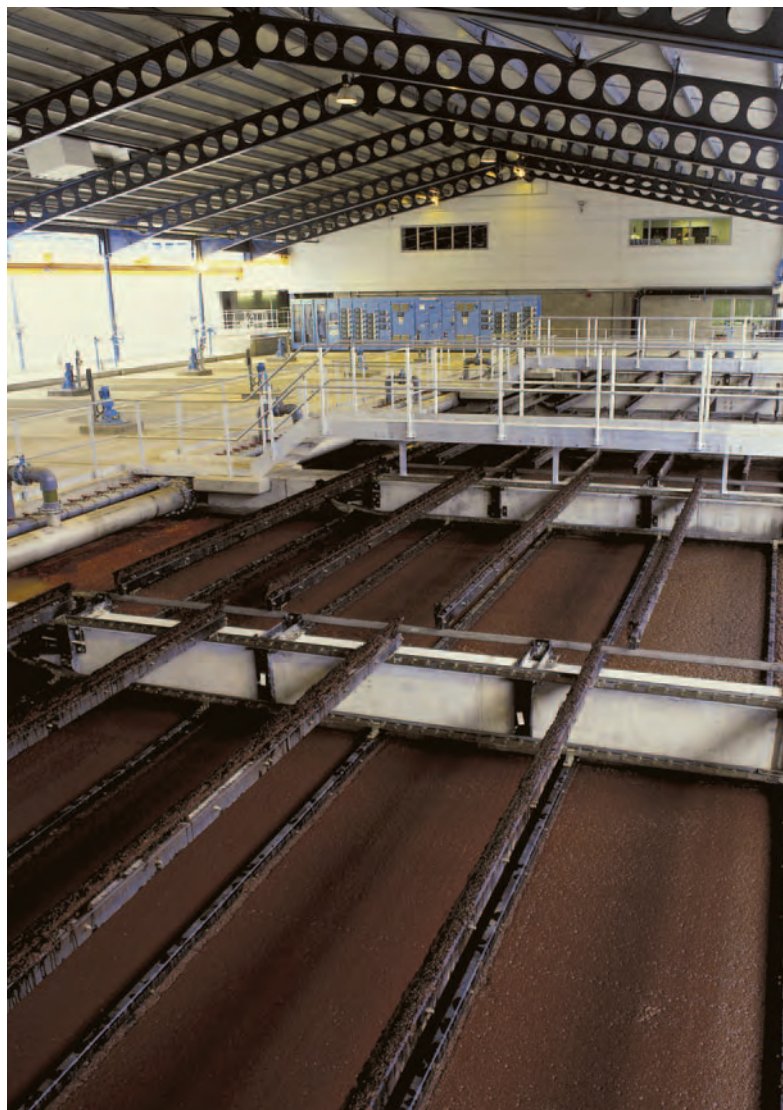
Every year, U.S. CSOs release more than 1.2 trillion gallons of raw sewage and wastewater prior to treatment.
