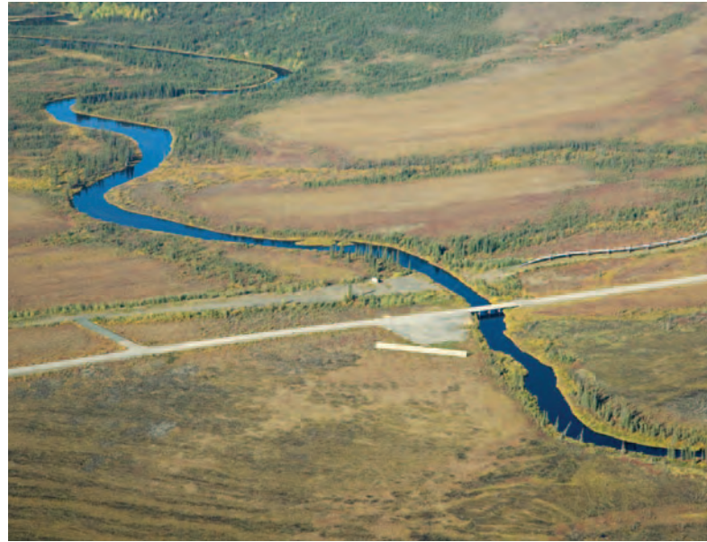
Constructed in 1977, The Trans Alaska Pipeline bisects the Kanuti River near the Dalton Highway.
