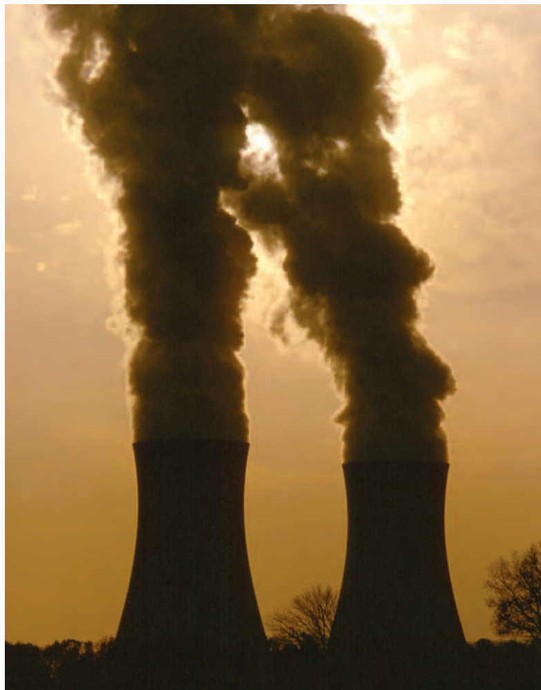
Since Three Mile Island in 1979, there has been no major nuclear power plant accident in the United States.
