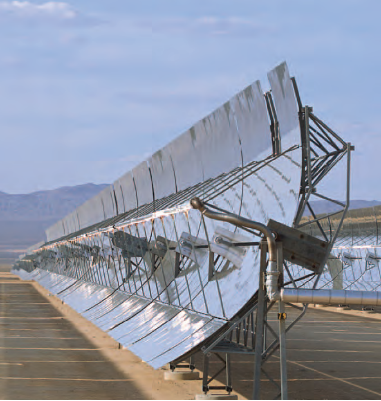
The parabolic-trough system concentrates heat through long curved mirrors tilted toward the sun.
