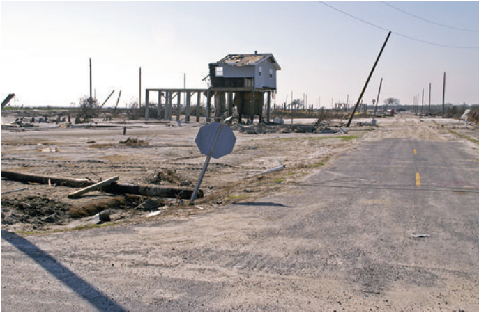
FIGURE 5-5. Johnson Bayou, Louisiana, November 16, 2005. This community at Johnson Bayou was almost totally leveled by the tidal surge and high winds of Hurricane Rita. Hurricane Rita left many people homeless and as of December 20, 2005 FEMA has taken 2,530,657 registrations from Hurricanes Rita and Katrina. Photo by Marvin Nauman/FEMA.
