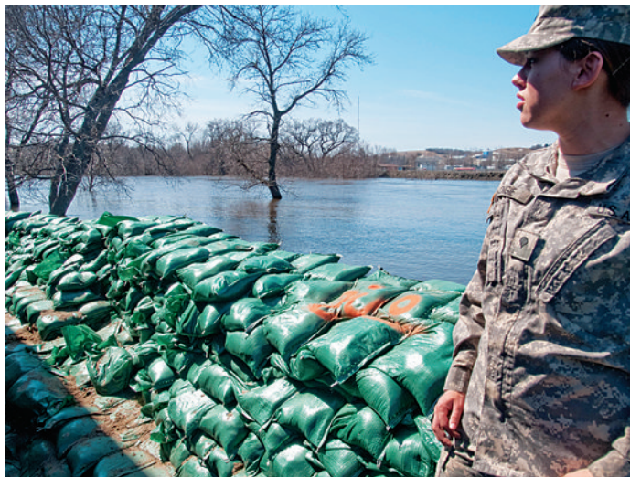
FIGURE 5-6. Valley City, North Dakota, April 14, 2009. North Dakota National Guard, Shayla Longie helps to protect homes along the Sheyenne River by running a 125 gal/min pump behind a dike made of sand bags. The river crested at a historic level of 22 feet. The old record was 19 feet. Photo by Michael Rieger/FEMA.
