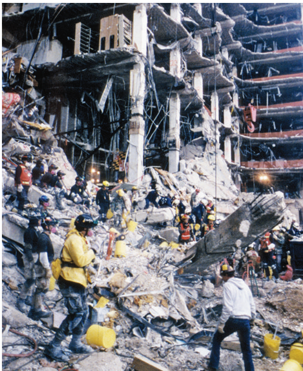
FIGURE 10-2. Oklahoma City, Oklahoma, April 26, 1995. High-powered explosives can cause devastating damage. Here search and rescue crews work to save those trapped beneath the debris, following the Oklahoma City bombing. FEMA News Photo.
