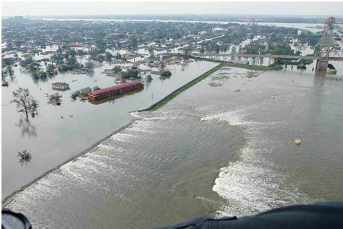
FIGURE 5-2. New Orleans, Louisiana, August 30, 2005. Aerial photograph of the break in the levee in the 9th ward. Neighborhoods throughout the area remain flooded as a result of Hurricane Katrina. Photo courtesy of Jocelyn Augustino/FEMA.
