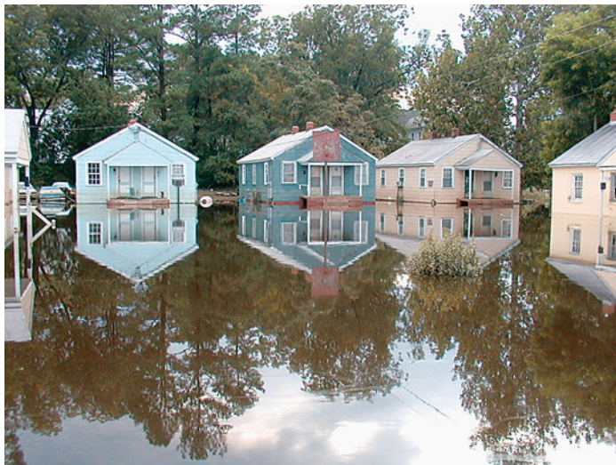
FIGURE 5–7. Franklin, Virginia, September 21, 1999. Flooding left the downtown section of Franklin under 6 feet of water after Hurricane Floyd. As the water has begun to recede, as shown by the high-water marks, hazards remained including propane tanks, gas tanks, chemical barrels, and pesticides. Photo by Liz Roll/FEMA.
