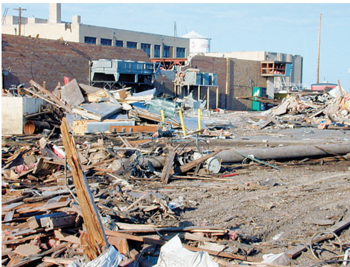
FIGURE 3-1. Hoisington, Kansas, April 26, 2001. The Hoisington tornado damaged the high school, a small shopping center, the hospital, and hundreds of homes in a matter of minutes. Hospitals are susceptible to storms, earthquake, and other manmade and natural disasters. A well thought out plan is essential, but even these may fail. Photo By Dave Saville/FEMA News Photo.
