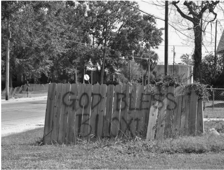
Figure 7.2 A damaged wooden fence containing the message “GOD BLESS BILOXI” (Mississippi). This picture was taken in 2006, or one year after 2005’s Hurricane Katrina event where the beginning phases of long-term recovery were just starting in Biloxi. (Photo by Brian Tomaszewski.)
