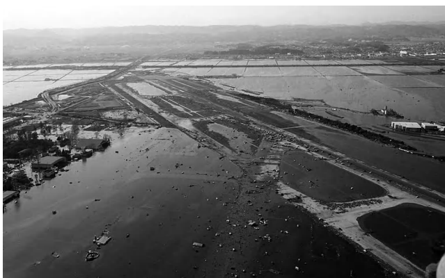
Figure 11.3 Impact at the Sendai Airport in Japan from the 2011 earthquake and tsunami. (From U.S. Air Force, Samuel Morse.)
