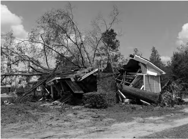
Figure 13.1 Damage from April 16, 2011, North Carolina F3 tornado. (From FEMA, David Fine.)
