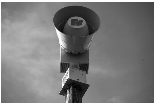
Figure 8.2 Outdoor warning sirens have long been a traditional public notification strategy. (From FEMA, Leif Skoogfors.)
