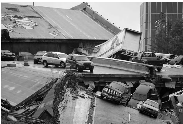
Figure 10.5 Cars rest on the collapsed portion of I-35W Mississippi River bridge in Minneapolis, after the August 2007 collapse. (From U.S. Coast Guard, Kevin Rofidal.)
