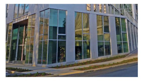
The window selection for the Net Zero Energy Bullitt Center in Seattle involved finding a highperformance window with automatic operability. The German window manufacturer Schuco provided a window design that minimized thermal bridging through the aluminum frame and opens 3" to 4" parallel to the building façade, reducing differential wear on the gaskets and airflow through the frame. Tvis = .60 and U = .25 overall, including operable lites. Source: Photograph © Kjell Anderson.
