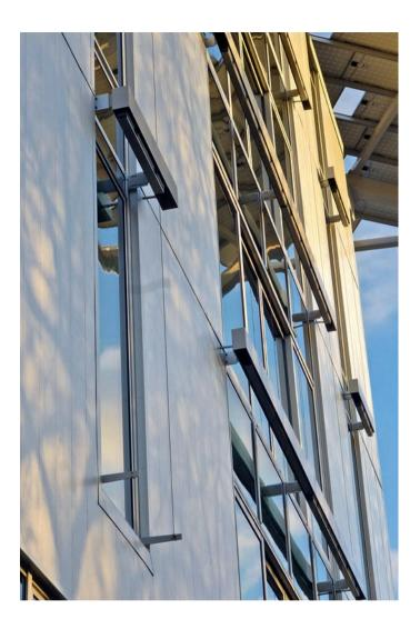
Automated external operable shades on guide wires control heat gain and glare much more effectively than internal blinds. Source: Photograph © Kjell Anderson.
