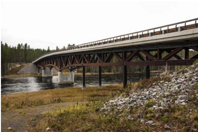
Figure 12.19 A 158-m-long bridge across Rena River, Norway.
