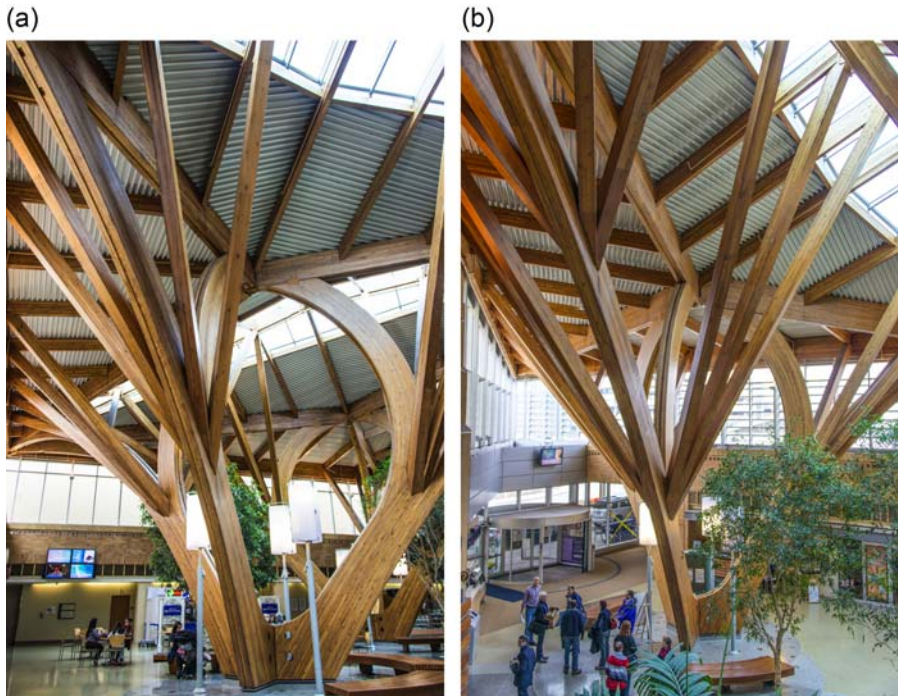
Figure 12.16 (a) and (b) Glulam primary structure in the hospital foyer.
