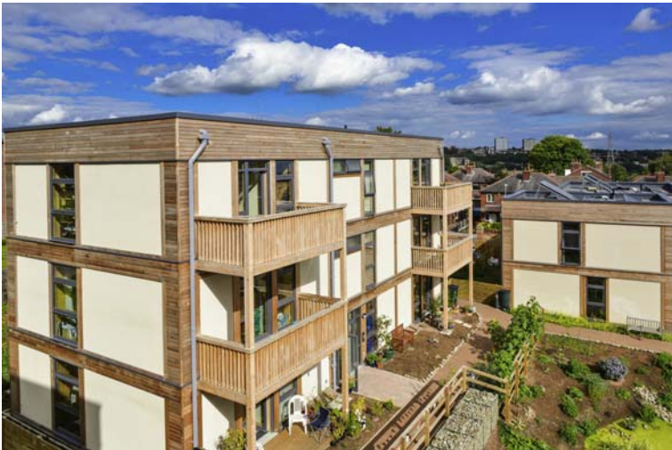
Figure 6.19 Load-bearing straw bale panels at the LILAC project, Leeds, UK, 2013. Courtesy of ModCell.
