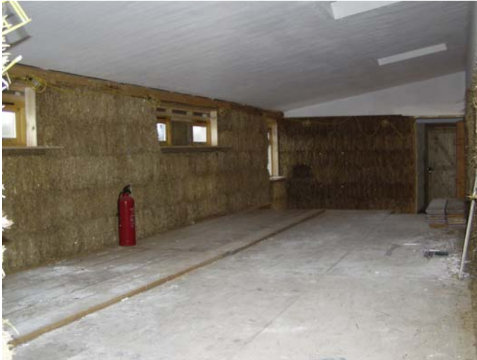
Figure 6.3 Load-bearing straw bale wall under construction.
