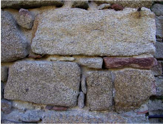
Figure 11.1 Granite ashlars in a building of Giglio island (Tuscany, Italy). Photograph: F. Fratini.
