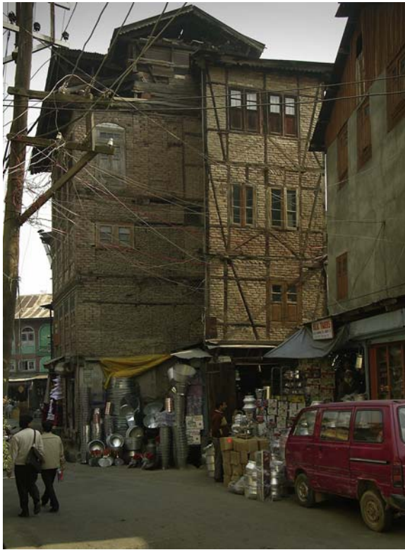
Figure 1.14 View of four- and five-story buildings of traditional taq (on the left) and Dhajji dewari (on the right) construction in the city center of Srinagar, Kashmir, 2005.
