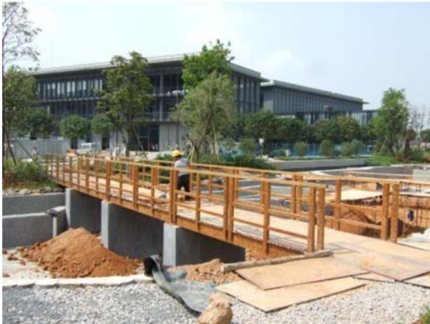
Figure 15.13 The Wanke 20-m-long bridge near completion.
