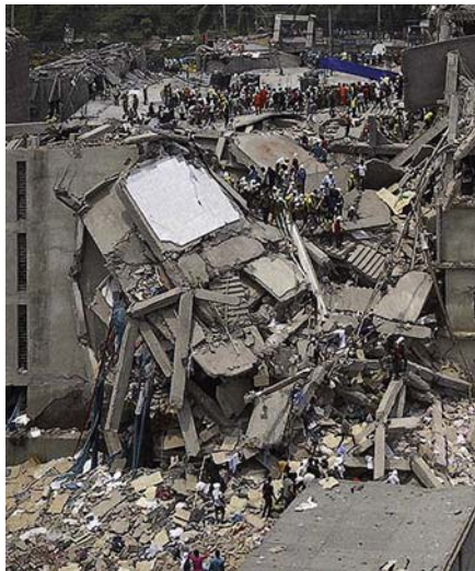
Figure 1.11 Rana Plaza after 2013 pancake collapse that killed 1,129 people. Photo by Rijans, Wikimedia CC.
