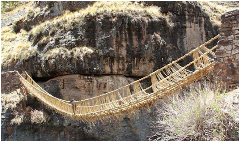
Figure 2.5 Inca suspension bridge in Huinchiri, Peru.
