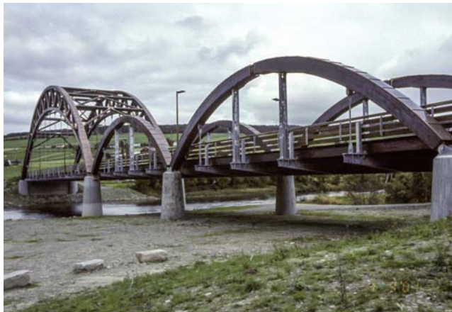
Figure 12.17 Side view Tynset Bridge.
