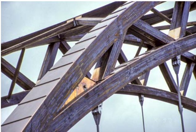
Figure 12.18 Connection and flashing details – Tynset Bridge.
