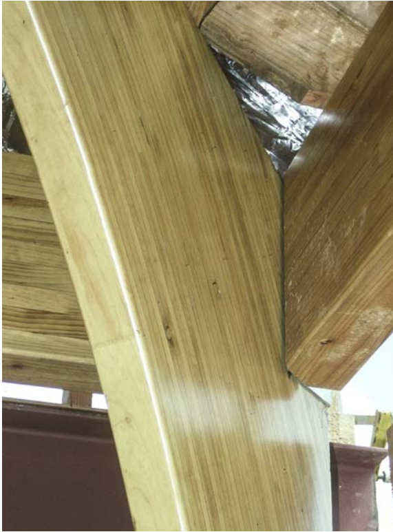
Figure 12.14 Curved glulam beam.
