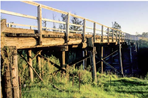
Figure 12.5 An 80-m-long multispan timber girder bridge in Australia.
