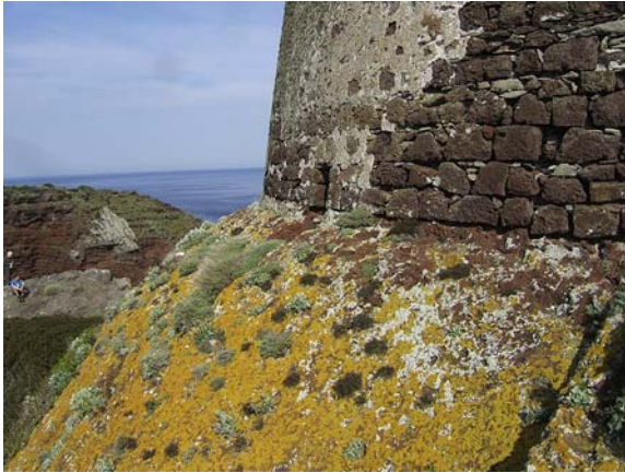
Figure 11.2 The Zenòbito Tower (XVIth century) in the Capraia Island (Tuscany, Italy), built in trachyte blocks.
