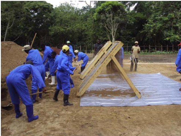
Figure 8.10 Sieving process of soil.
