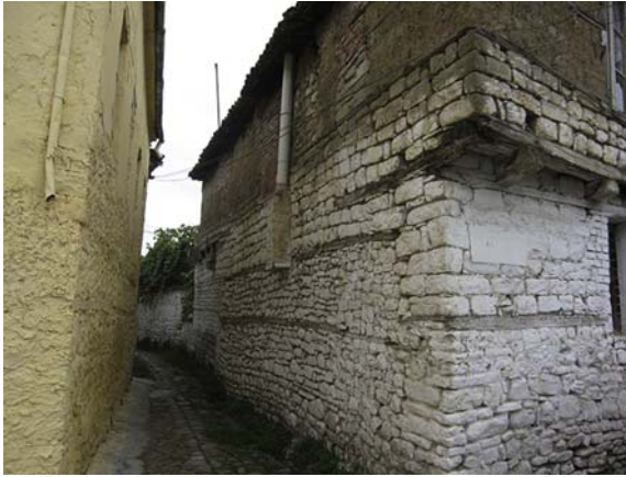
Figure 11.18 Masonry with hooping wood reinforcement in Elbasan (Albania). Photograph: L. Rovero.
