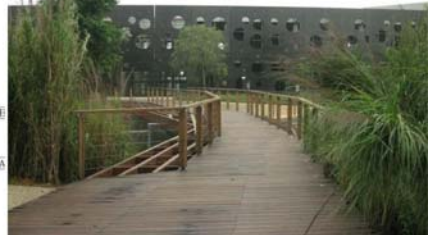
Figure 15.14 The Wanke 40-m-long bridge: (a) plan layout of glulam girders and (b) completed bridge.
