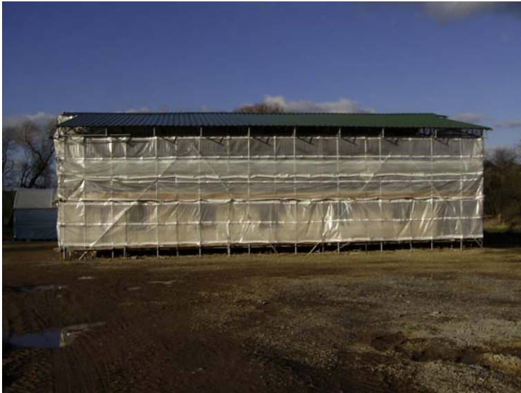
Figure 6.15 Temporary shelter for straw bale construction.
