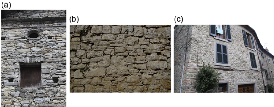
Figure 11.13 (a) Random rubble masonry with a little amount of bedding mortar in Lunigiana (Tuscany, Italy). (Photograph: L. Dipasquale.) (b) Random rubble masonry in Alberobello (Apulia, Italy). (Photograph: L. Dipasquale.) (c) Random rubble masonry with a lot of bedding mortar in Cortona (Tuscany, Italy). (Photograph: L. Rovero.)
