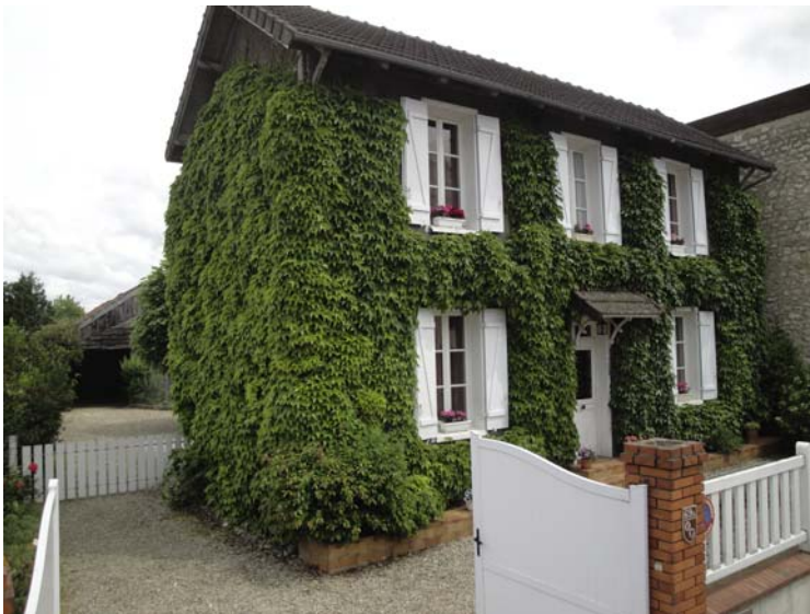
Figure 6.2 Feuillette house, Montargis, France (built 1921). Photo courtesy of RFCP.
