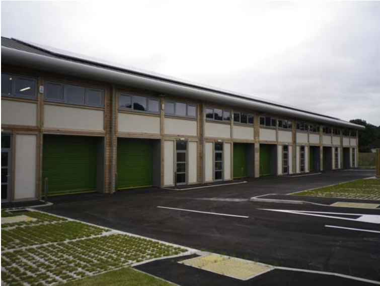
Figure 6.18 Straw bale cladding panels at the Inspire Bradford project, Bradford, UK, 2012.
