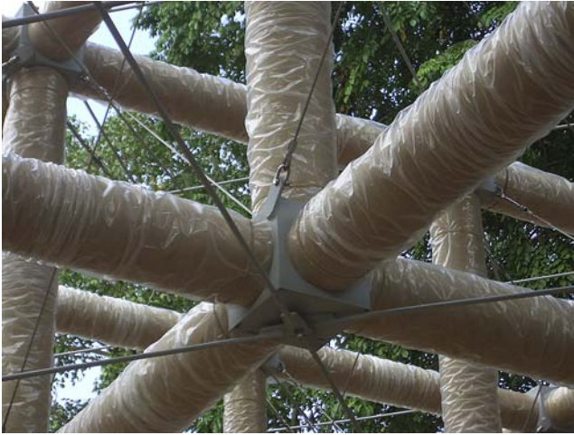
Figure 16.18 Details of space truss from the Singapore Biennial Pavilion, 2006. With permission from Eddie Chng, Sonoco Products Company.
