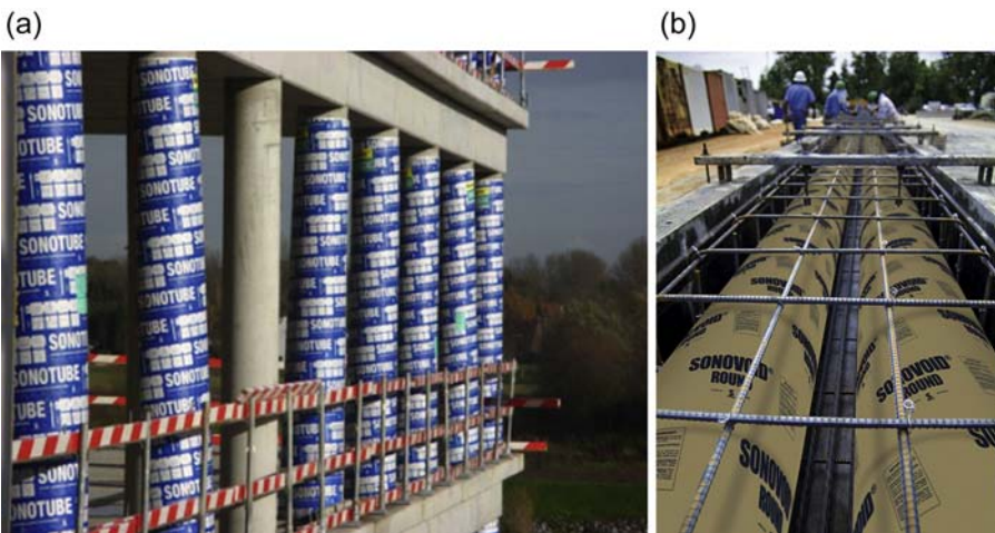
Figure 16.2 (a) Column forms and (b) voided slab tubes. Photographs with permission from Sonoco Products Company.
