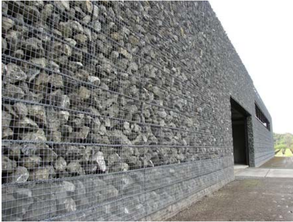
Figure 11.23 Dominus Winery by Herzog & de Meuron realized with gabions.
