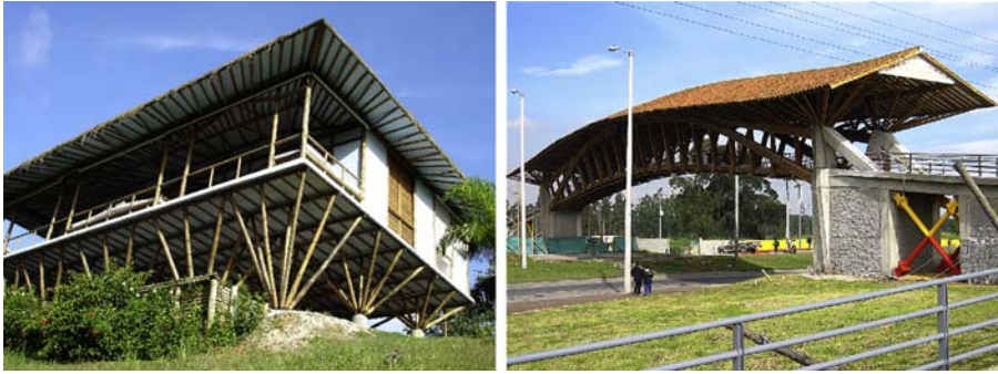
Figure 14.2 Common structures constructed with bamboo. Courtesy of Simón Vélez.
