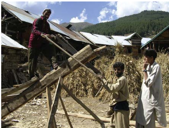
Figure 1.15 Contemporary continuation of preindustrial technique of sawing timbers into boards in Kashmir.
