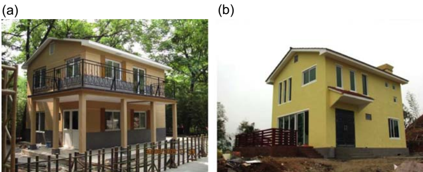
Figure 15.8 Completed glubam stud-wall houses: (a) 100-m 2 tea house built in Black Bamboo Park in Beijing in August 2009 and (b) 120-m 2 mountain house in Cailun Forest, Leiyang, Hunan Province, completed in November 2009.
