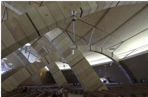
Figure 11.21 Liturgical Hall “Padre Pio” of Renzo Piano in San Giovanni Rotondo (Apulia, Italy). Photograph: F. Fratini.
