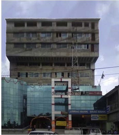
Figure 1.10 Front façade of the Rana Plaza , Bangladesh before collapse. Elevation view of front façade of Rana Plaza near Dhaka, Bangladesh. This rectified image was constructed by author from a combination of news media TV video images to show the façade prior to collapse. This photo reconstruction of the building serves to bring into focus a fact that, in addition to its structural failings, it was unremittingly ugly as a work of architecture. I would say that these two aspects of building design are actually closely related — the developer Sohel Rana’s grotesque failure even to grasp the truth of his own engineers’ warnings of imminent collapse are of a piece with his ignorance and even contempt for architectural expression that is in any way responsive to the local and national culture (see TEDxAmoskeagMillyard talk [11]).
