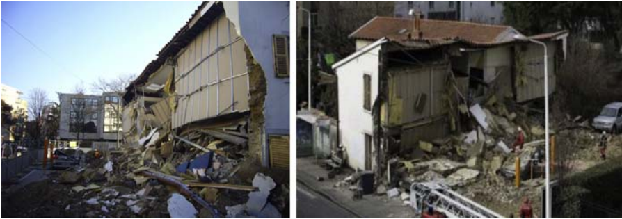
Figure 10.11 Picture of the collapse of a rammed earth construction in the city of Lyon (France), left: basement after removing the collapse rammed earth, right: the rammed earth wall after its collapse.
