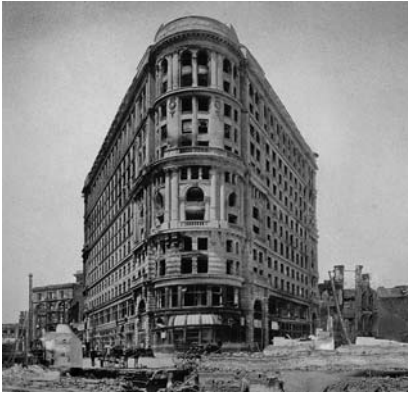
Figure 1.20 View of the 1904 steel skeleton frame with infill masonry Flood building after the 1906 San Francisco earthquake and fire.
