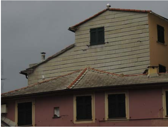
Figure 11.8 The Ligurian slate (ardesia) used as tiles for roofs and wall protection (Genoa, Italy).
