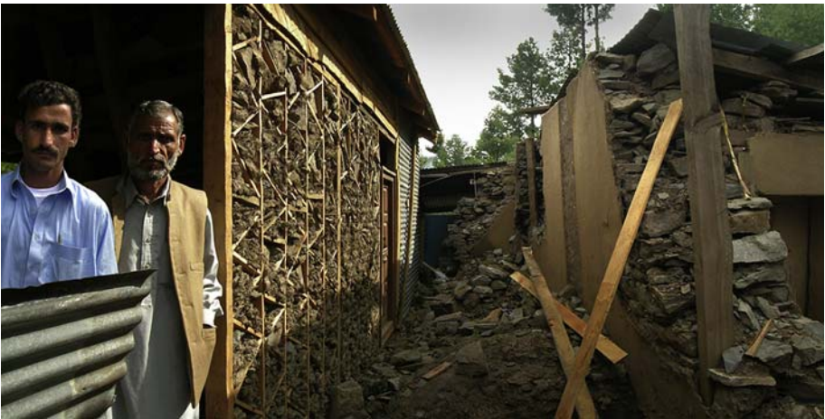
Figure 1.31 The owner and carpenter of a new house under construction in rural Pakistan near to the building shown in Fig. 1.29 after the earthquake destroyed the owner's original rubble stone home, the ruins of which are on the right. The decision to reconstruct in dhajji construction was because the one home in the village that did not collapse was of that construction and the reinforced concrete village store collapsed.
