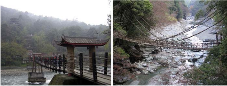
Figure 2.6 Ancient suspension bridges made from plant-fibre ropes: Anlan Bridge, Chengdu, China (Photo credit: Prince Roy ) and Iya Valley Bridge, Kazurabashi, Japan (Photo credit: Osaki ).
