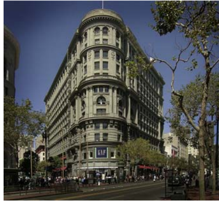
Figure 1.21 The same view shown in Fig. 1.20 but 100 years later. Most of the steel skeleton-frame buildings were repaired after the earthquake despite the fact that all were burnt out by the fire.
