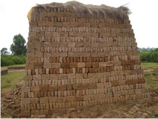
Figure 9.9 Protection of cement-stabilized (unfired) clay bricks at a community brick project (cooperative) in Kenya (note grass cover on pile, to reduce the effect of rain).
