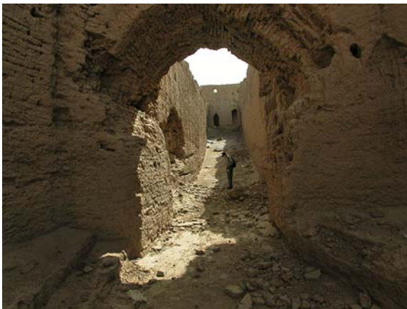
Figure 1.3 View of an archeological site in Bam with high walls that came through the 2003 earthquake with very little damage.
