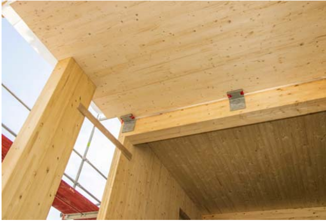
Figure 12.24 CLT construction in Austria similar to that used in the Forté building.
