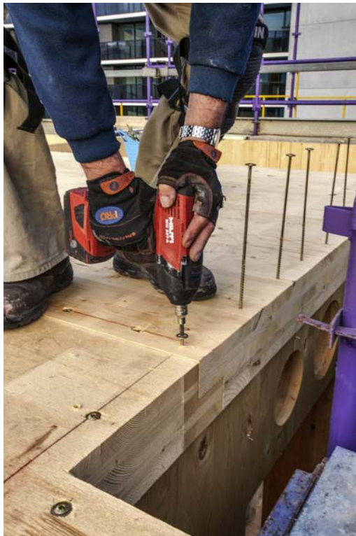
Figure 12.23 Connecting panels – Forté building (Emma Cross photographer).
