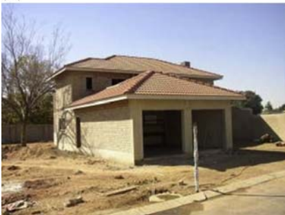
Figure 8.19 Examples of Hydraform dry-stack interlocking CSEB system. (a) Double-story building in Johannesburg using CSEB interlocking system. (b) House construction with confinement of the dry-stack masonry units.
