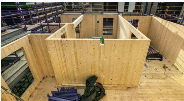
Figure 12.22 Prefabricated panels — Forté building (Emma Cross photographer).
