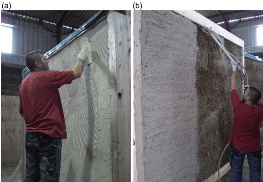
Figure 6.14 Rendering of straw bale wall. (a) Manual finishing off of lime render. (b) Lime render sprayed directly onto surface of the straw bales.
