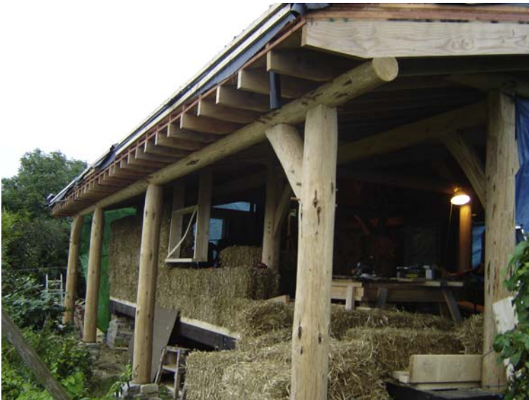
Figure 6.16 Non-load-bearing straw bale building under construction.
