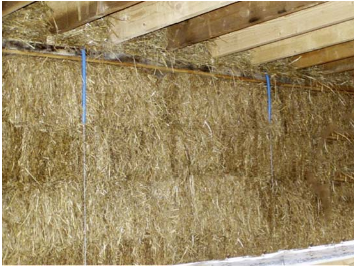
Figure 6.1 Load-bearing straw bale wall.
