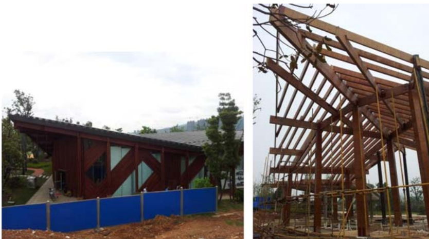
Figure 15.10 Glulam heavy frame building.
