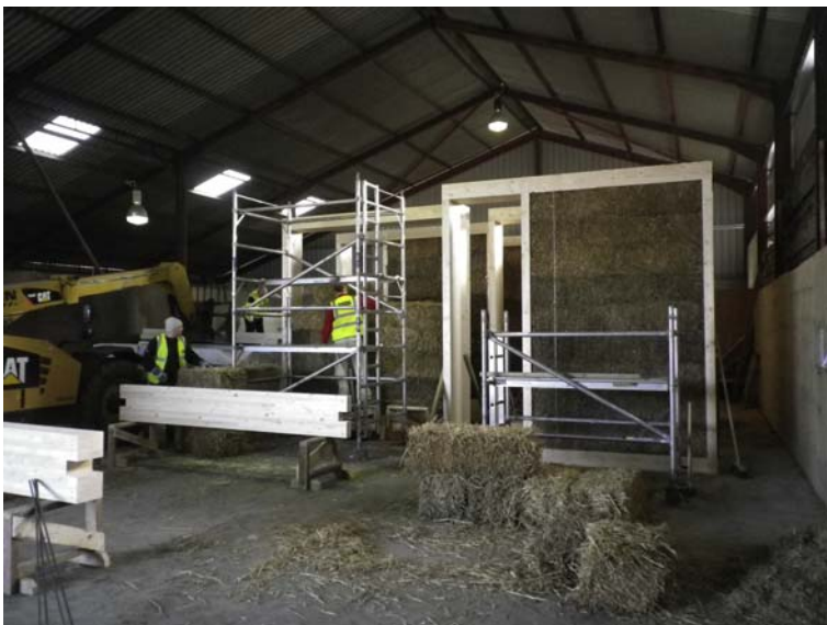
Figure 6.17 Fabrication of prefabricated straw bale panels.
