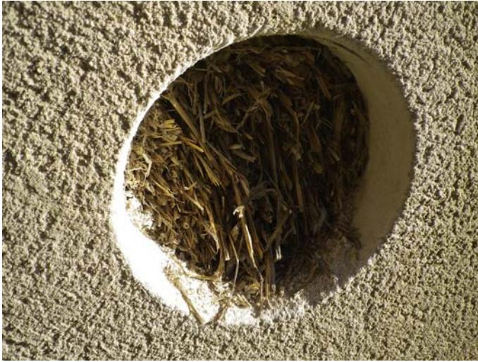
Figure 6.10 External render core removed from straw bale wall panel.
