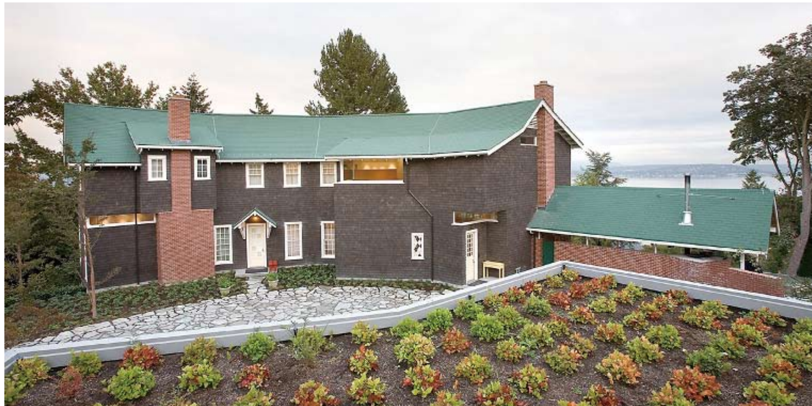
Above: Final landscape site plan Below: Auto-court with recycled concrete paving Facing: Edible garden with iconic apple tree
