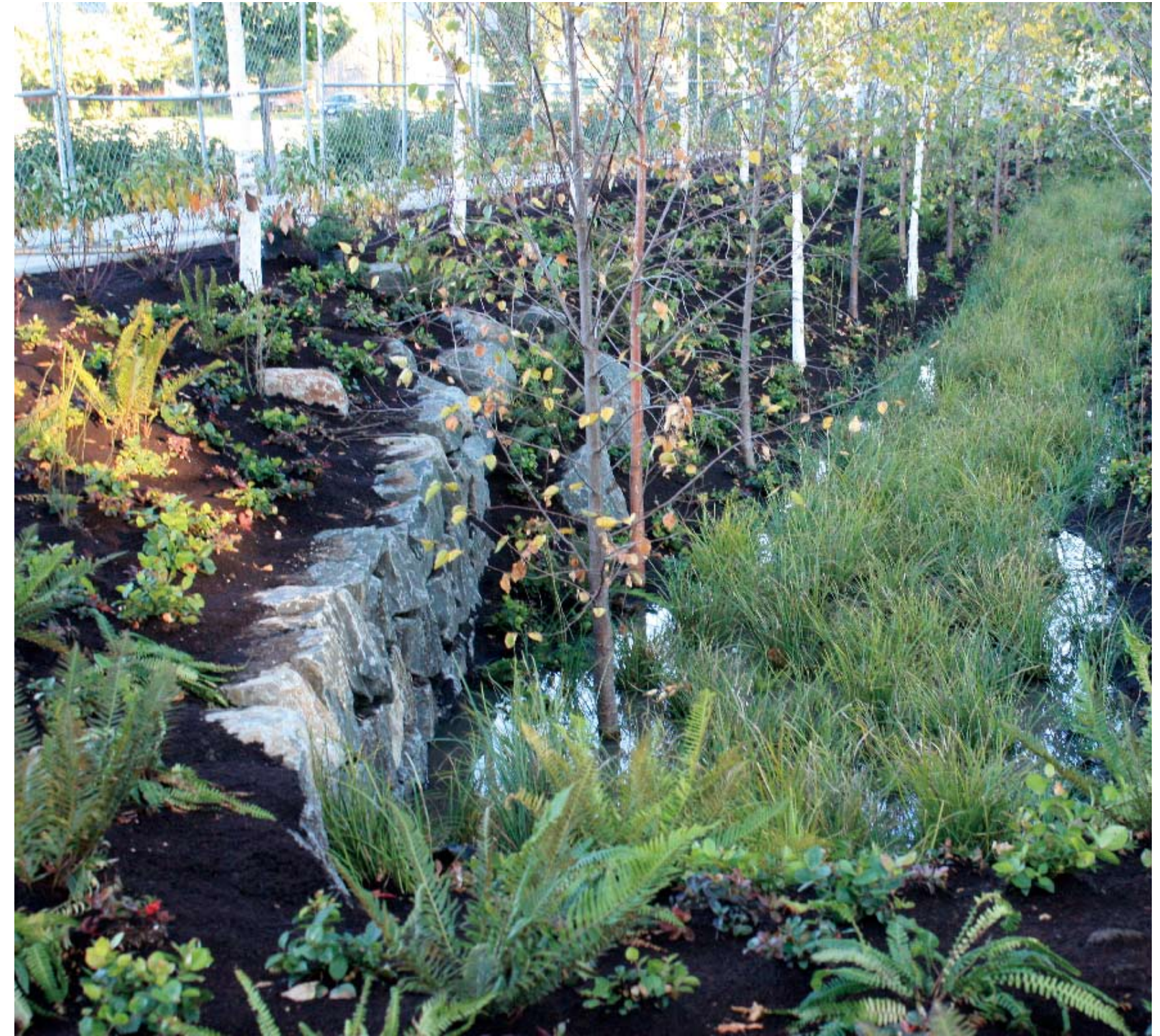
Above: The bioswale in the Birch Forest is planted with grasses, shrubs, and trees that adapt well to inundation. The city commented that this is the best looking, and functioning, bioswale that they have ever seen
