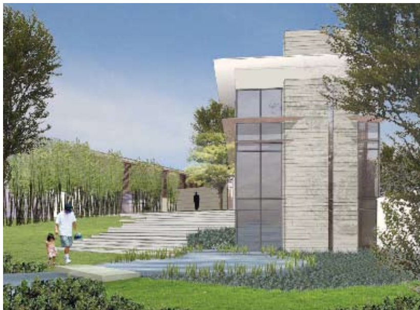
Above: Site plan Below: Backyard of villa E18 Facing: The courtyard at villa W33 is composed of floating planes of water, grass, and paving
