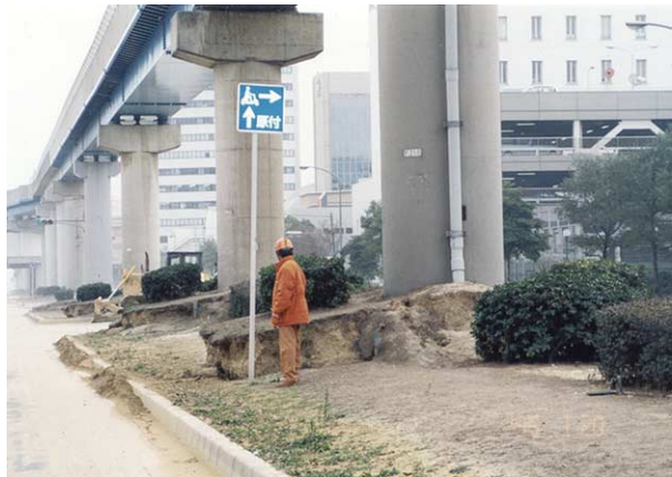
Figure 12 An elevated transport link in Kobe following the 17 January 1995 earthquake. The bridge piers were piled, and the structure is generally undamaged despite the settlement of the surrounding soil by up to 1 m.
