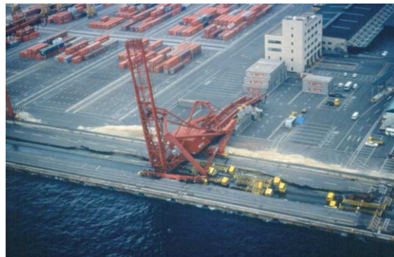
Figure 1 Liquefaction of reclaimed fills at the Port of Kobe in 1995 caused complete suspension of operations. The lateral displacement of the quay walls in this picture pulled apart the crane legs, causing collapse. Photograph by Leslie F. Harder, Jr.
