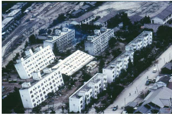
Figure 11 Tilted buildings with shallow foundations in Niigata, Japan (1964) as a result of liquefaction-induced bearing-capacity failure.
