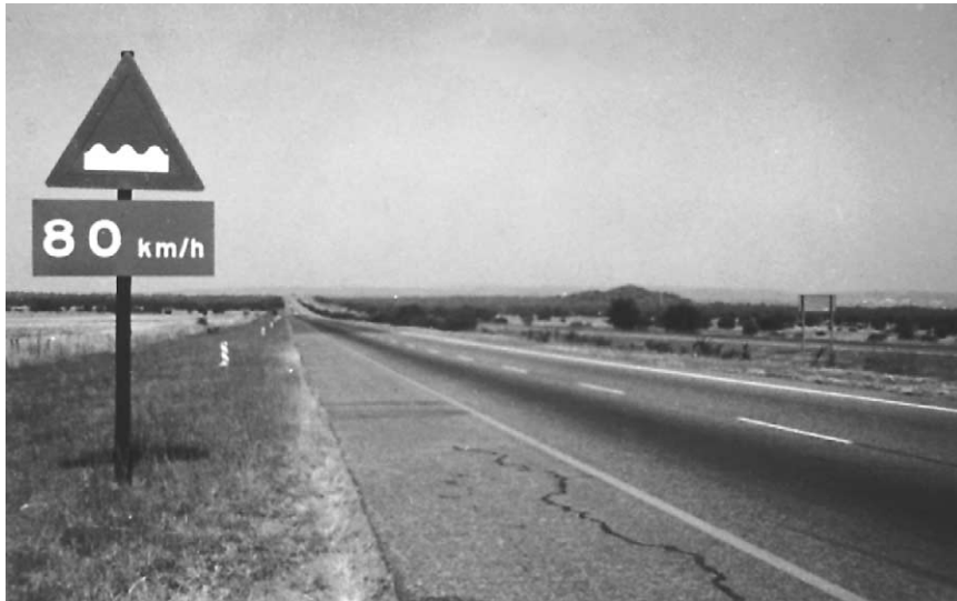
Figure 4 Breakup along the CapeTown Johannesburg road, South Africa, due to expansive clay.
