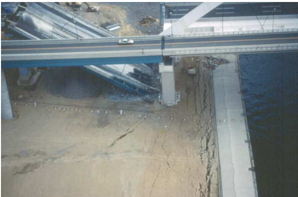
Figure 15 This span of the Nishinomaya Bridge collapsed following the 1999 magnitude 6.9 Kobe earthquake in Japan as a result of liquefaction-related foundation deformations. Ground cracks behind the quay walls and parallel to the water edge are indicative of the lateral ground movements that occurred. Sand boils are visible on the ground surface. Photograph by Leslie F. Harder, Jr.
