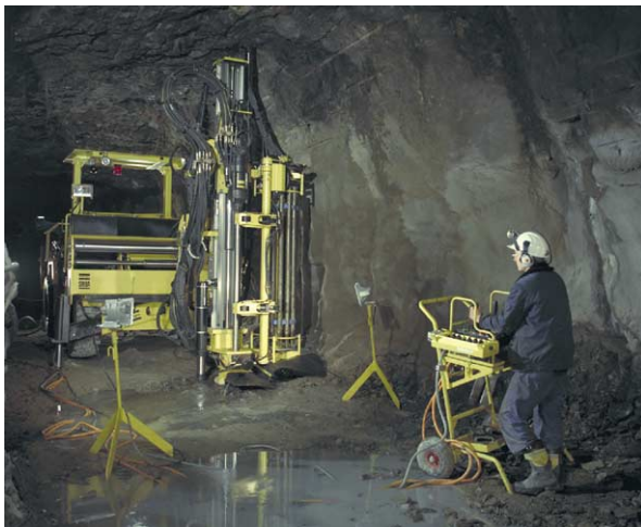
Figure 3 Underground exploration drilling (Simba H1354 for Echo Bay, Canada). Photograph by Atlas Copco.
