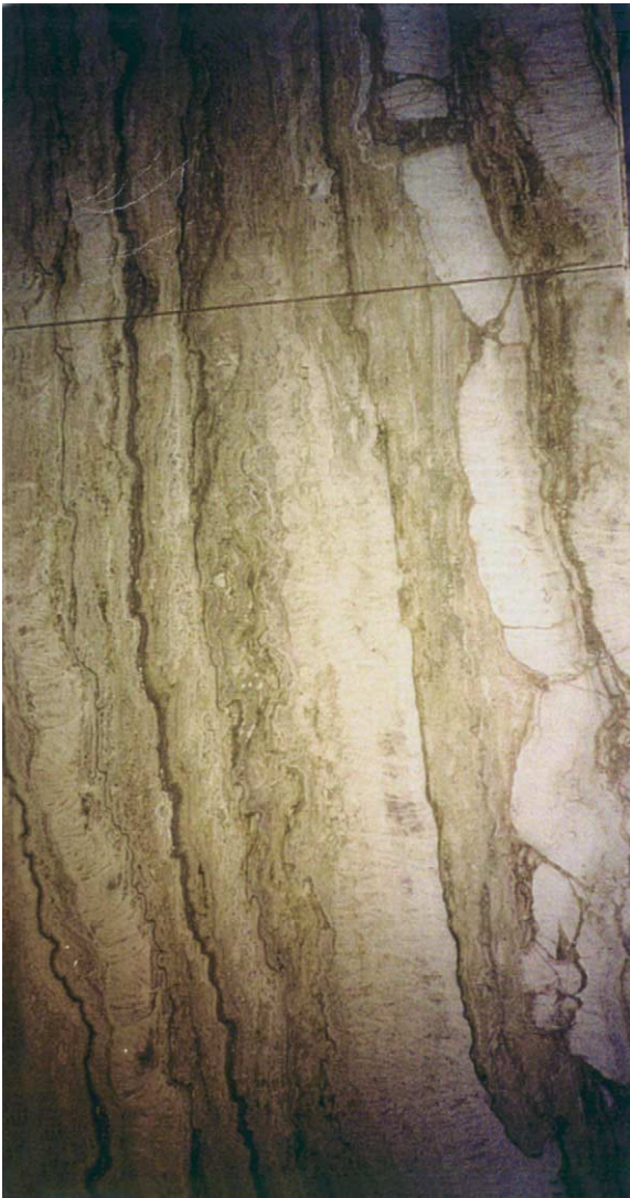
Figure 14 Travertine cladding on a McDonald's Restaurant, Hereford, England. Photograph by GJH McCall.
