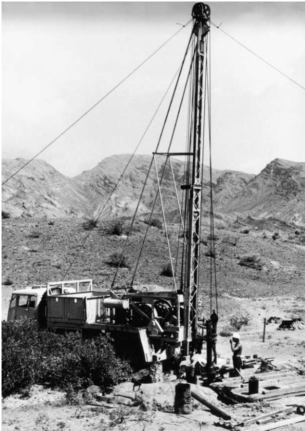
Figure 7 Royal Engineers boring for water in the South Arabian Federation in 1964. Military geologists from the British reserve army were used to guide such deployments during a time of intermittent conflict. © Crown Copyright/MOD. Reproduced with the permission of the Controller of Her Majesty's Stationery Office, and courtesy of the Royal Engineers Library, Chatham.
