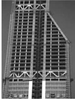
Figure 11.3 Multiple antennas in a large building.
