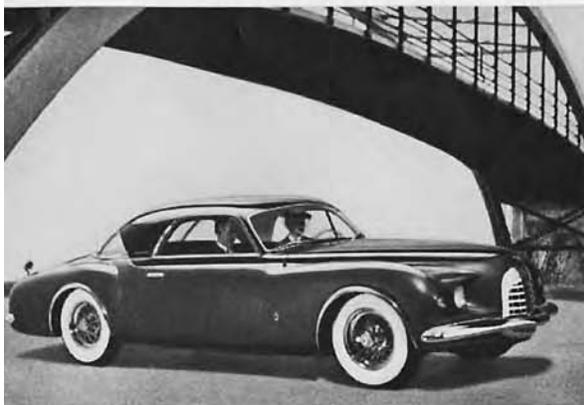
**THE K-310**, designed and engineered by Chrysler and handcrafted by Ghia of Turin, Italy. Only 59" high, with a wheelbase of 125½", it is designed to use the Chrysler FirePower V8 Engine and full-time Power Steering. This "idea car" represents an entirely new American theme in motor car functional styling.
