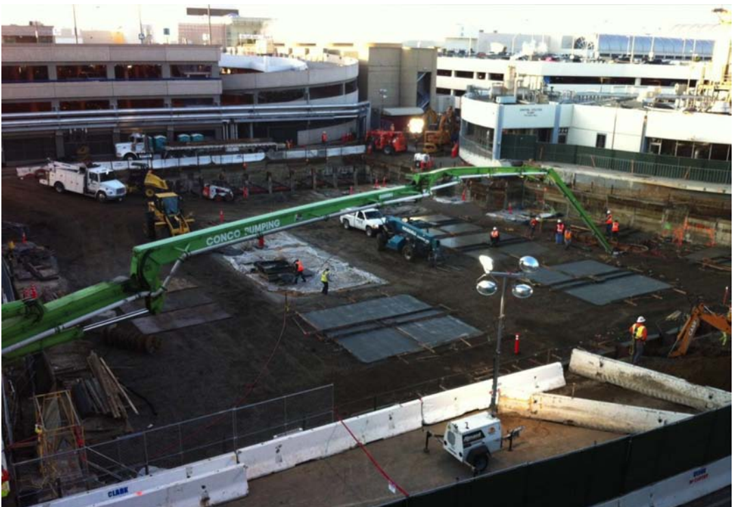
Figure 5-5. Replacement Central Utility Plant Construction
