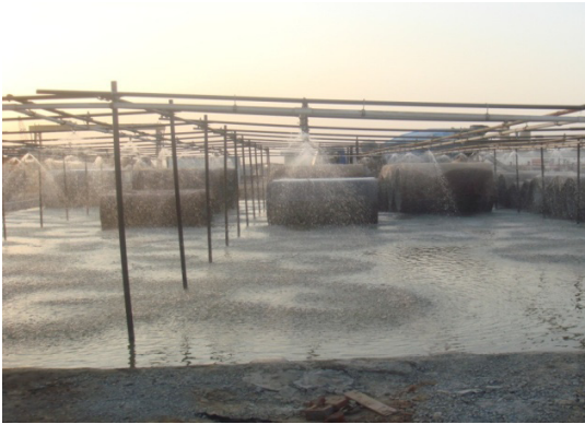
Figure 1-16. Curing of pipes by sprinklers
