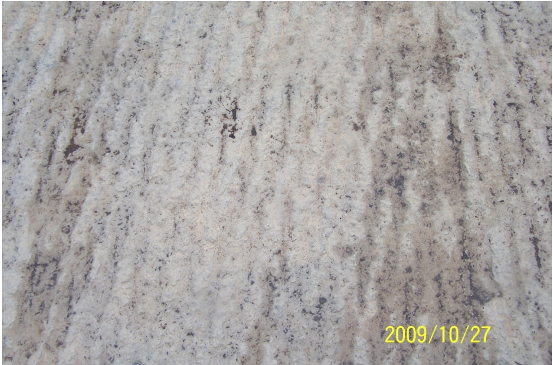
Figure 4-2. Whitewashed Milled Surface
