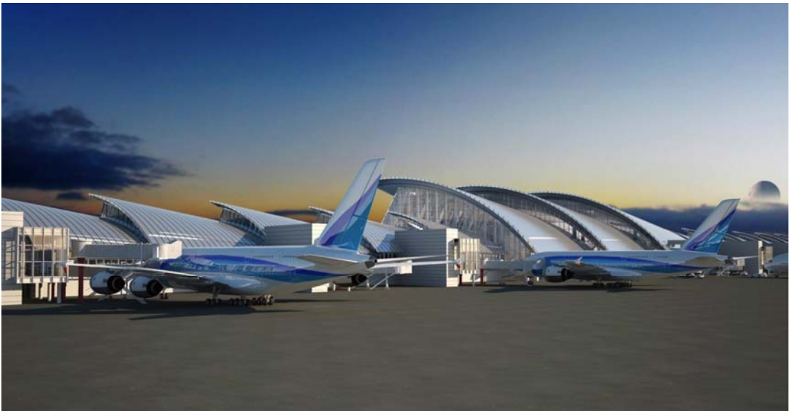
Figure 5-3. Exterior Rendering of the completed Tom Bradley International Terminal West Improvements
