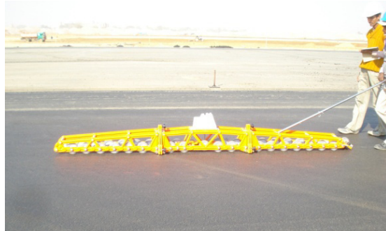
Figure 1-12. Rolling straight edge check
