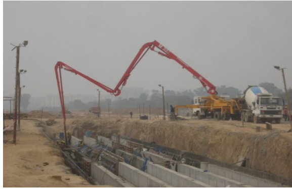
Figure 1-15. Boom placer
