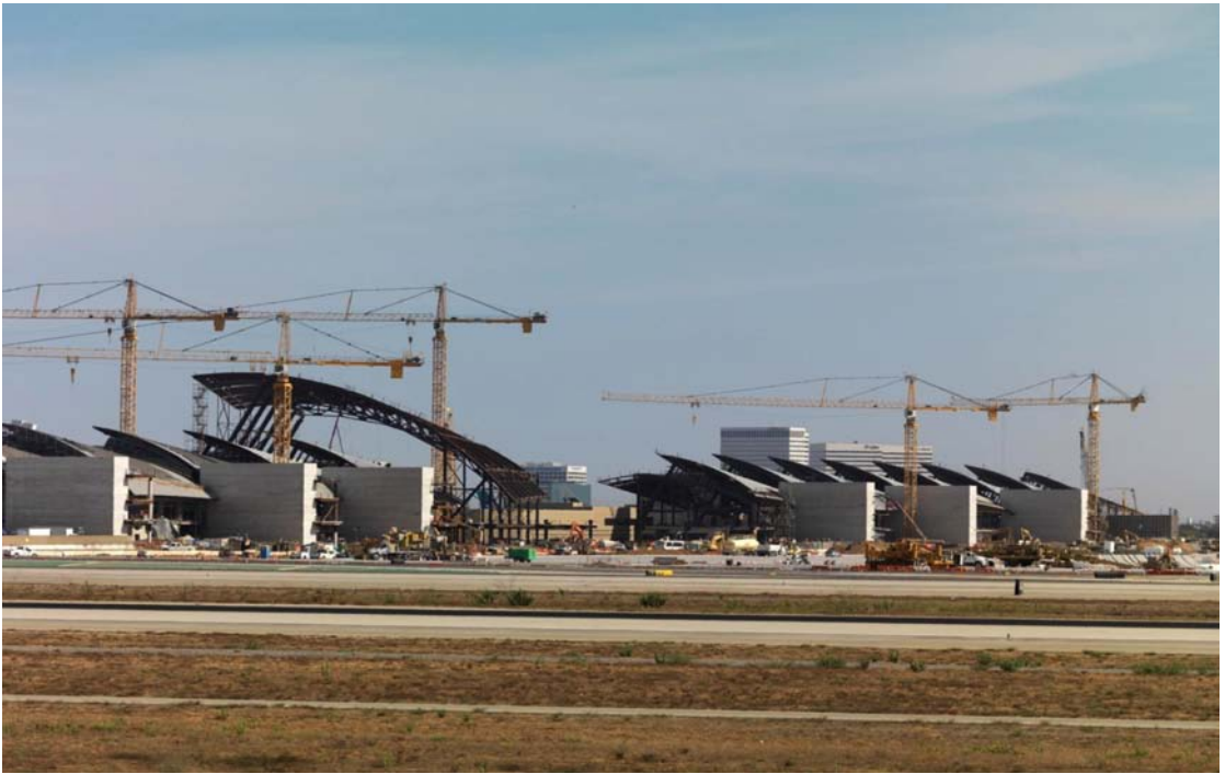
Figure 5-2. Construction of the Tom Bradley International Terminal West
