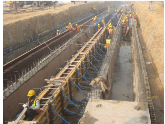
Figure 1-17. Box culvert construction
