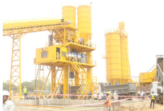
Figure 1-9. Batching plant Source: Delhi International Airport Limited (DIAL); reproduced with permission
