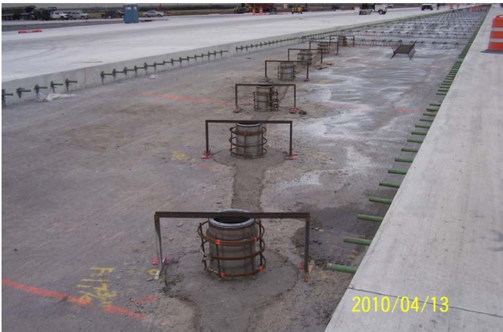
Figure 4-3. Reinforcing Cage around Light Can with Alignment Jig In-place
