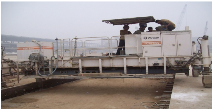
Figure 1-13. Wirtgen slip form paver
