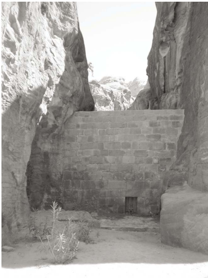
Fig. 3: As the dams were thought to detain rather than to retain water, they had an outlet at the bottom. The orifices were 10 to 14cm in diameter and pierced through the sandstone blocks or made of ceramic pipes.
