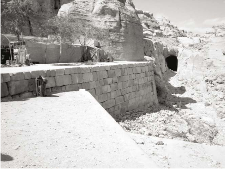
Fig. 4: After having been diverted by a 8m high dam, the stream of a flood was directed to the Wadi Mudhlim i.a. through this rock-cut tunnel (82m long, 4.8m wide, about 8m high).
