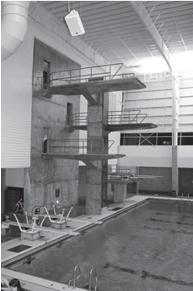
Figure 12-14. Diving facility. The diving well is separate from the pool and features a tower and springboards. The tower has cement platforms at 5-, 7-, and 10-meter heights above the water. The springboards are at 1- and 3-meter heights.
