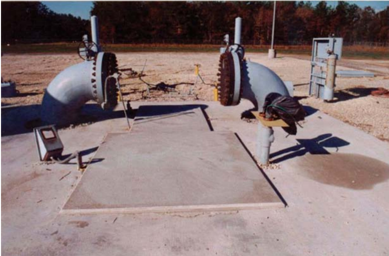
Figure 12.9 Grout cap is poured with the pump removed.
