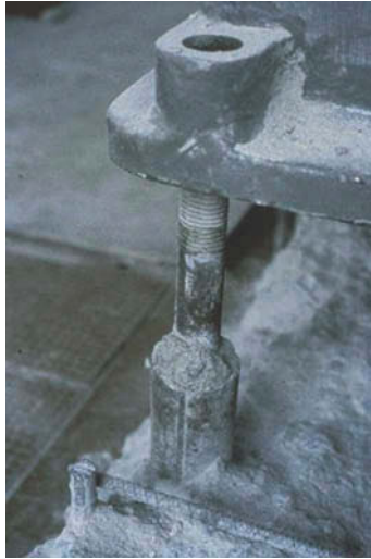
Figure 2.2 Bolt sleeve filled with grout.
