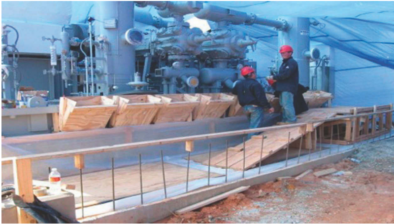
Figure 3.4 Environmental control is essential to successful grouting.
