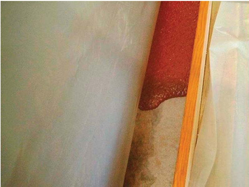
Figure 12.2 The ability of the grout to flow and sufficient clearance is necessary.
