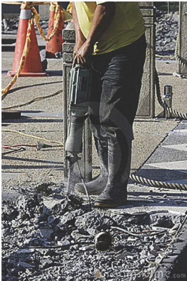
Figure 9.2 Jackhammers are not recommended for concrete surface preparation.
