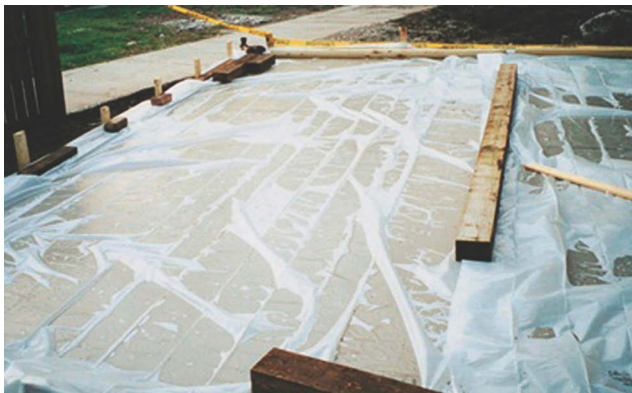
Figure 1.10 Polyethylene sheeting is applied to reduce rapid drying.
