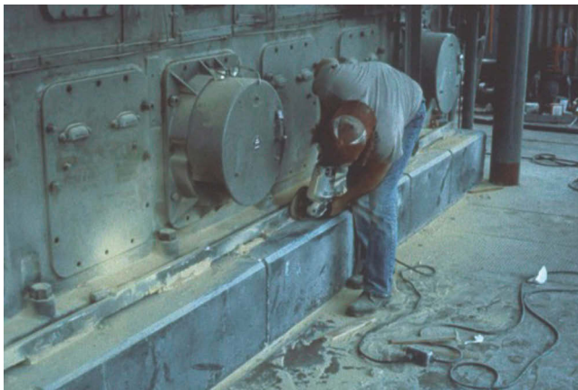
Figure 13.4 Grinding off the chock overpour.
