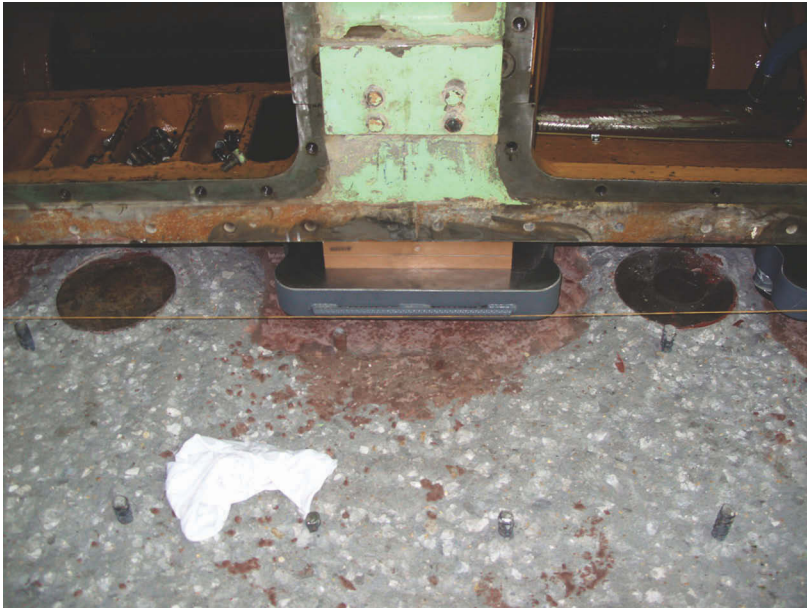
Figure 9.1 Aggregate shown is imbedded in the concrete.
