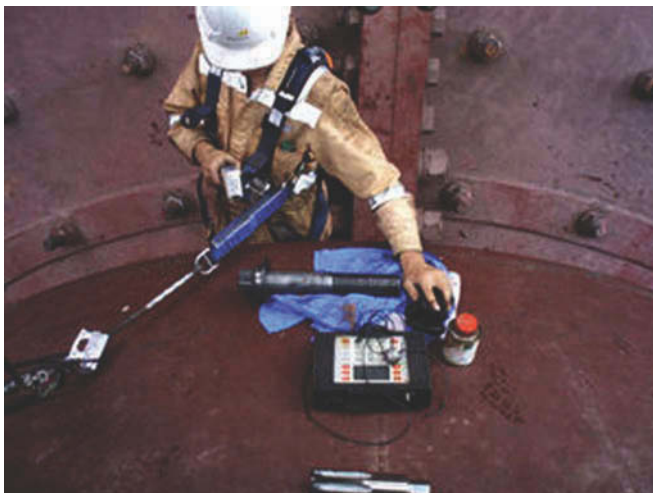
Figure 2.9 A technician gathers preinstallation relaxed bolt length.
