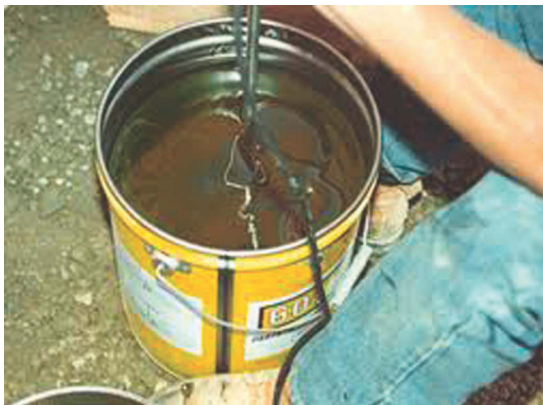
Figure 4.3 Avoid vortexing of the liquids to minimize air entrainment.
