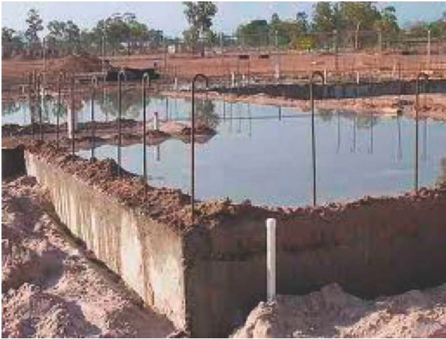
Figure 1.11 Water flood is another form of reducing the possibility of rapid drying but is labor intensive.
