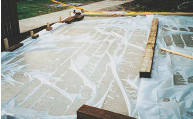
Figure 1.8 Foundation covered with polyethylene sheeting to retard rapid evaporation.
