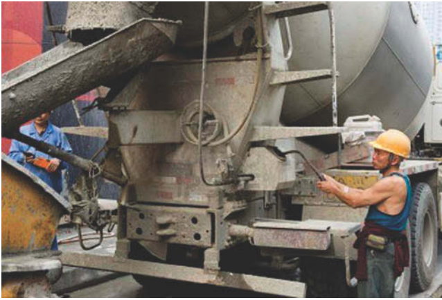
Figure 1.6 Do not allow water to be added randomly to the mix.
