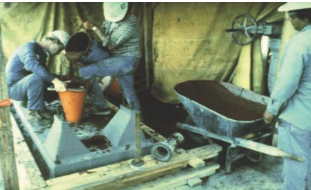
Figure 11.12 Utilizing a traffic cone as a head box for grout installation.
