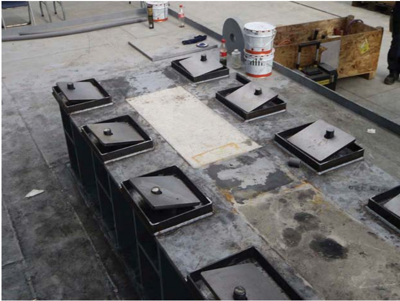
Figure 12.14 The soleplates are set in position and rough leveled.
