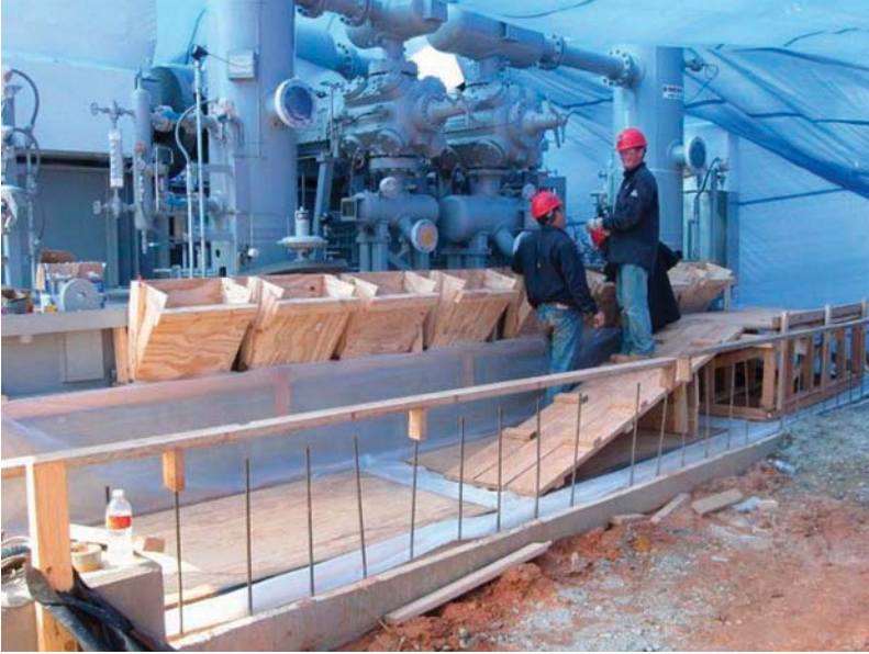
Figure 12.1 Head box can facilitate grout placement under large skid-mounted equipment.
