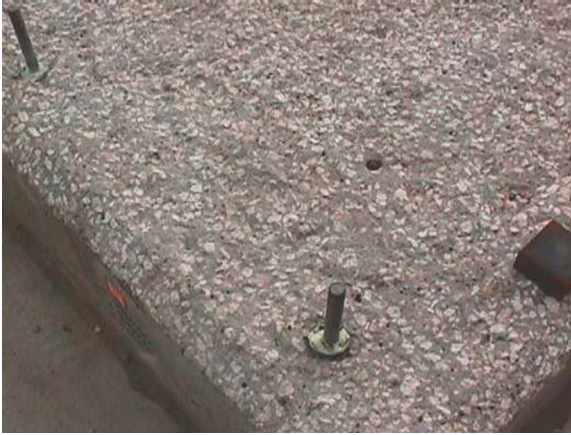
Figure 3.1 Properly chipped concrete.
