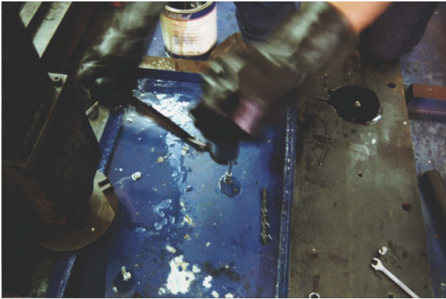
Figure 10.8 Injecting the epoxy liquids into the baseplate voids.
