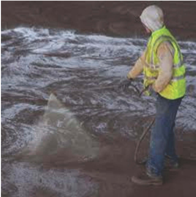
Figure 1.9 Spray-applied curing membrane.
