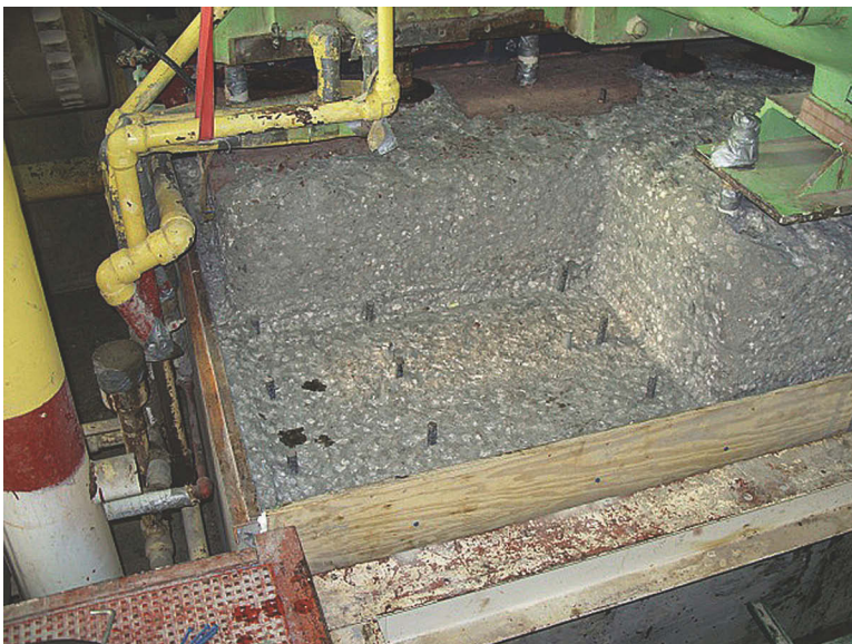
Figure 8.1 Concrete chipped and rebar installed to prevent edgelifting.
