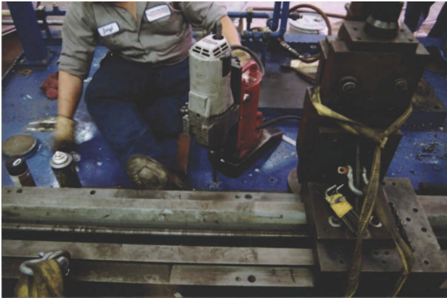
Figure 10.4 Drilling injection and vent holes into the baseplate.
