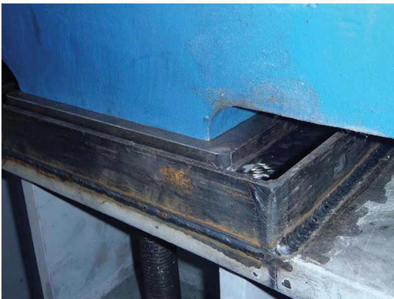
Figure 12.15 The compressor is set and aligned to the prime mover.
