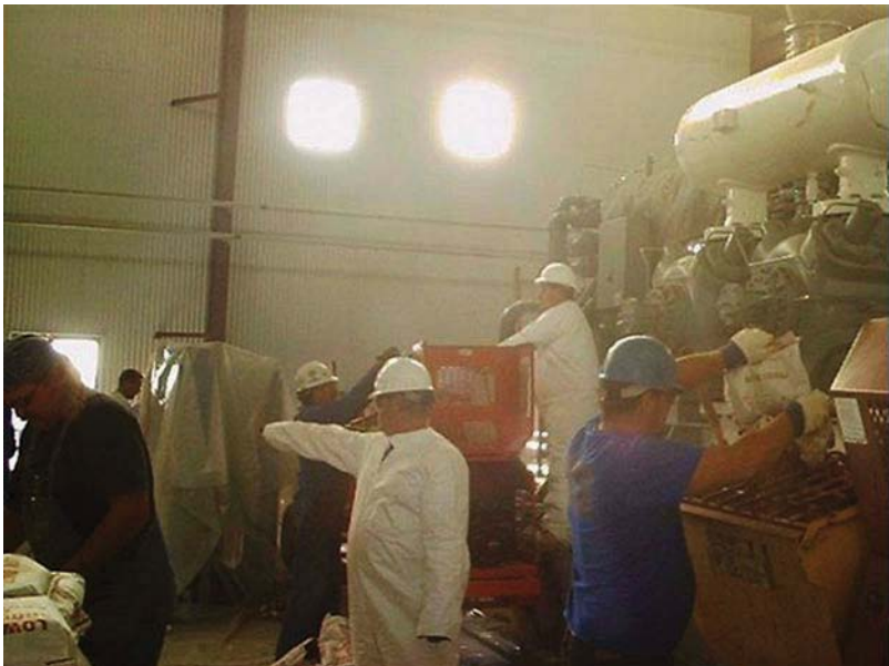
Figure 12.6 Mixing teams should work together during grout mixing and placement.
