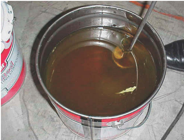
Figure 11.9 Follow proper mixing techniques to avoid whipping air into the liquids.
