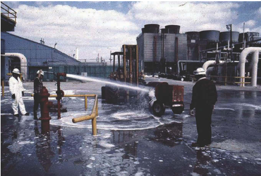
Figure 11.14 Cleaning uncured grout from the mixer is easily accomplished using water.
