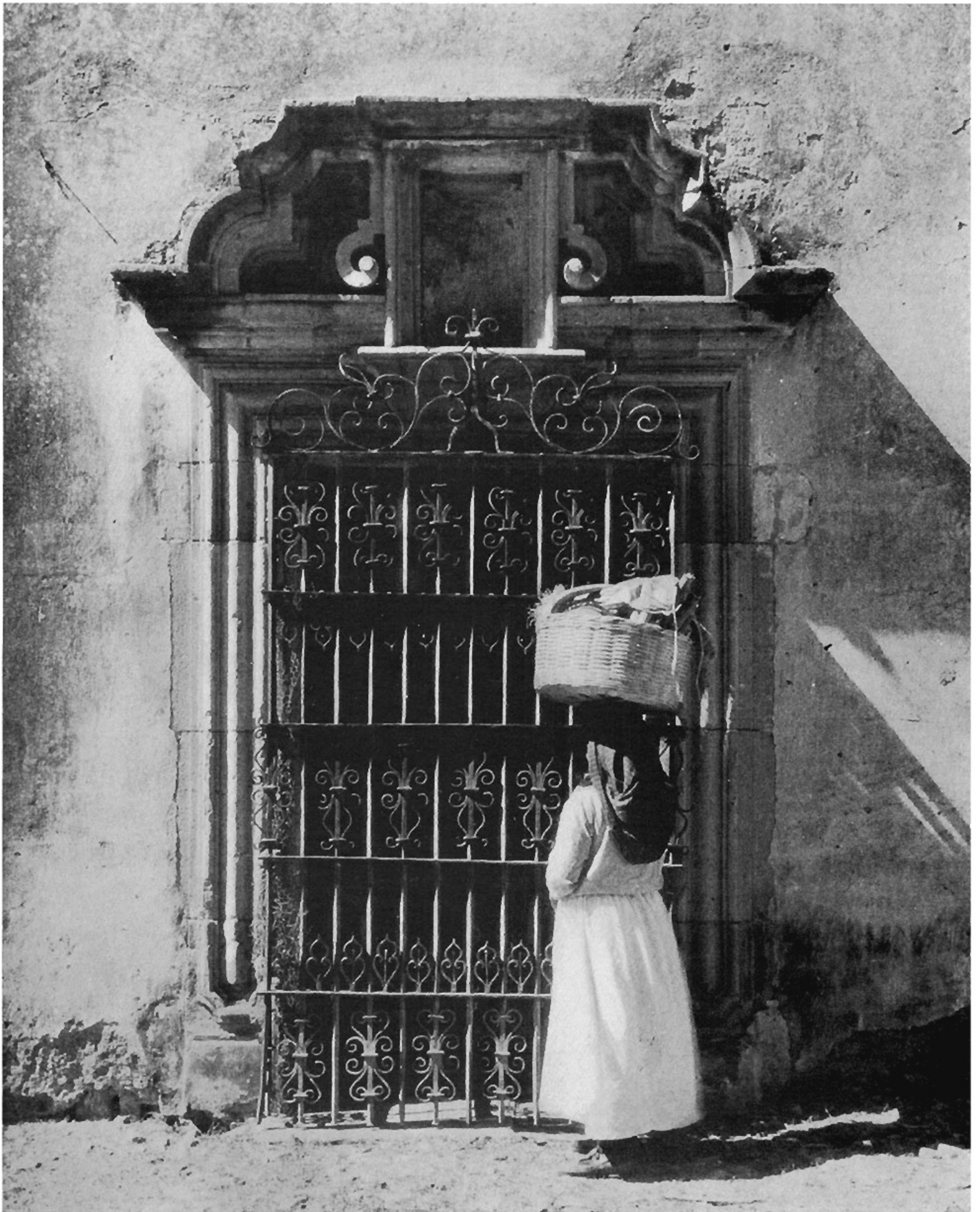
House of the Conde Rul at Valenciana, near Guanajuato. Window with a wrought iron grille. A carved stone figure is missing from the niche above
