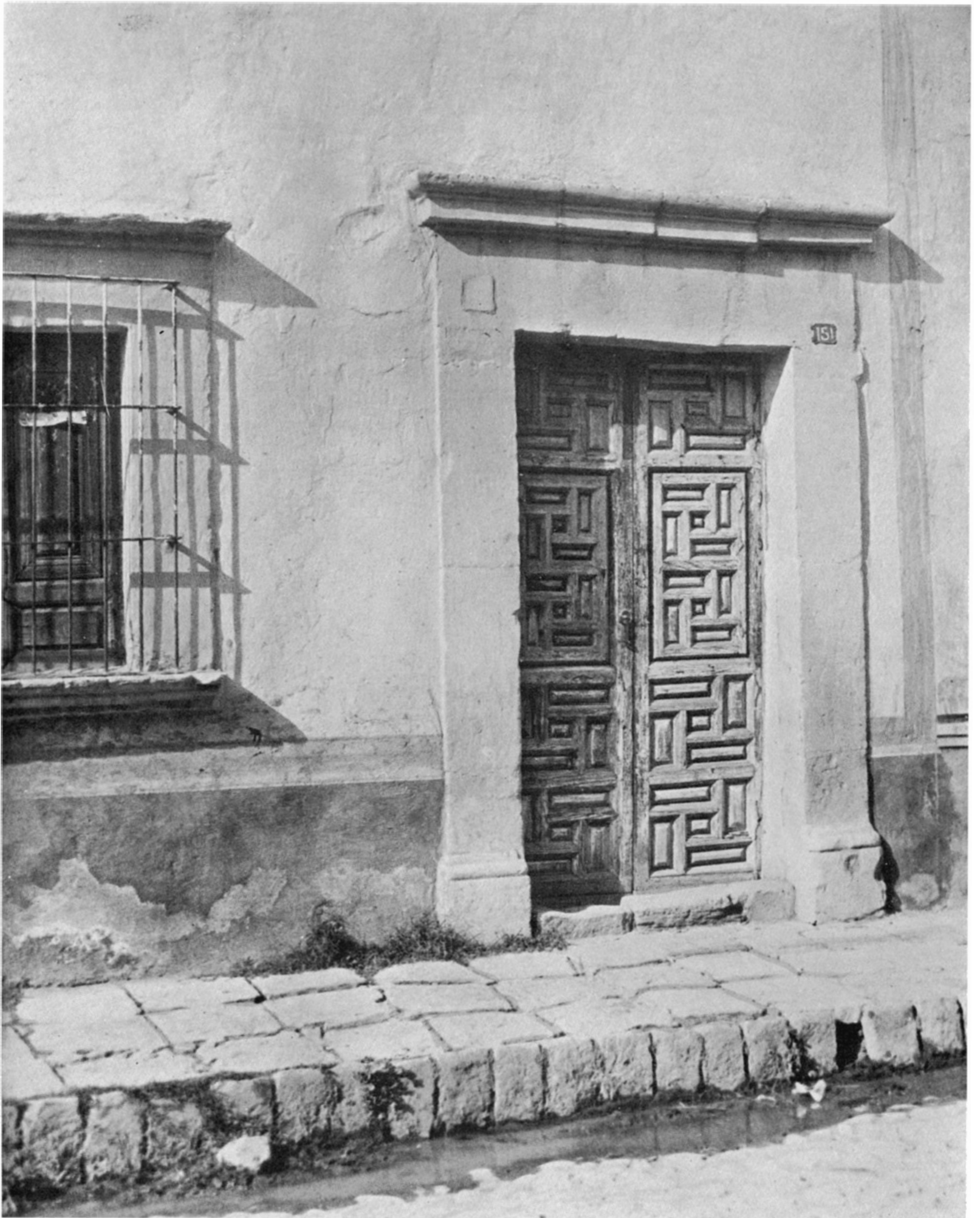
House of the Blue Door. Walls are of masonry, plastered and painted. Stone trims are also painted
