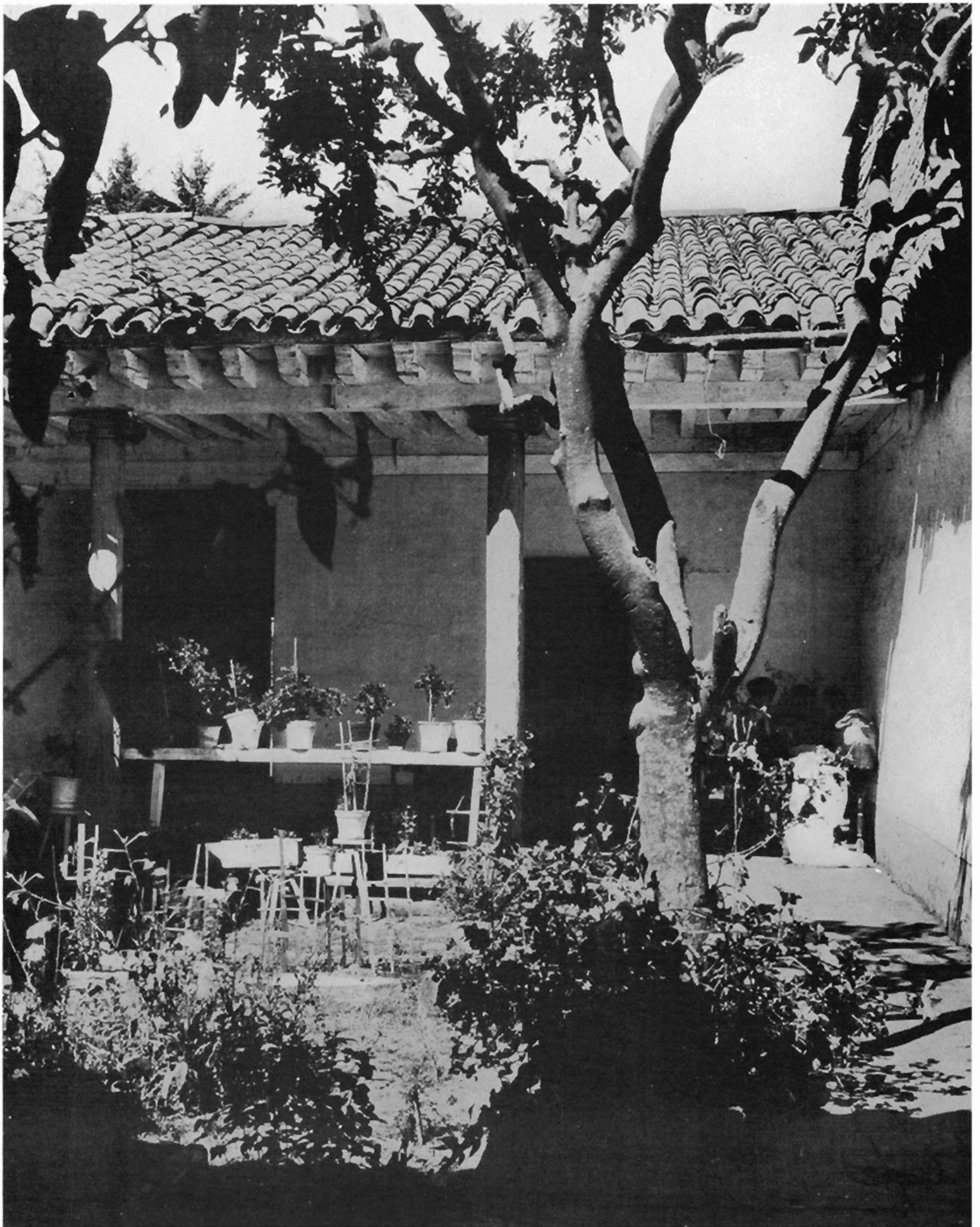
A small patio with corridor across the front side only. The columns and caps are of wood. Wood shakes across the projecting beam ends support a fill of brick and mortar below the tile. The frieze and dado are flat paint
