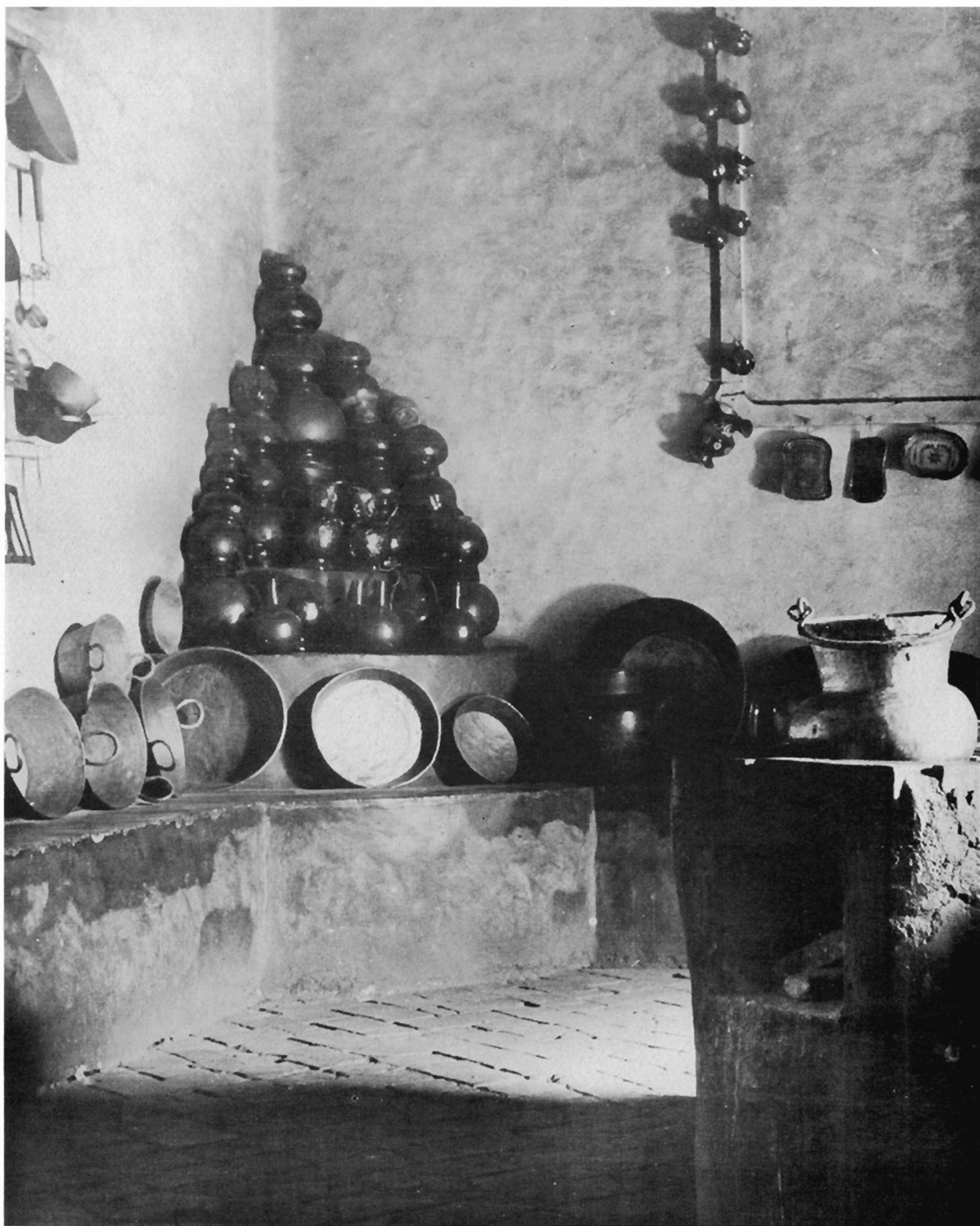
The kitchen of Doña Louisa Maria. Masonry shelves for the pots are topped with paving brick, the front is plastered, painted with red ochre, and polished to a lacquer finish as are the sides of the brasero, the corner of which shows in the foreground. Pots form the initials L. M. on the far wall
