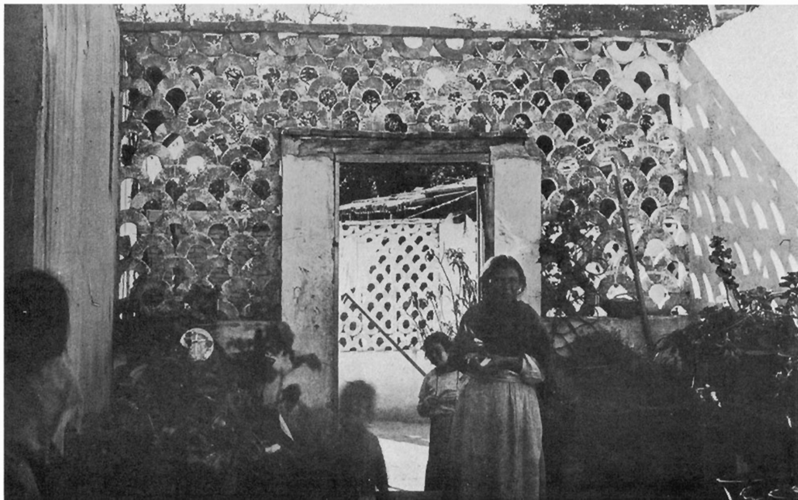
Above. Detail of a cornice of painted stone with a frieze of blue and white glazed tile. Below. A citarillo of shaped bricks, used to screen a rear yard from a small front patio
