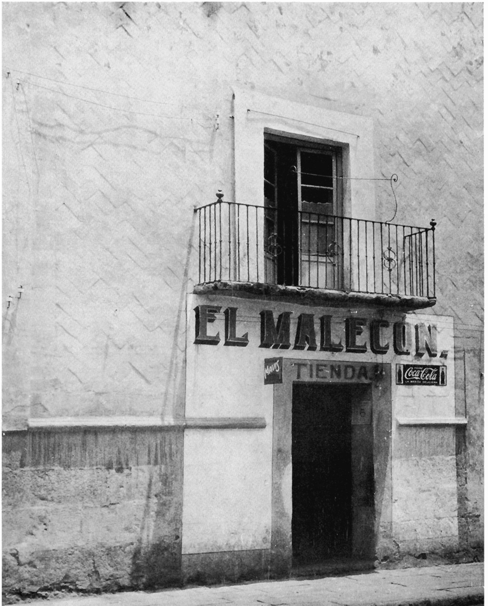
A masonry wall faced with brick laid in a herringbone pattern, and painted a cream pink with water paint. The stone base is oil painted a light plum brown
