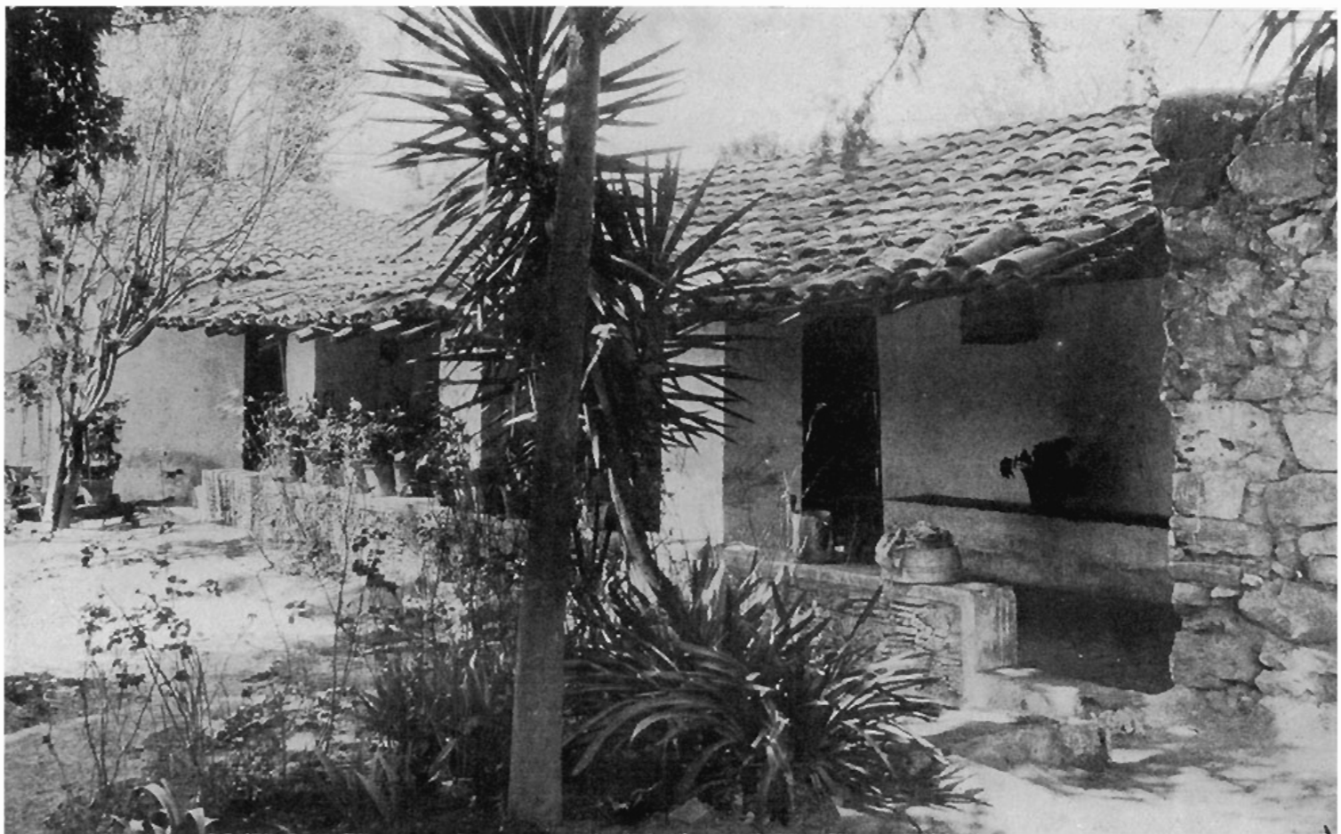
Above. A typical flat roofed adobe house. The plaster is carried down to cover the rock face below. Base, window trim, and outside border band are red, inside border band a lighter red, and field a cream pink. Below. House at an orchard. A door is the only opening in the outside wall along the highway
