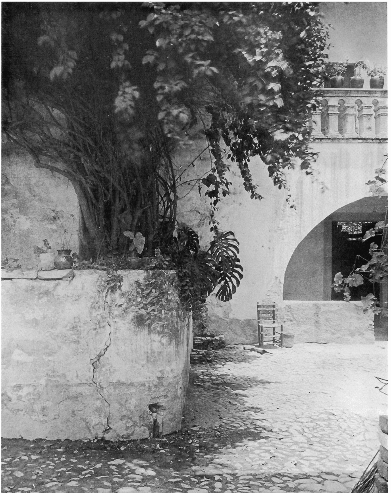
Corner of the patio of a large two-story house. A masonry wall raises the planting above the pavement and protects it from insects. The moulds of the second floor balustrade are roughed out in brick, then run in plaster
