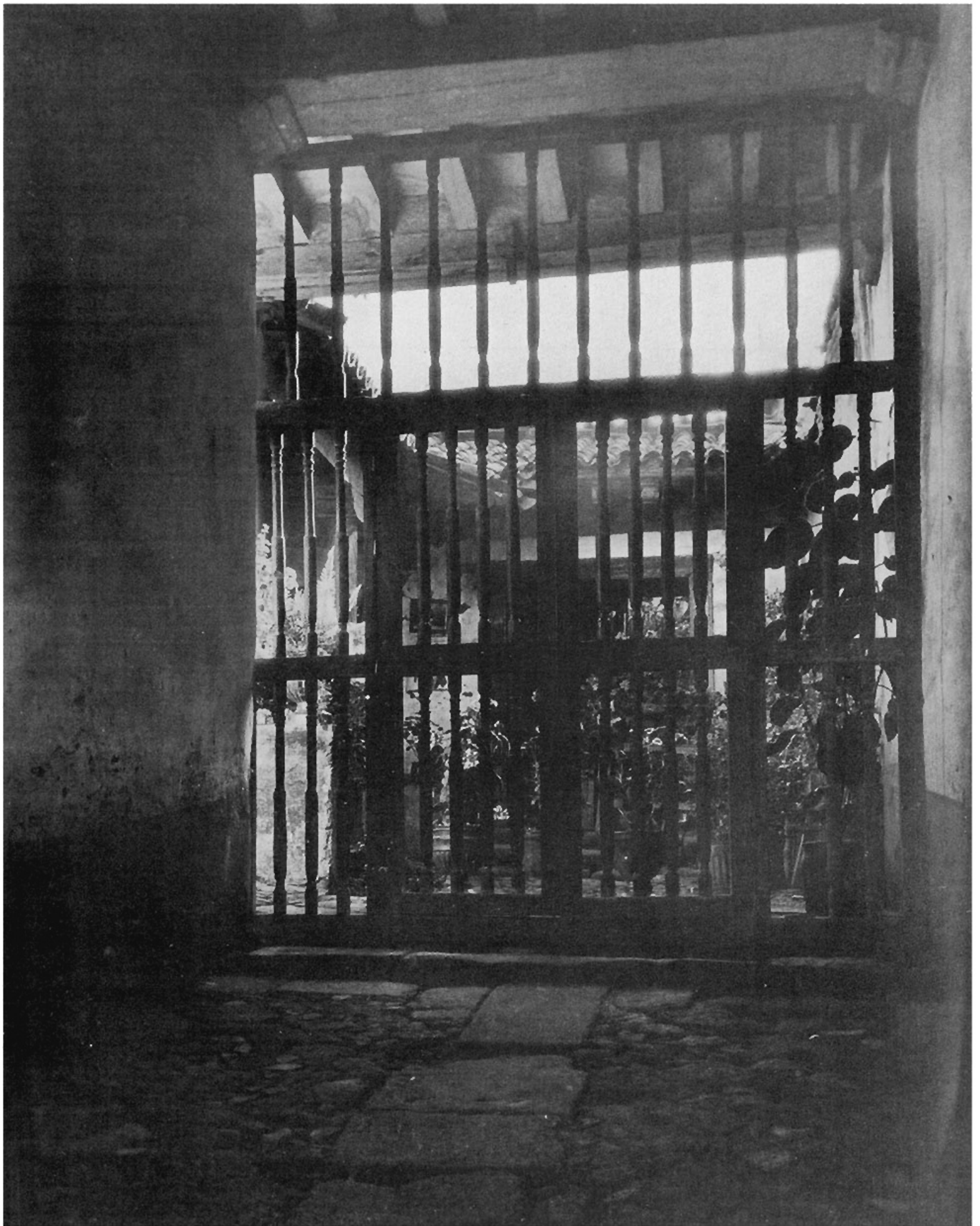
Porton of a small house. A porton screens the patio from the entry way, affording some protection while the great doors of the zaguan stand open during the day. It permits a view and allows a free circulation of air
