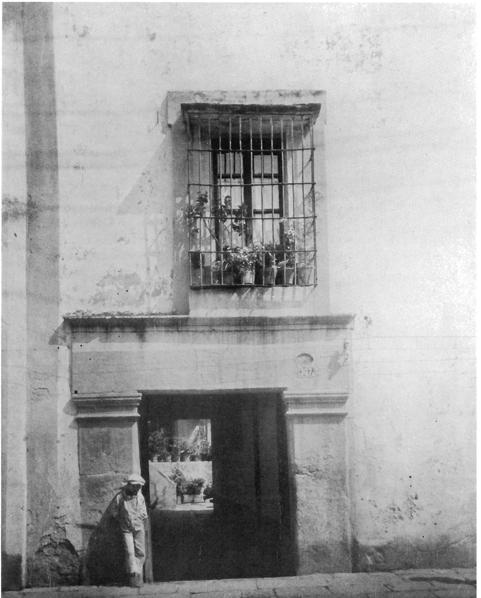
Entrance to a dwelling. The entry is three steps below the sidewalk level. The trim of the door and window is of cut stone in a plastered masonry wall. The off center window is not unusual
