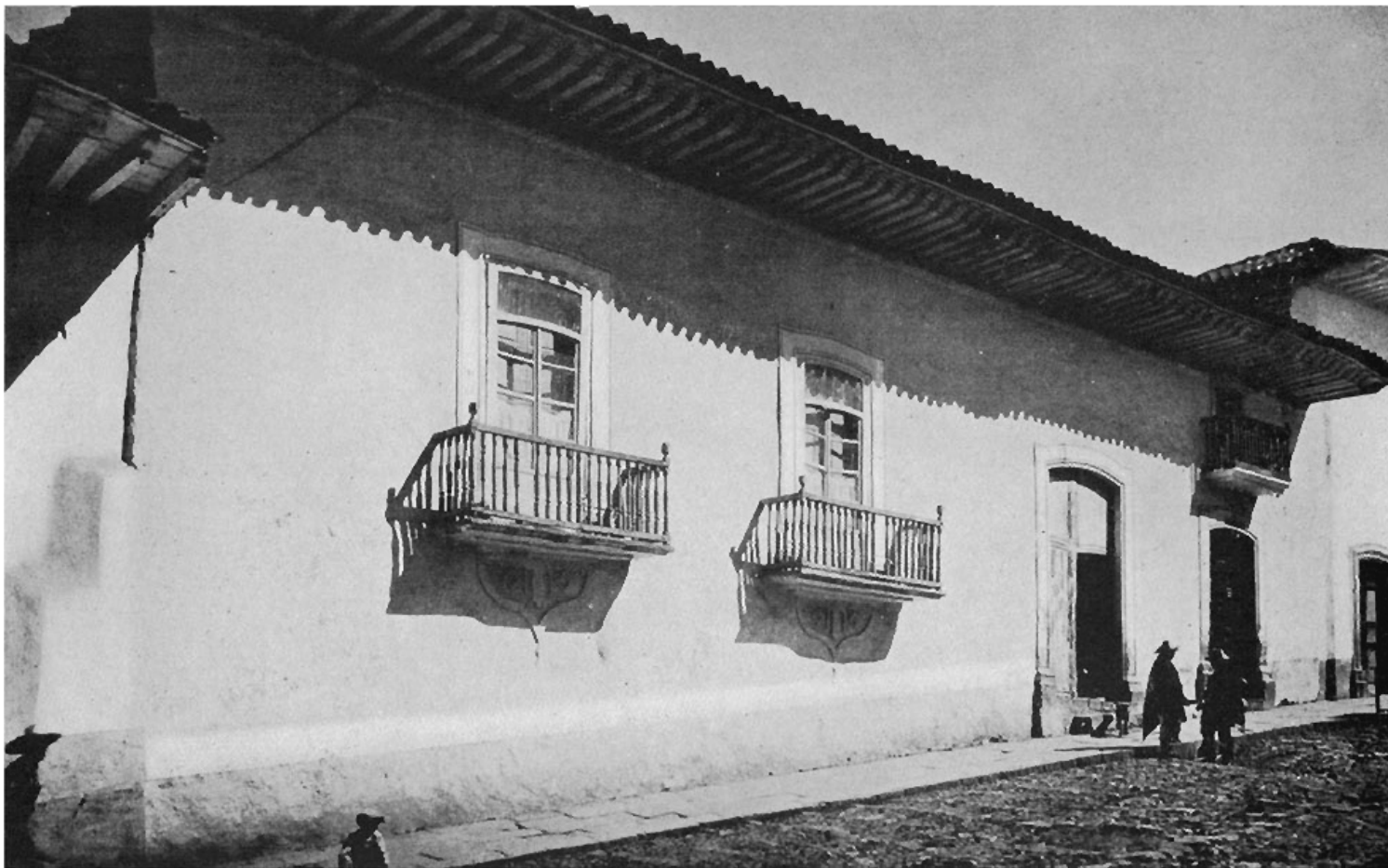
Above. Casa del Virrey. The very low first floor occupied by shops and quarters for servants and animals is typical of many Patzcuaran houses. The original turned wood balcony rail has been replaced by one of iron. Below. Facade of a house, painted light blue with trim and beam ends cream white and base dark red
