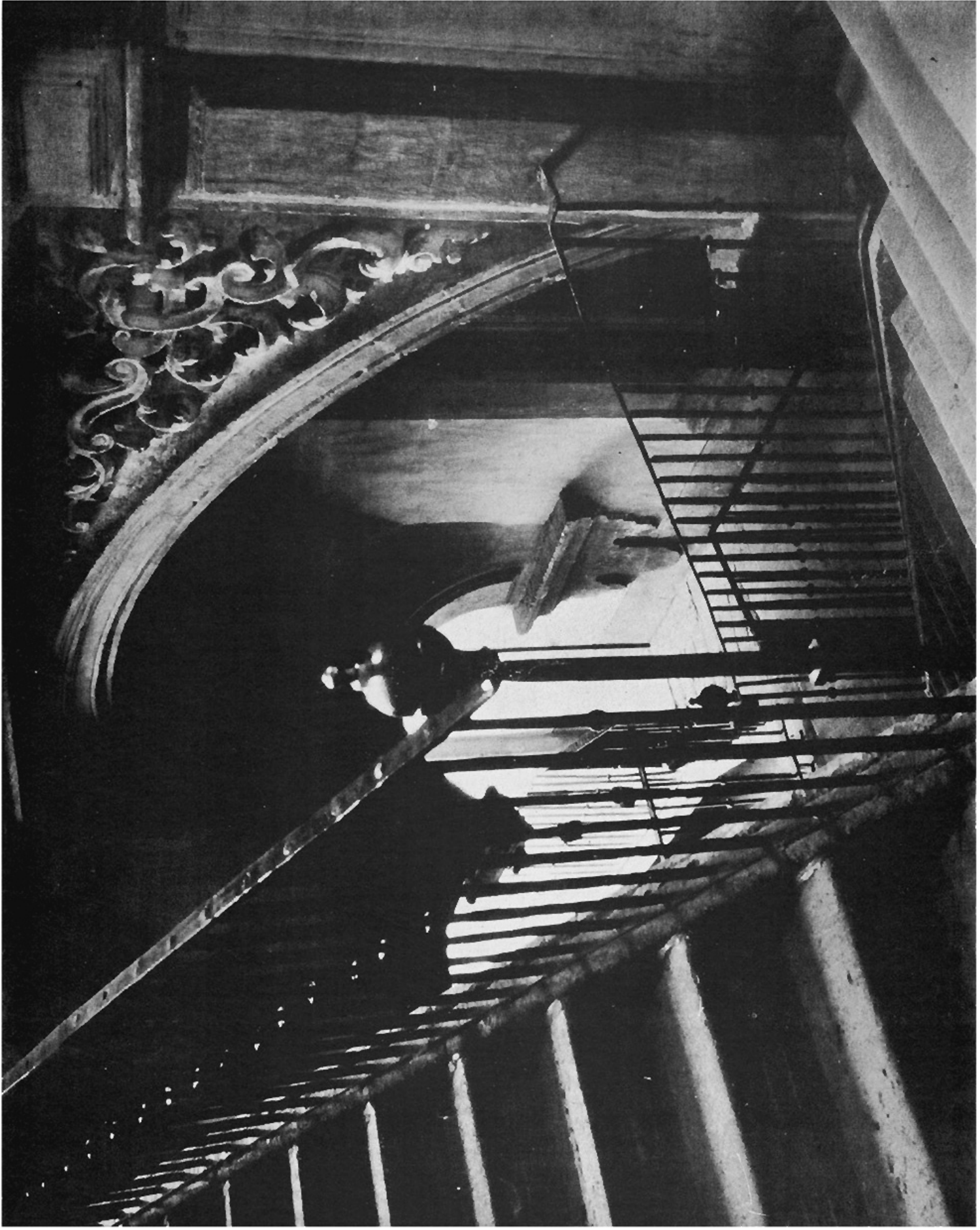
House of the Marquesa de Uluapa. A view from the landing of the stair which connects the entre suelo with the main floor. The stone treads and trimmer are carried on heavy open wood stringers set rather close together. Risers have glazed tile inserts. The finials are brass
