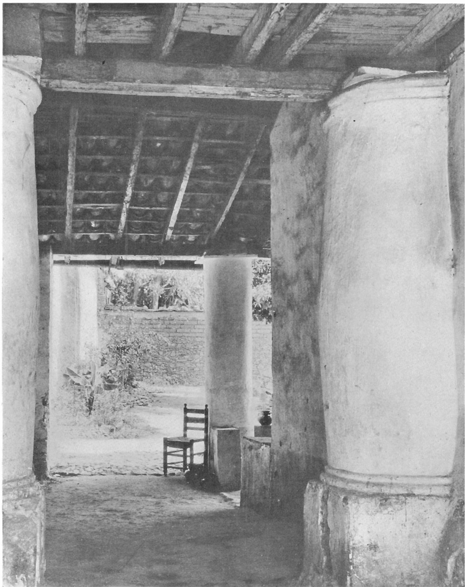
View through the entrance of a small house. An open corridor with exposed tile roof faces the garden. The plain round columns are of mixed masonry plastered and painted white, and capped with thin paving brick
