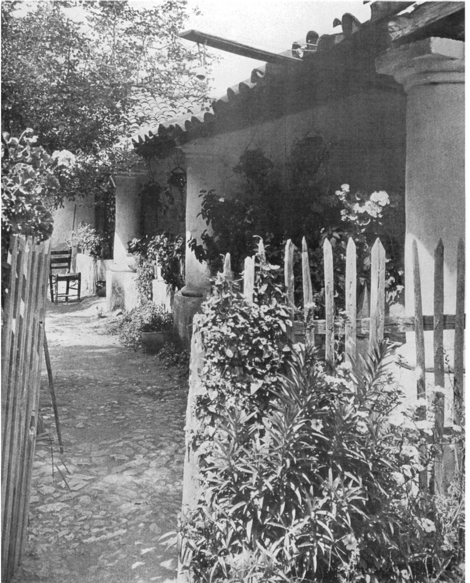
The Carpenter's House. View of the open corridor. The pathway is of earth and broken stone
