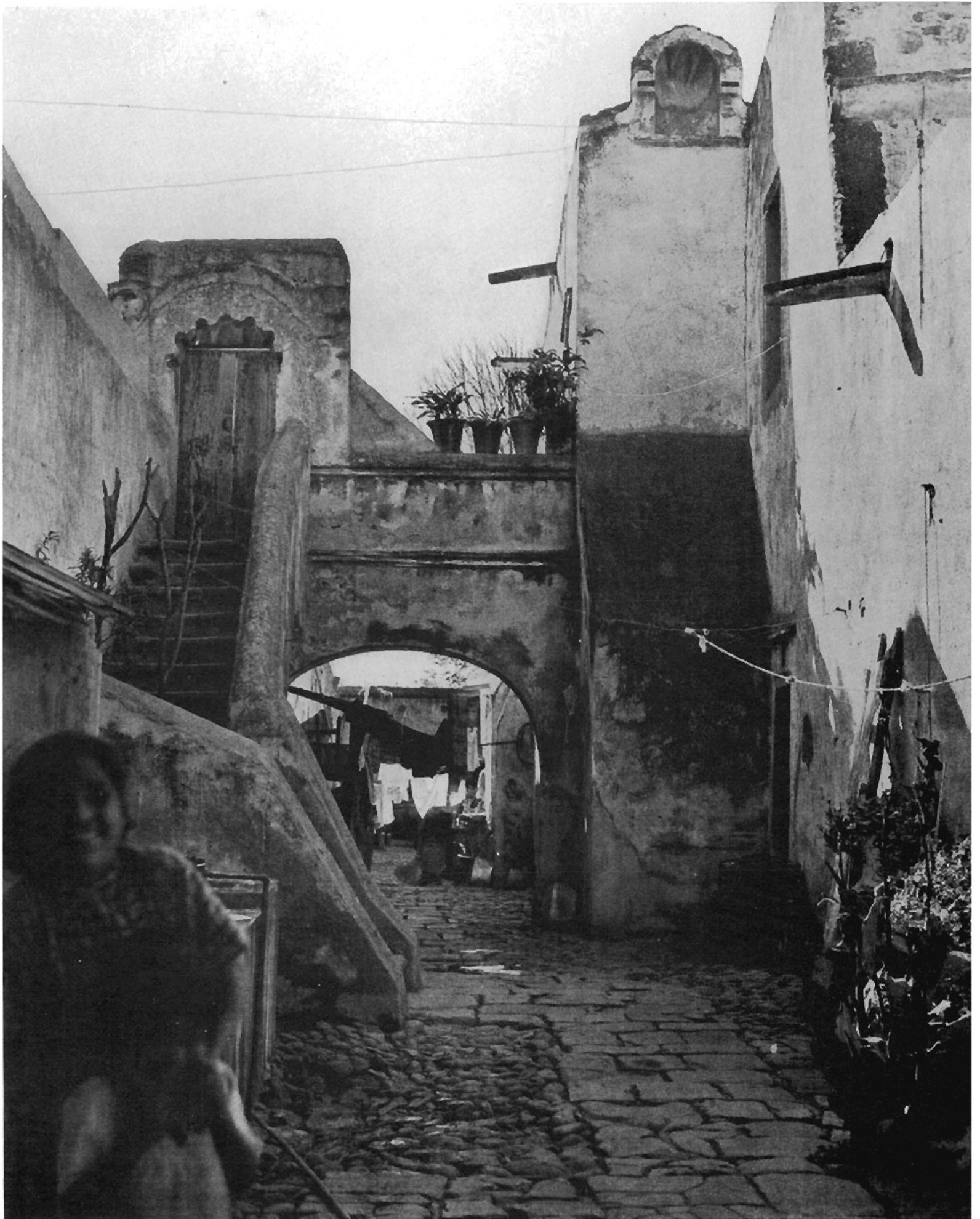
A Vecindad. Walls of masonry plastered and painted. From the top of the stair the bridge leads to rooms on the second floor rear
