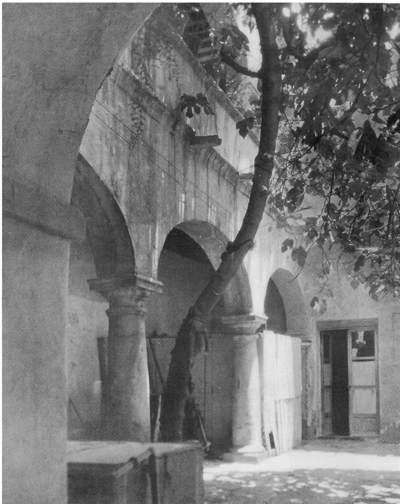
Arcaded side of patio in an early Eighteenth Century House. Columns of stone, walls of mixed masonry, plastered over. A single fig tree with its shadows softens the light and contrasts with the salmon pink painted walls
