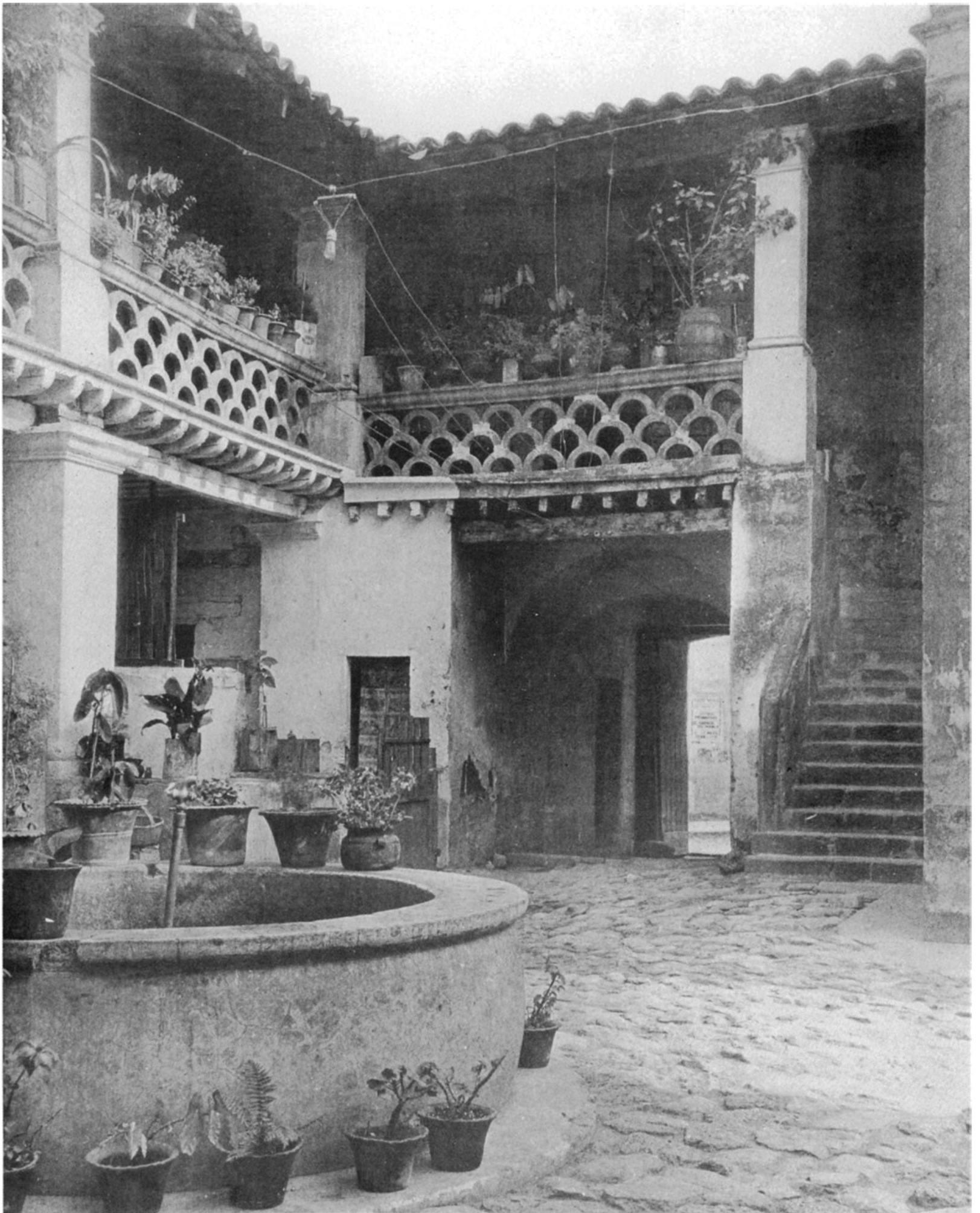
Patio of a casa de altos. A view toward the entrance. The open balustrade is of shaped bricks
