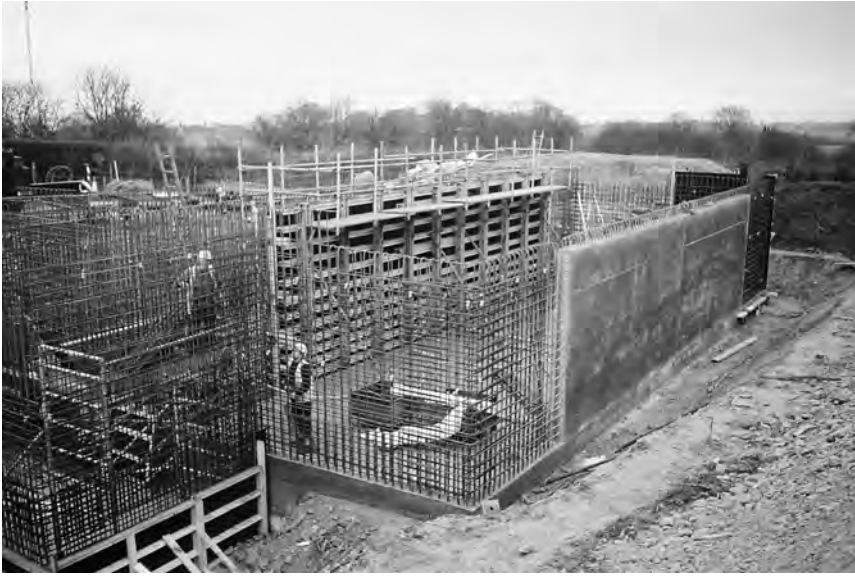
Figure 1.1 A tank under construction (Photo: J.P. Forth/A.P. Lowe).
