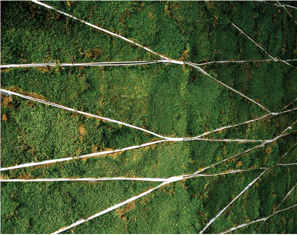
LEFT: Moss-filled panel. Photo: Michael Vahrenwald BELOW: Assembly. Photo: MOS
