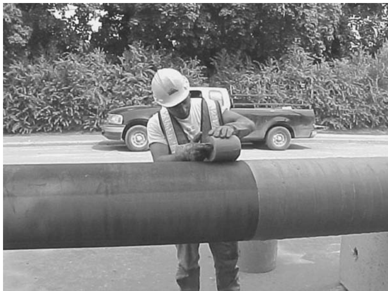
FIGURE 10.6 Wrapping a water main pipe with adhesive tape to provide a barrier against soil corrosion. (Courtesy of Drinking Water Services, City of Ottawa)
