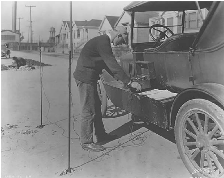
FIGURE 7.4 An electrolysis surveyor using a McCollum earth current meter from the early 1920s. (Courtesy of East Bay Municipal Utility District).
