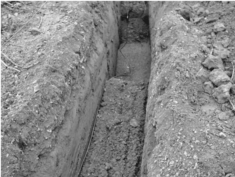
FIGURE 13.18 Conventional groundbed using petroleum coke backfill and 5 cm cast iron anodes. (Courtesy of Dean Rookes, West Coast Corrosion Prevention Ltd.)
