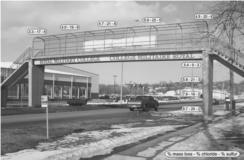
FIGURE 9.19 Results of a study investigating the transport and effects of deicing salt-laden aerosols.
