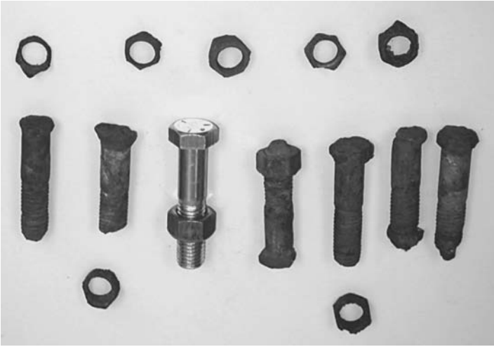
FIGURE 7.31 Severe corrosion of fire hydrant bolts and nuts due to stress cells. (Courtesy of Drinking Water Services, City of Ottawa)
