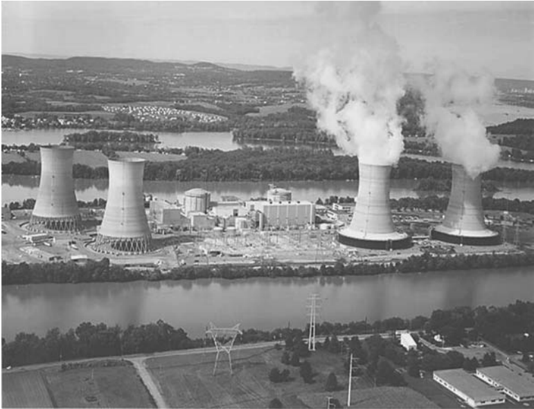
FIGURE 8.12 Natural draft cooling towers with their characteristic height and distinctive hourglass shape. (Courtesy of Russ Green, TMI)
