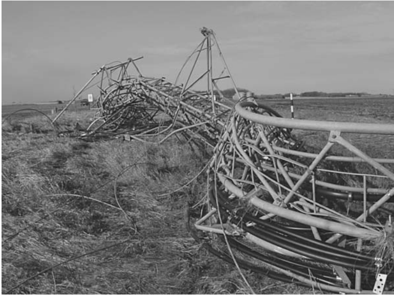
FIGURE 7.16 Mangled communication tower fallen due to loss of the anchor shown in Fig. 7.15. (Courtesy of Anchor Guard)
