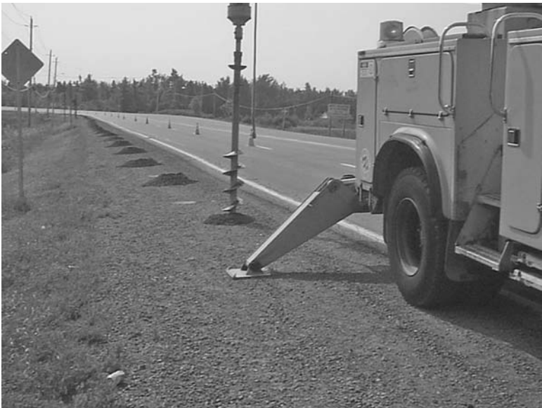
FIGURE 13.17 Holes being drilled for sacrificial anode installation (a); thermit welding of anode connection on watermain (b); anode cluster ready to be buried and connected to fire hydrant tap. (Courtesy of Drinking Water Services, City of Ottawa)
