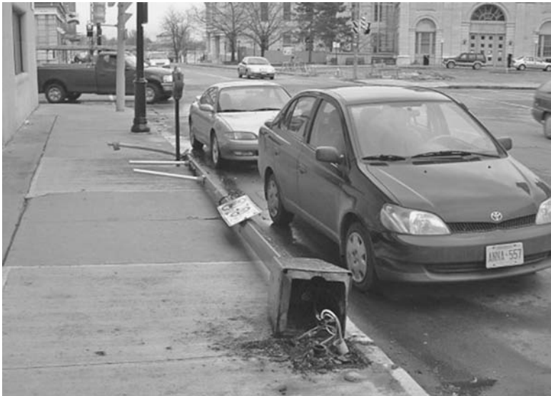
FIGURE 11.17 City lamppost fallen due to corrosion of its base. (Courtesy of Bruce Hector, Rust Check Kingston)
