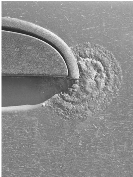
FIGURE 14.5 Beach marks indicative of the cyclic progress of a car door coating failure.
